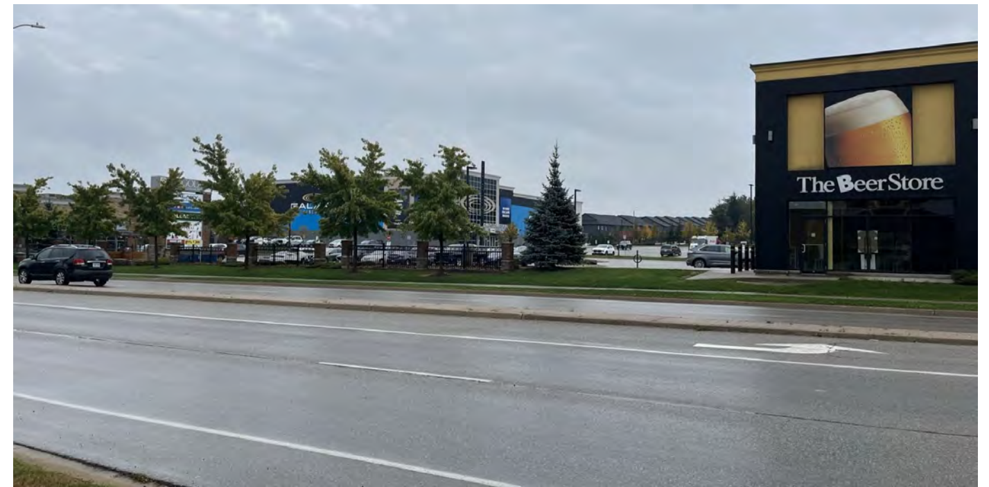
Photo 1 Looking South-East along Clair Rd E to Subject Lands
