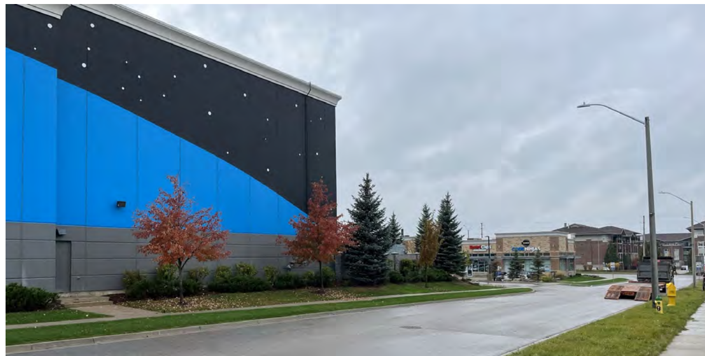
Photo 5 Looking West along Hawkins Dr to Subject Lands
