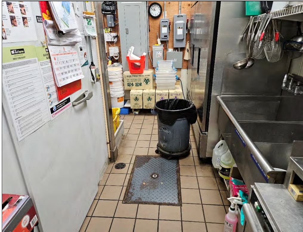
Photo 33: Kitchen area and grease trap in kitchen at Thai Express
