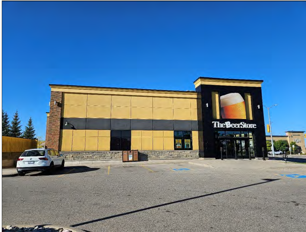
Photo 17: The Beer Store (Building C), front of building.
