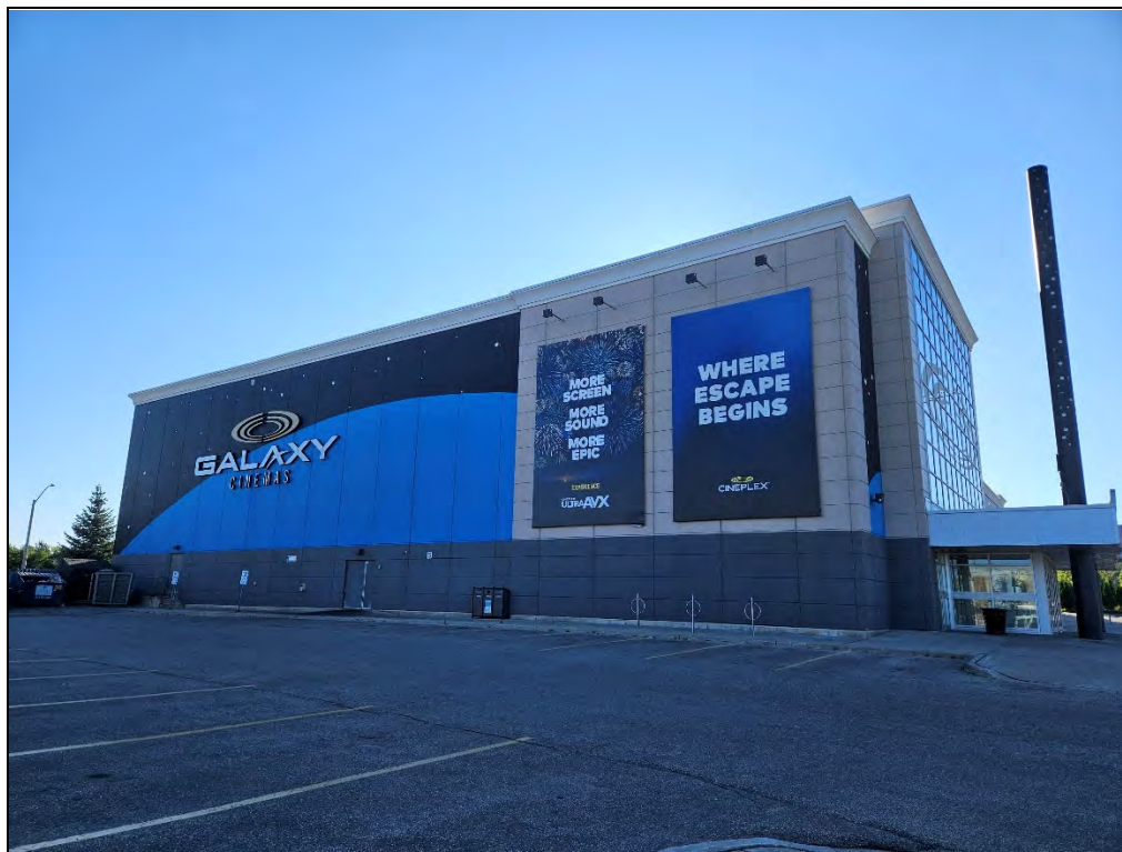
Photo 2: 85 Clair Road East, Galaxy Cinemas (Building A).
