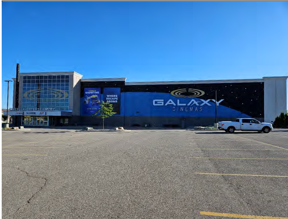
Photo 1: 85 Clair Road East, Galaxy Cinemas (Building A). Front of building.
