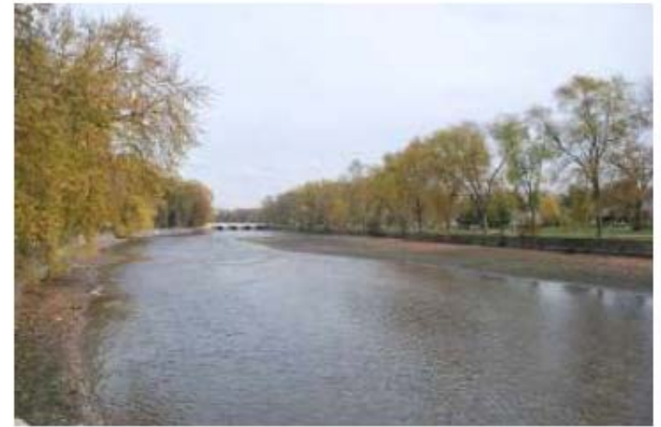
View of Gordon Street Bridge with similar views of mature trees and the stone walls.
