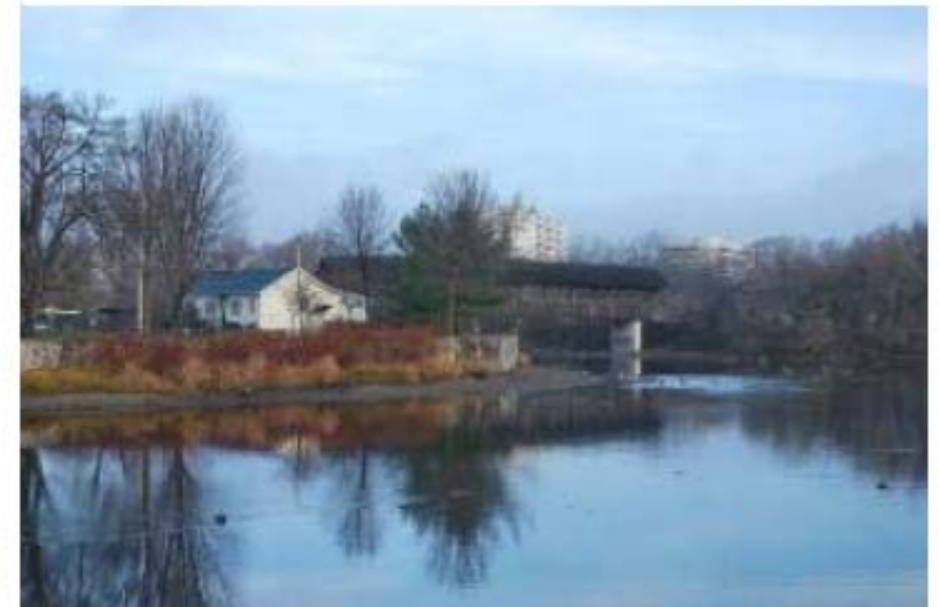
View of the Covered Bridge and naturalizing vegetation on the east bank.
