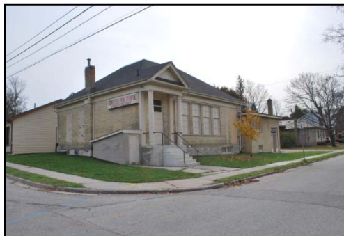
Blocking of window openings should be avoided
