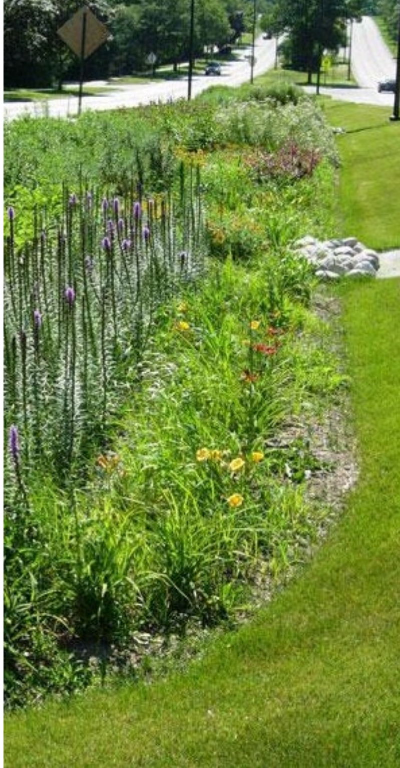
Figure 6: This bioswale in the median of Grange Avenue in Greendale, Wisconsin, adds visual interest while also providing flood storage, filtering run-off, and supporting local pollinator populations. Source: Aaron Volkening
