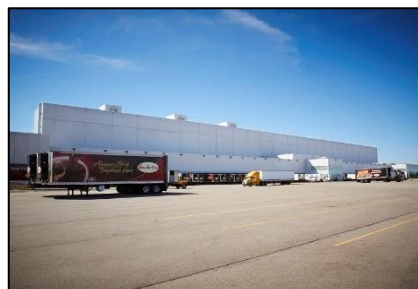
TDL Group Distribution Centre 950 Southgate Drive
