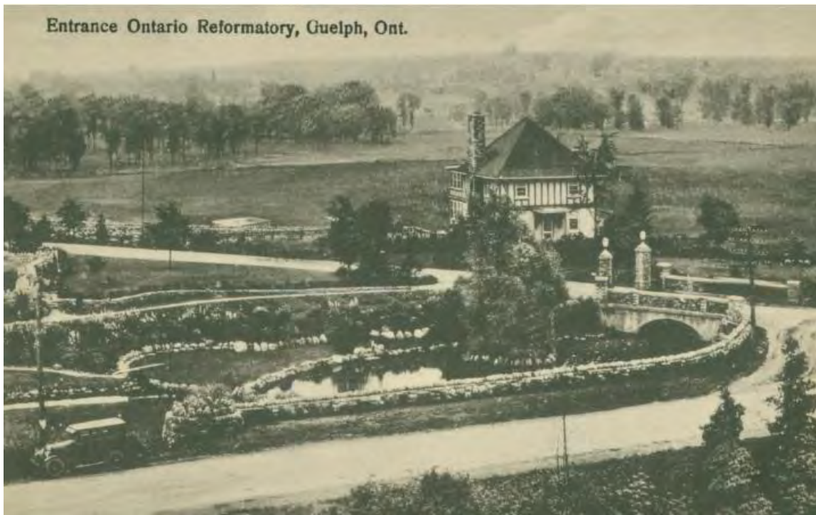
Photograph 4: 1920's Picture of Dry Stone Wing Wall with Circular End Treatment. The height of the wall is noticeably taller. The existing wall has been partially buried due to road grading. Photo from the Guelph Civic Museum.
