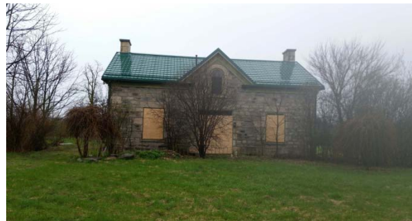
Figure 17: Listed residential building at 331 Clair Rd. E.
