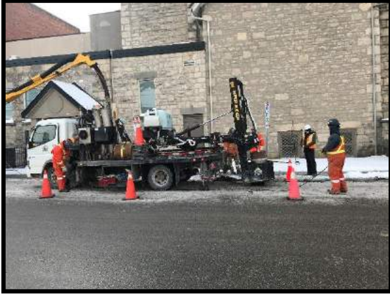
Image 17: Daylighting (January 9, 2020; Facing South)
