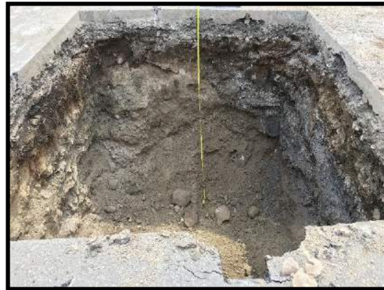
Image 8: Mechanical Excavation (July 26, 2019; Facing Southeast)
