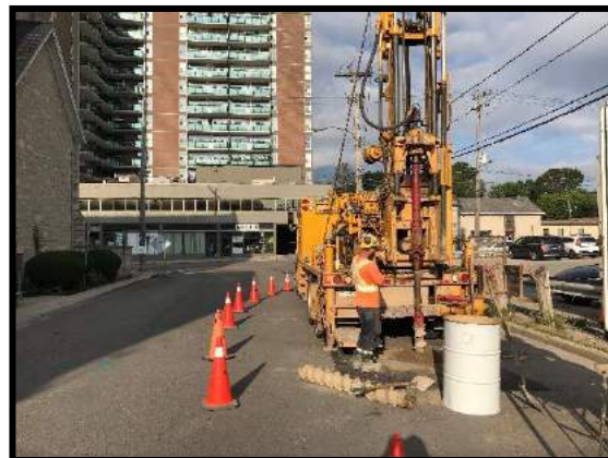
Image 16: Mechanical Drilling (August 20, 2019; Facing West)
