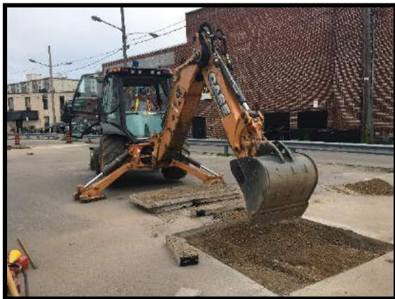
Image 3: Mechanical Excavation (July 22, 2019; Facing Northeast)
