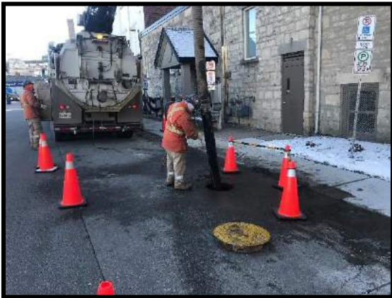
Image 19: Daylighting (January 17, 2020; Facing Southeast)
