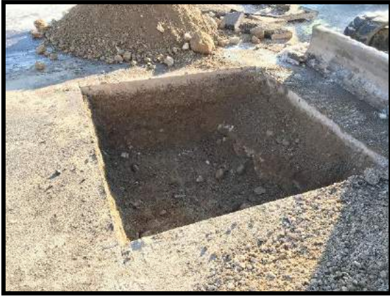
Image 5: Mechanical Excavation (Nov 12, 2019; Facing East)
