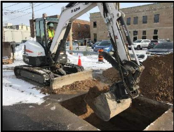
Image 7: Mechanical Excavation (November 13, 2019; Facing Northeast)
