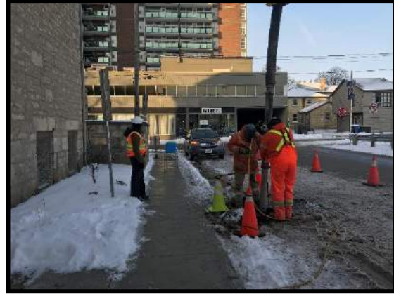
Image 18: Daylighting (January 9, 2020; Facing West)
