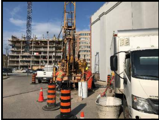
Image 1: Site Conditions (August 16, 2019; Facing Southwest)
