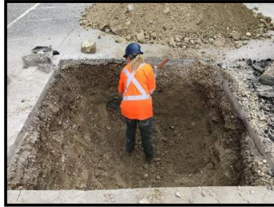
Image 6: Mechanical Excavation (July 23, 2019; Facing East)
