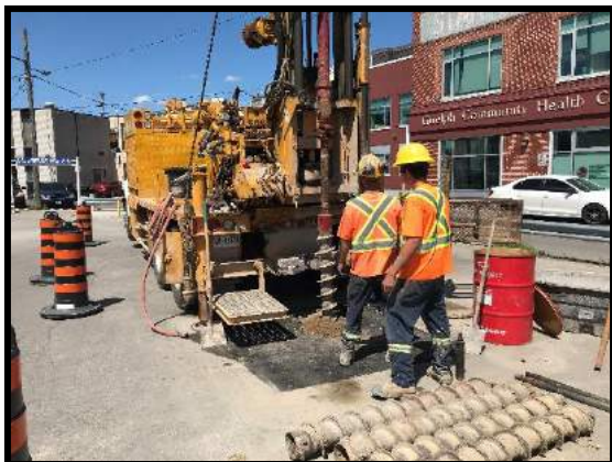
Image 15: Mechanical Drilling (August 14, 2019; Facing Northeast)
