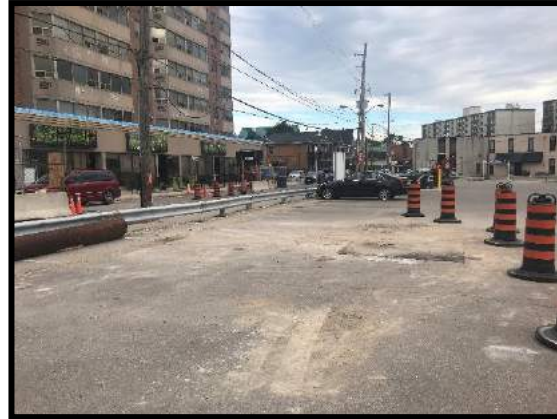
Image 2: Site Conditions (August 22, 2019; Facing North)
