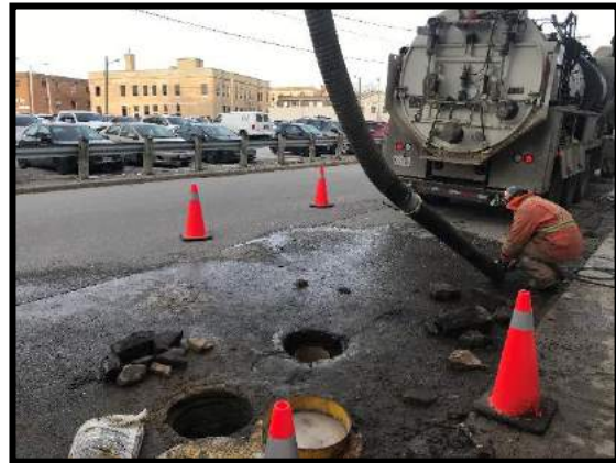
Image 20: Daylighting (January 17, 2020; Facing Northeast)
