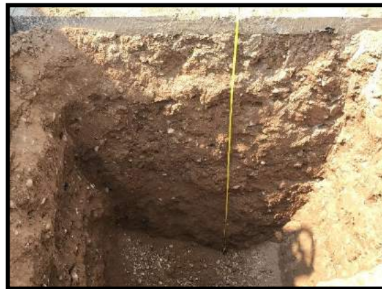
Image 4: Mechanical Excavation (July 25, 2019; Facing Northwest)
