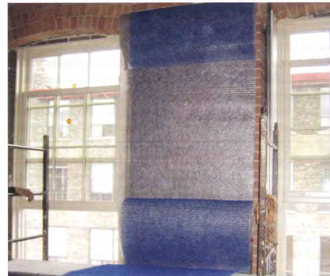
Figure 2: Application of the polymer mesh system (two layers).
