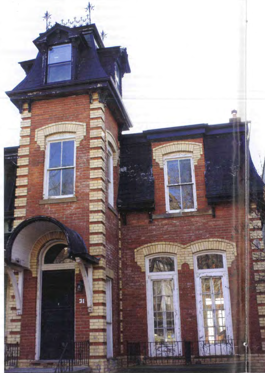
The Gemini House is a low-energy demonstration home on the University of Toronto's St. George Campus. All photos in this article provided by Ekaterina Tzekova.
