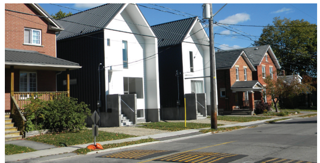
Example of infill development in Guelph.
