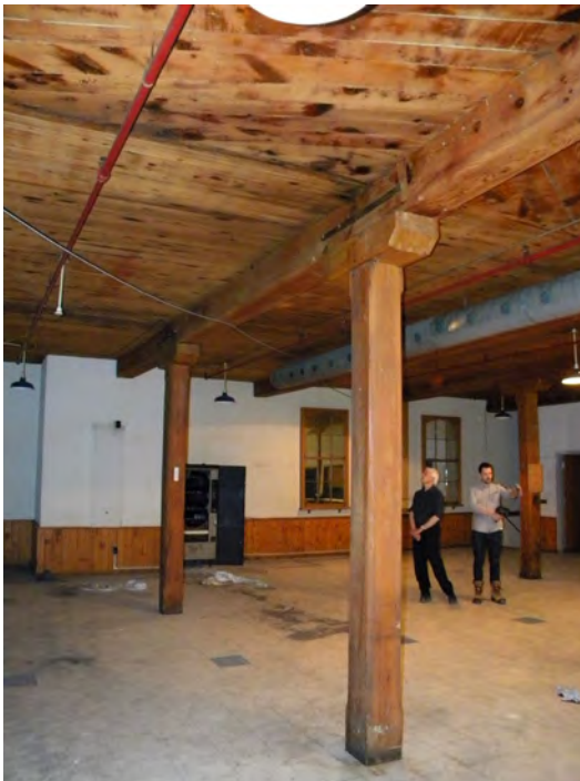
41. Building #2d, heavy timber structure. (Source: City of Guelph)
