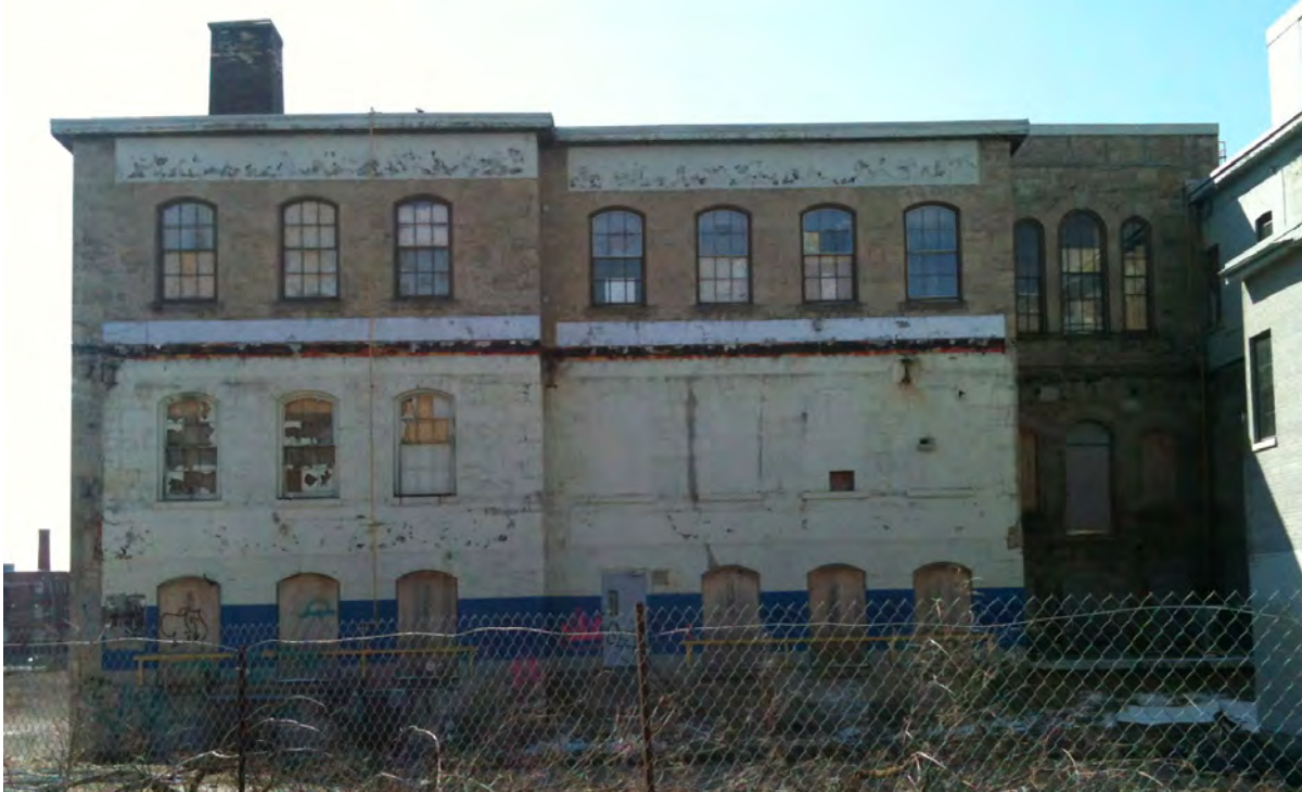
35. Building #2d, North Elevation, 2014 (Source: ERA)
