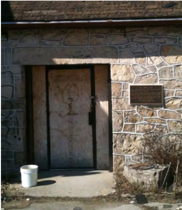
8. Building #1, door opening on East Elevation, 2014 (Source: ERA)
