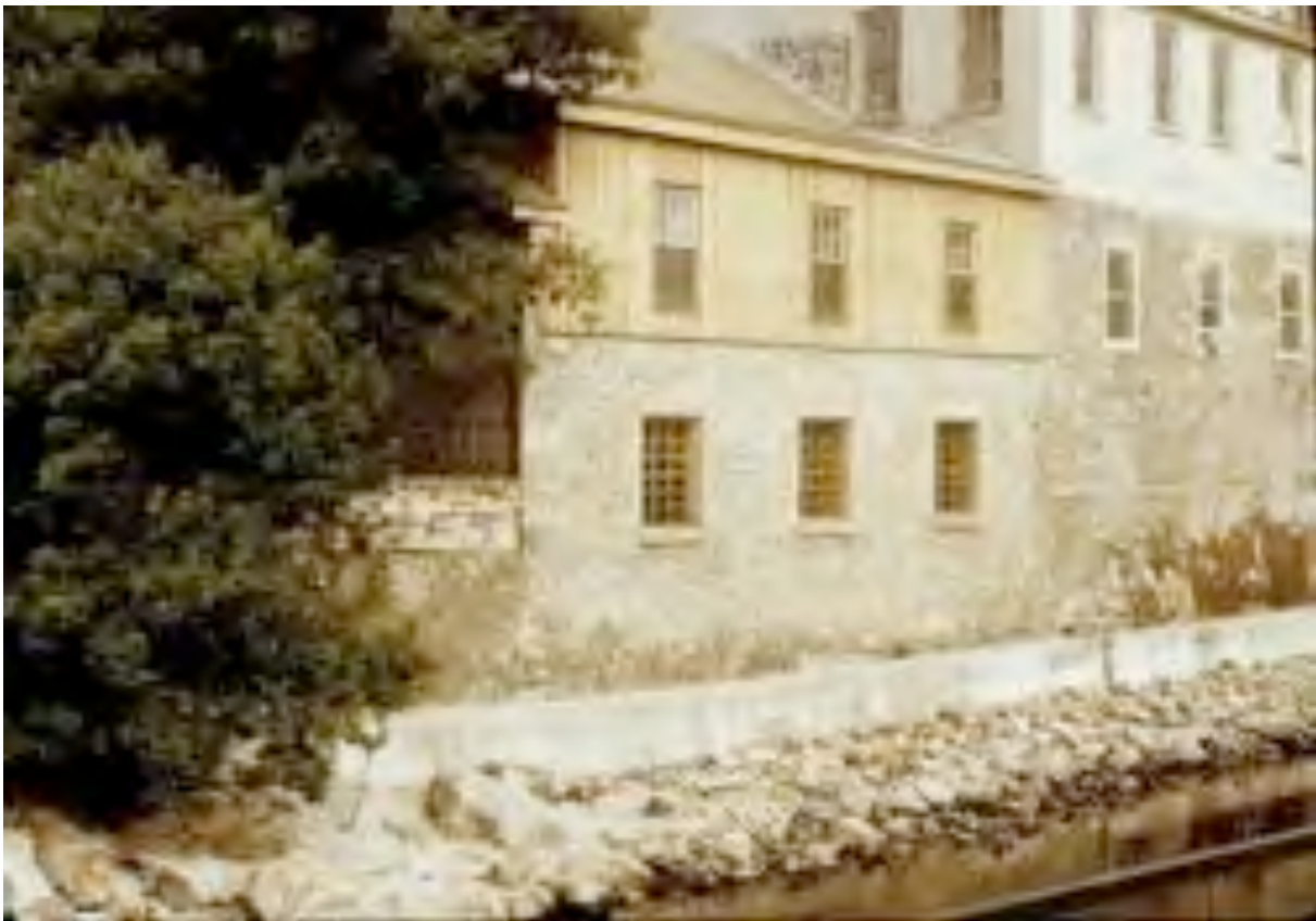
View of former distillery buildings before and after renovations by W C Wood Company, 1968 and 1980. Source: Couling Collection, Wellington County Museum and Archives
