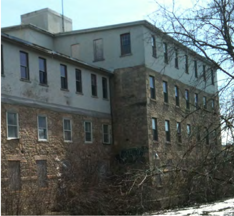
25. Building #2b, North and West Elevations, 2014 (Source: ERA)
