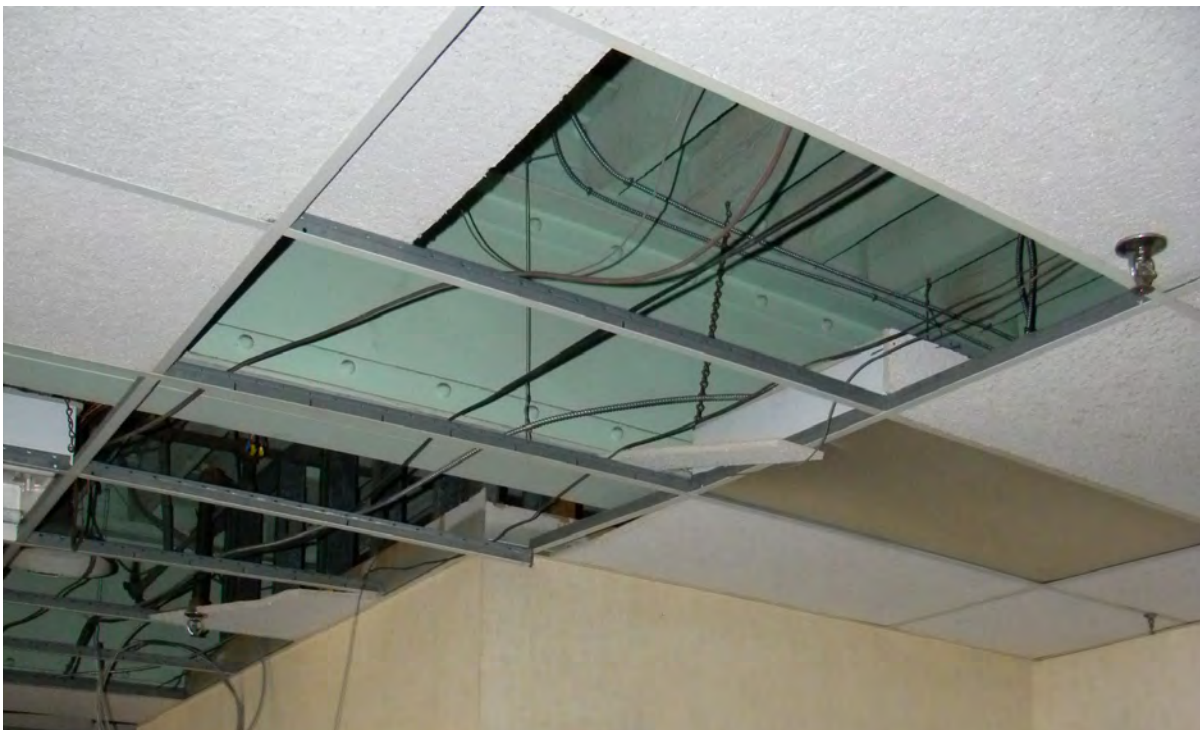
27. Building #2b, I-beam members (Source: City of Guelph)
