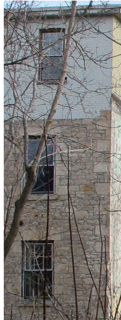
28. Building #2b, West Elevation showing varied window construction and quoined corners, 2014 (Source: ERA)
