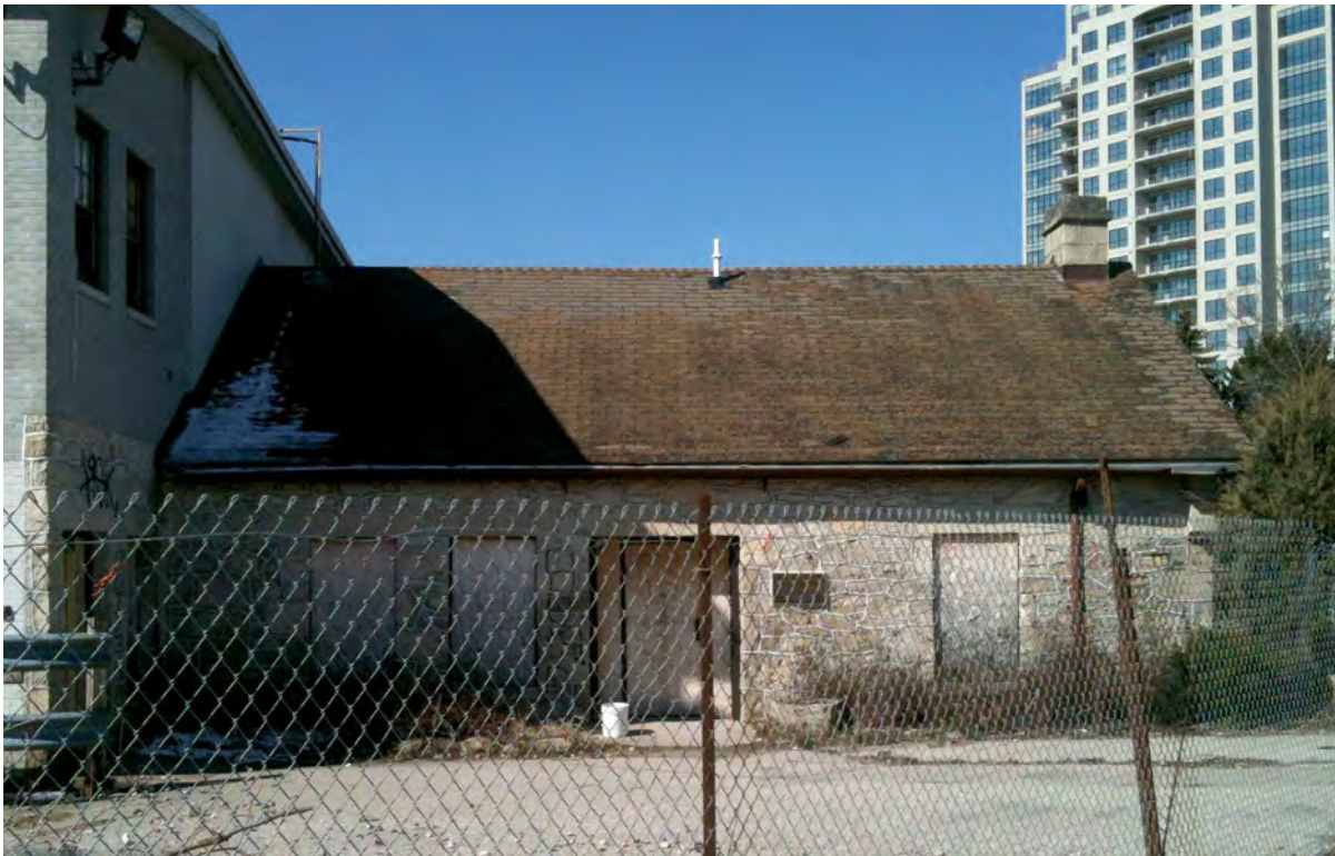
5. Building #1, East Elevation (Source: ERA)
