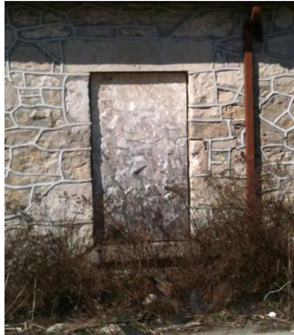
9. Building #1, representative window opening on East Elevation, 2014 (Source: ERA)
