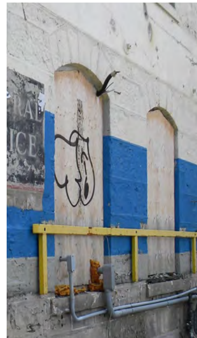
38. Building #2d, North Elevation, arched window (Source: City of Guelph)
