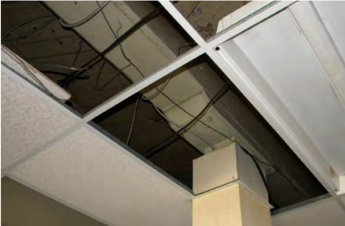
26. Building #2b, heavy timber structure (Source: City of Guelph)
