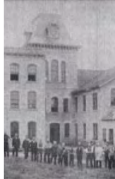
29. Building #2c, North Elevation with former roof. (Source: “Summary History”, p. 12)
