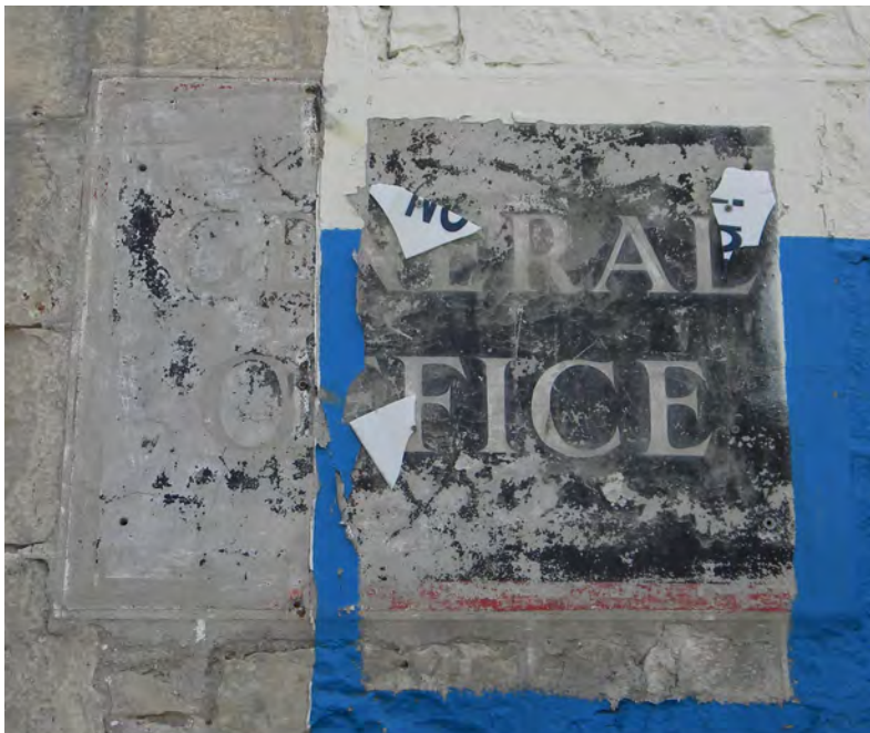
37. Building #2d, North Elevation, General Office' sign (Source: City of Guelph)
