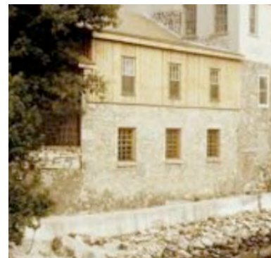
7. Building #1, West Elevation. Upper photo from 1968 taken prior to renovations by WC Wood Company shows original roof profile. Lower photo from 1980 shows roof dormer. (Source: "Summary History", p. 18)
