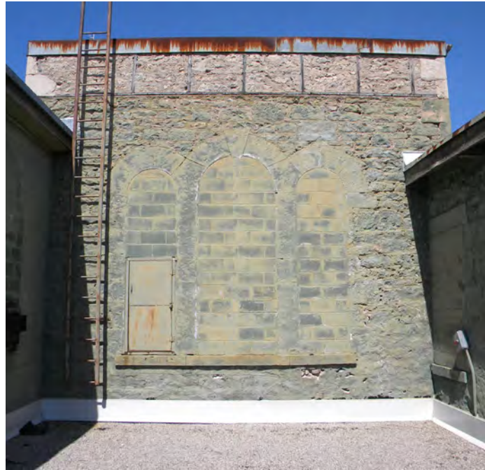
33. Building #2c, South Elevation, third floor (Source: City of Guelph)
