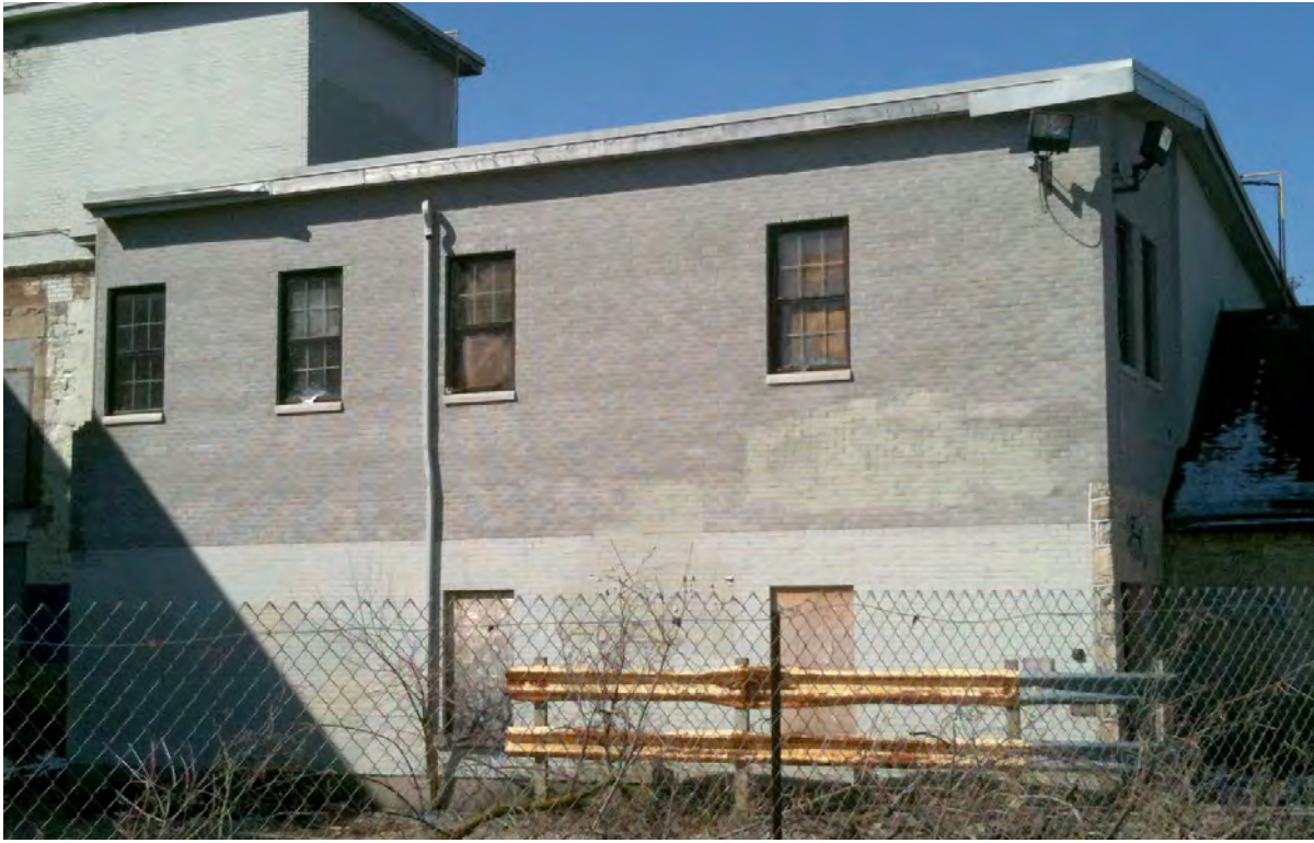
16. Building #2a, East Elevation, 2014 (Source: ERA)
