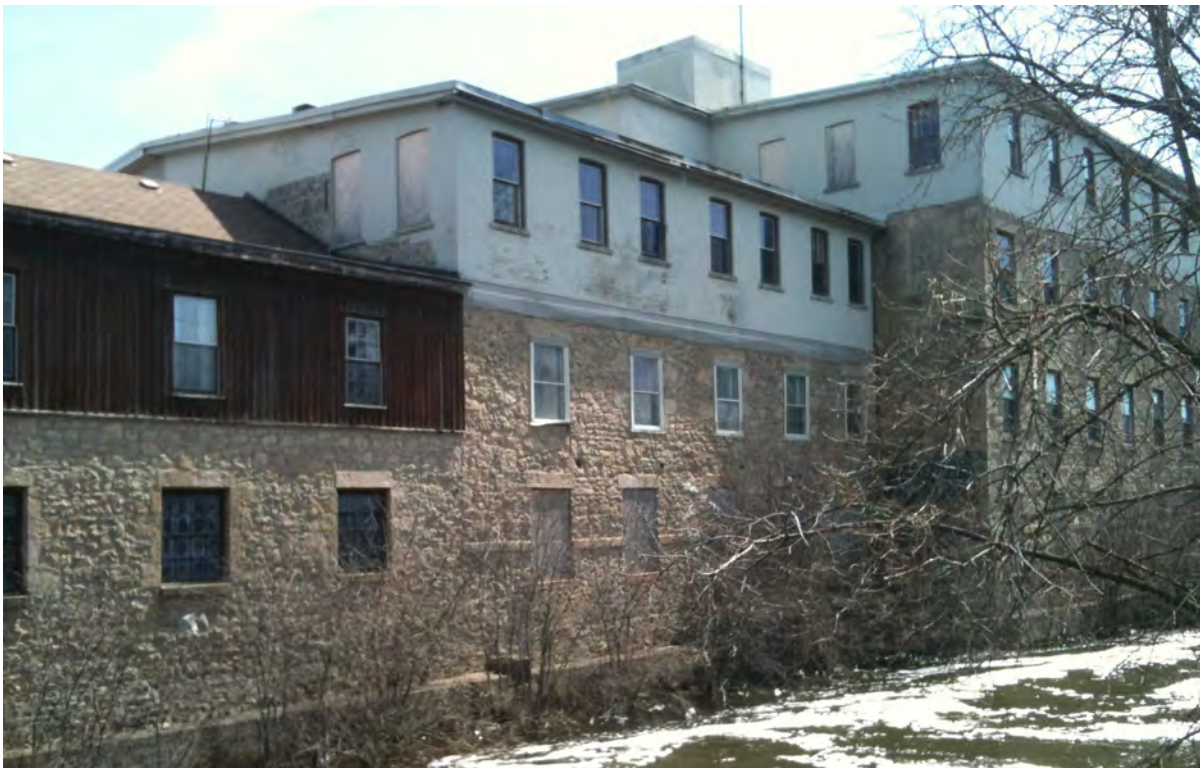
17. Building #2a, West Elevation, 2014 (Source: ERA)
