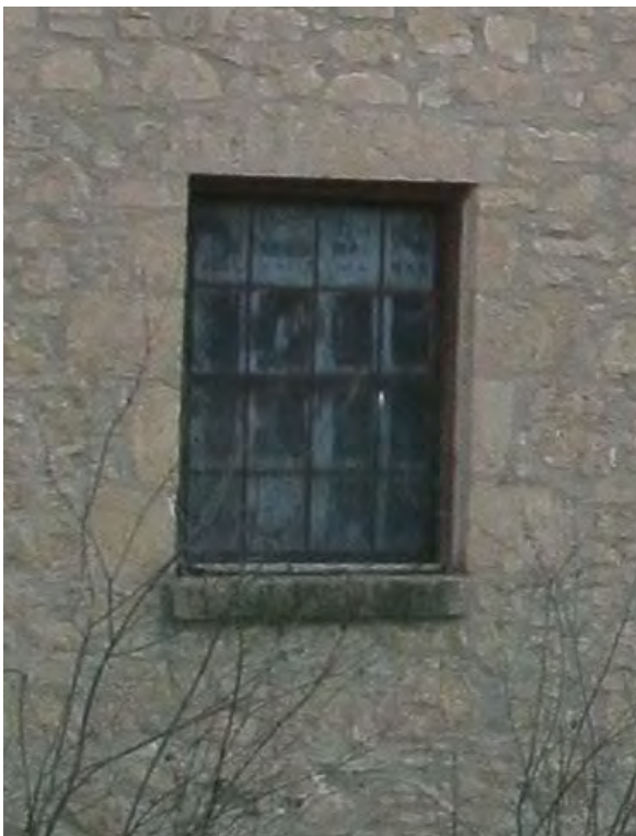
10. Building #1, representative window at lower floor of West Elevation, 2014 (Source: ERA)
