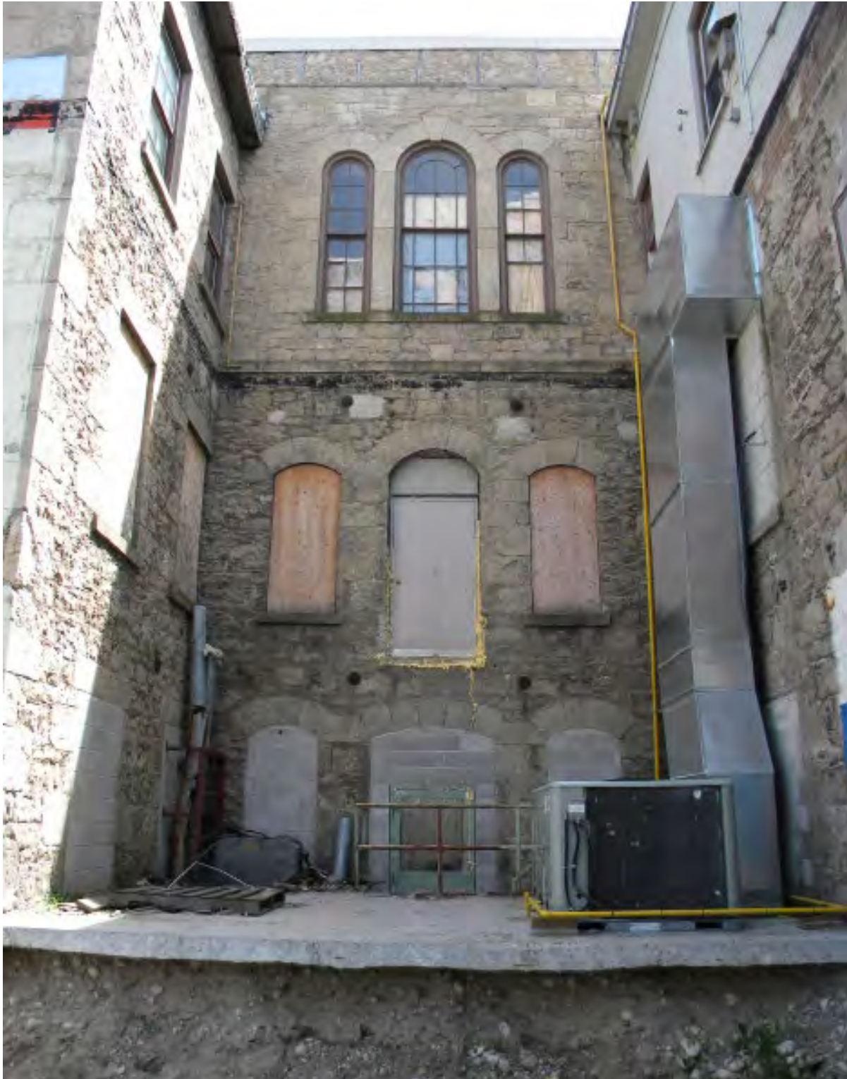
31. Building #2c, North Elevation, 2014 (Source: ERA)
