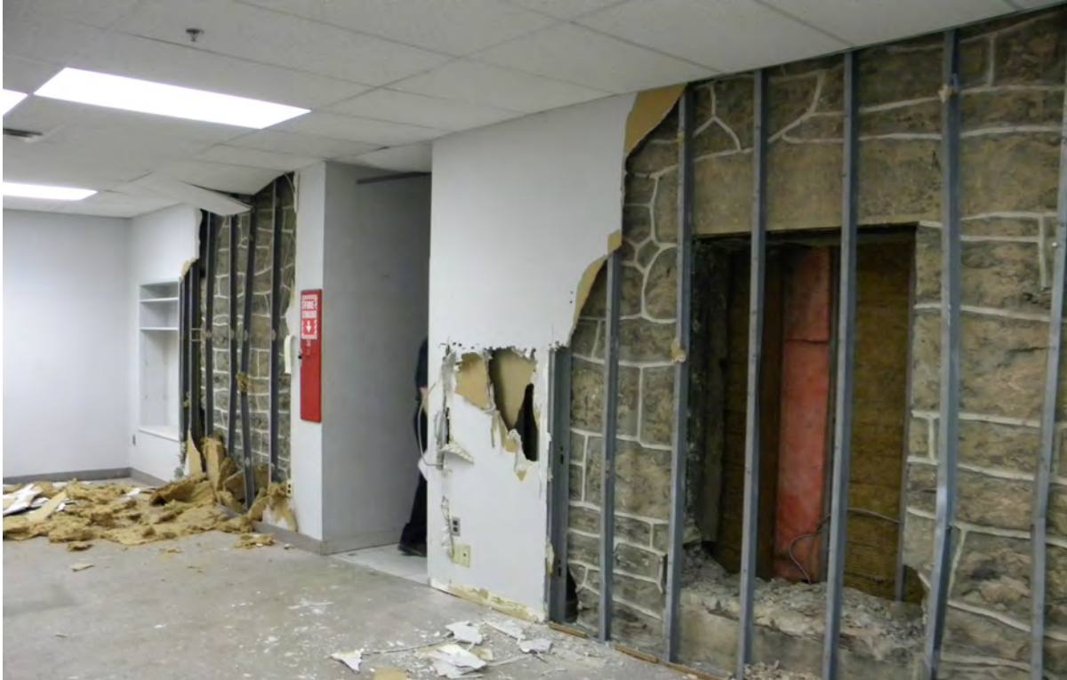
21. Building #2a, East Elevation, original exterior wall (Source: City of Guelph)
