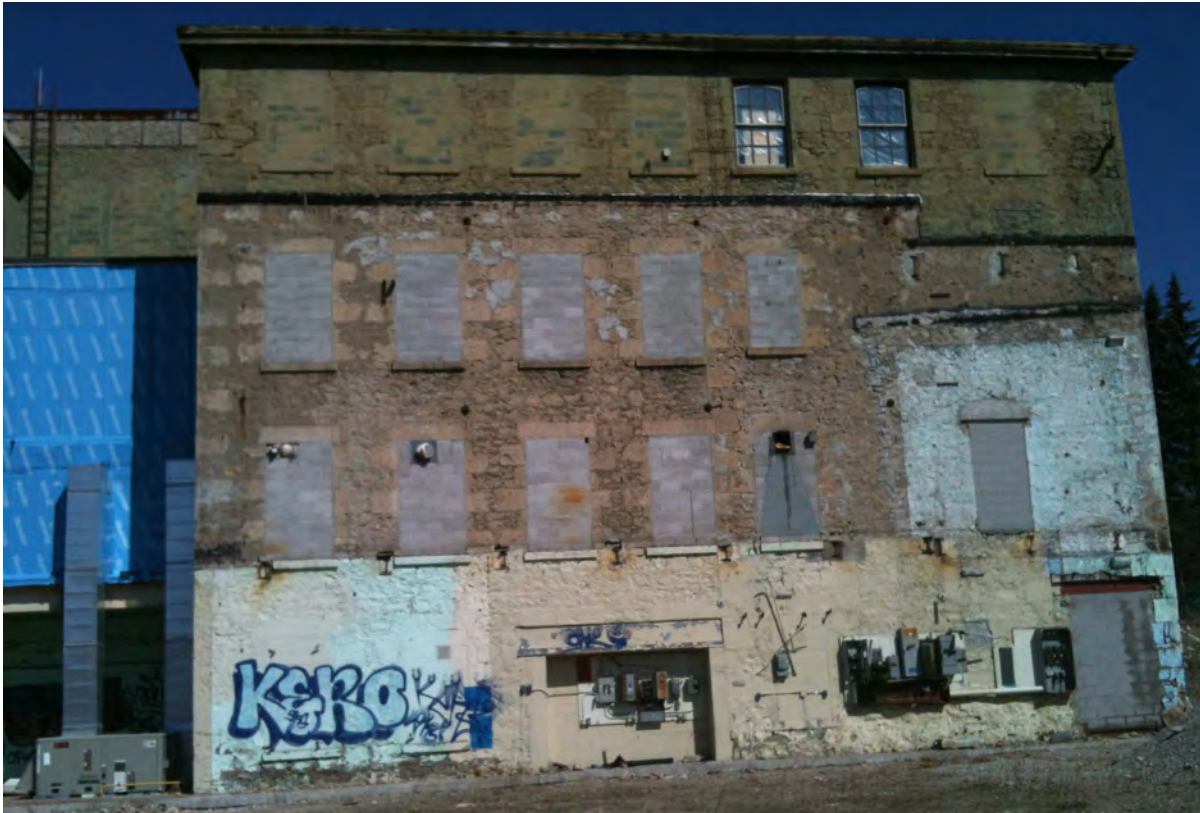
40. Building #2d, South Elevation, 2014 (Source: ERA)
