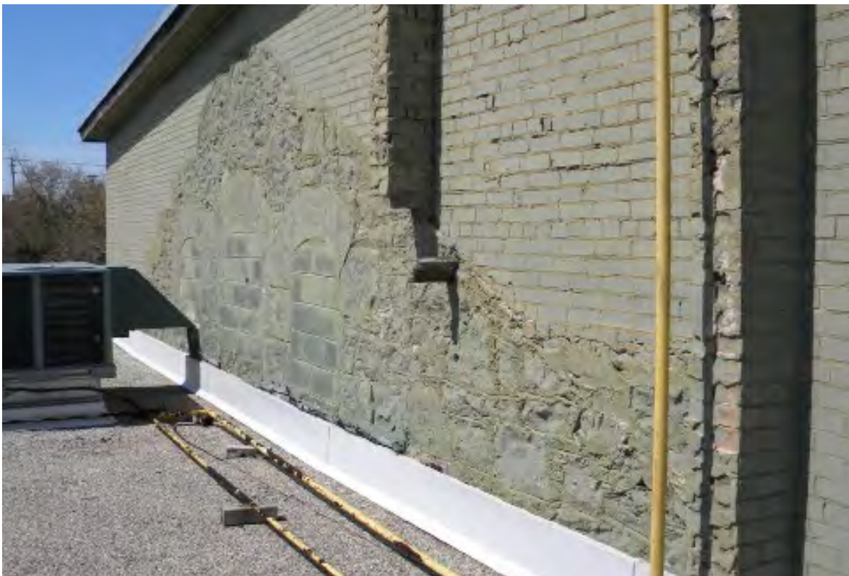
24. Building #2b, South Elevation, original roof gable (Source: City of Guelph)
