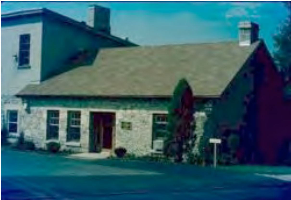
View of former distillery buildings after renovations by W C Wood Company, 1973 and 1980. Source: Couling Collection, Wellington County Museum and Archives
