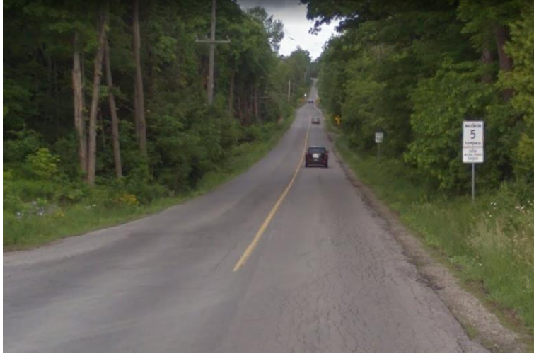
Figure 5. Looking west (down slope) along Niska Road from Pioneer Trail (on left) to Speed River. Source: Google Earth 2016 image
