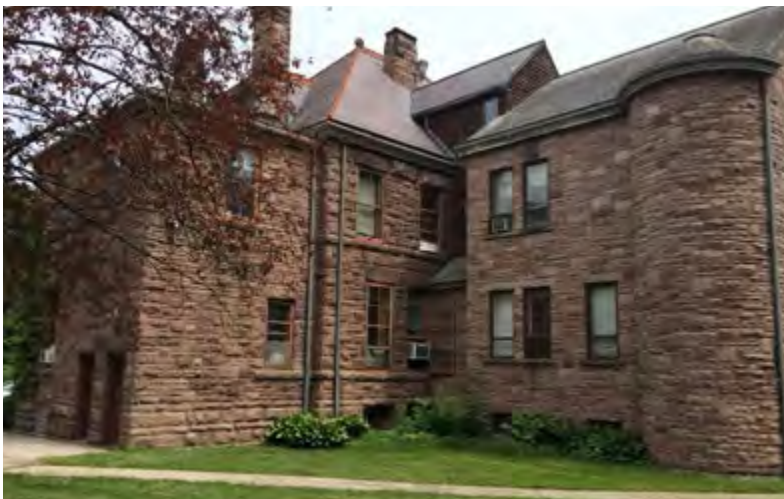
20. View of Riverslea's north elevation (Source: ERA).
