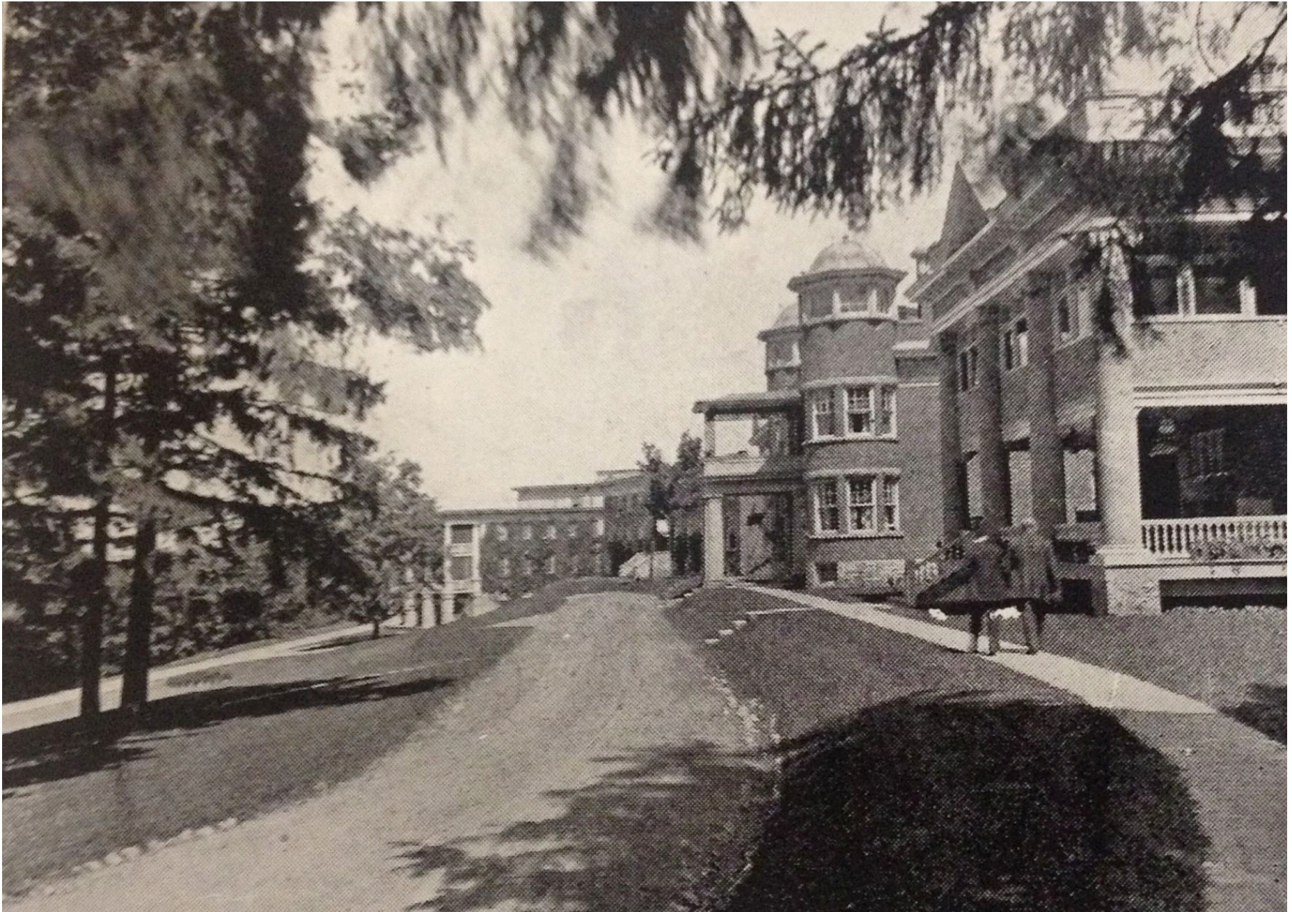
62 Archival image of the west elevation of historic buildings within Homewood campus [Source: Guelph Public Library]
