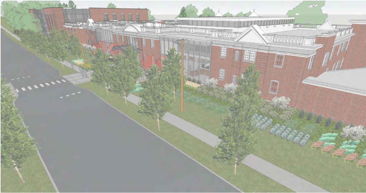
30. Rendering showing the proposed alterations to the Manor's Delhi Street elevation, including new curtain-wall additions, removal of the existing corridor addition, and new entry sequence. Looking southwest (Source: Cornerstone Architecture).
