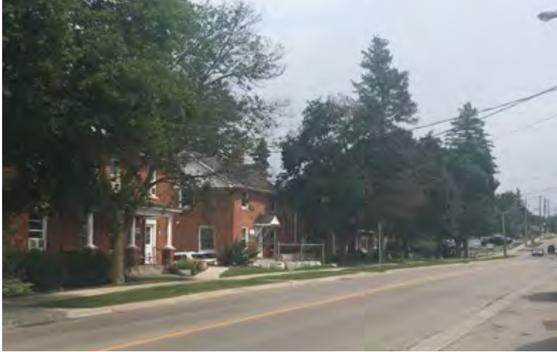
23. View of the auxiliary buildings on the east side of Delhi Street, looking southeast (Source: ERA).
