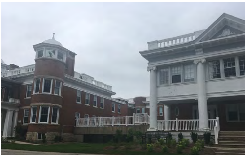
14. Partial view of the Manor building's west elevation, showing the raised basement addition between the south and central wings (Source: ERA).
