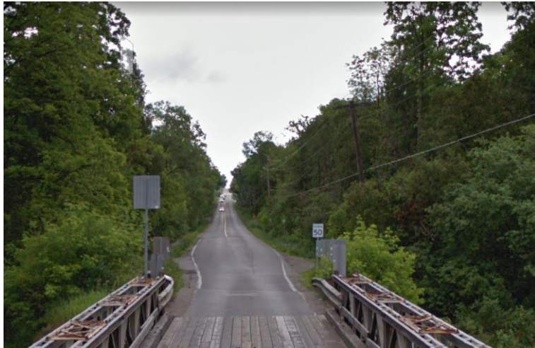
Figure 6. Looking east (up slope) from Niska Road bridge to Pioneer Trail. Source: Google Earth 2016 image
