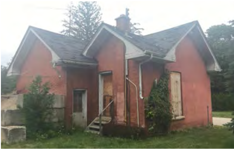
22. View of one of the Riverslea outbuildings, looking south (Source: ERA).
