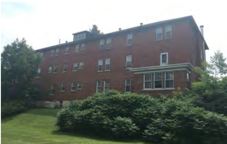
25. View of the Nurses' Residence's east elevation (Source: ERA).
