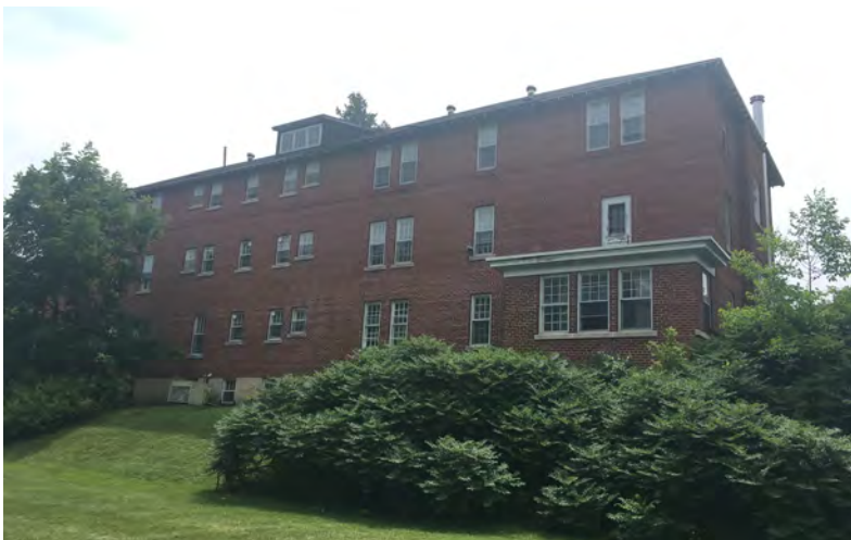
36. View of the Nurses' Residence's east elevation (Source: ERA).
