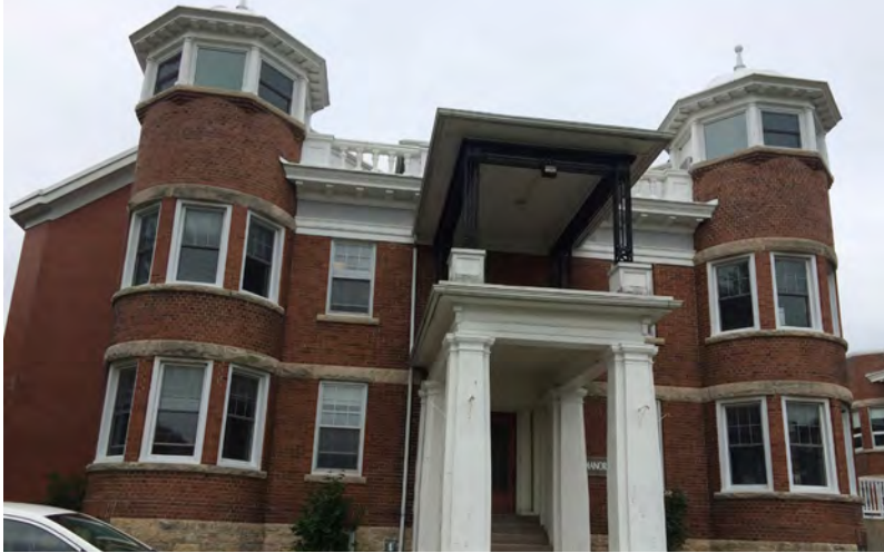
15. Partial view of the Manor building's west elevation, showing the central wing (Source: ERA).
