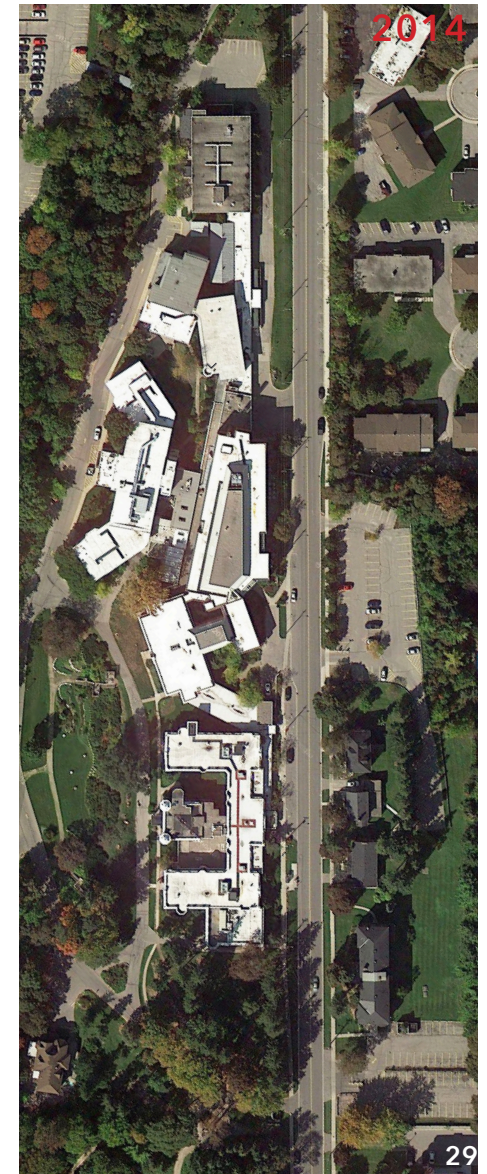
Aerial image of the Homewood campus [Source: Google Earth]
