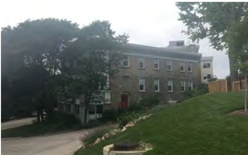
13. View of the Colonial's south wing, looking north from the river valley terrace (Source: ERA).
