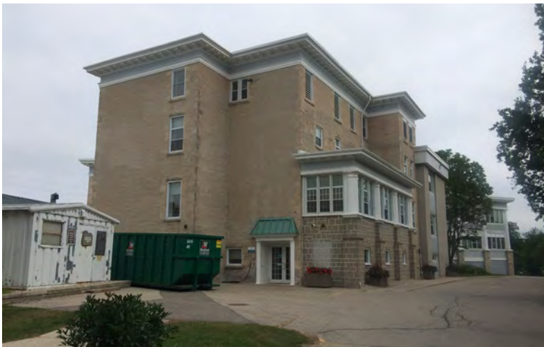
22. View of the Vista's north and south elevations, looking south (Source: ERA).
