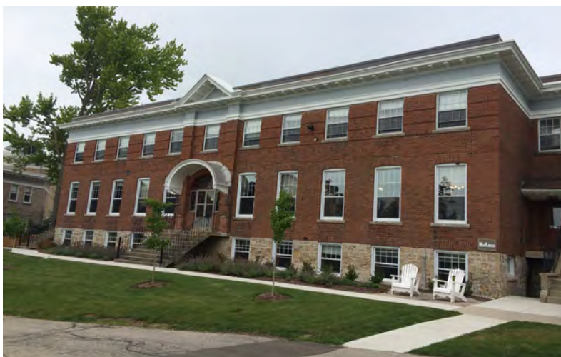
17. View of the MacKinnon's west elevation (Source: ERA).
