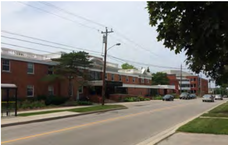
9. View of the Manor building's east elevation, looking north along Delhi Street (Source: ERA).
