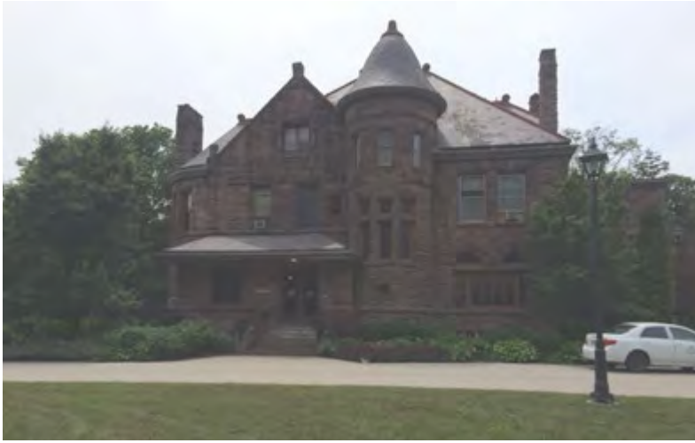
19. View of Riverslea's east elevation (Source: ERA).
