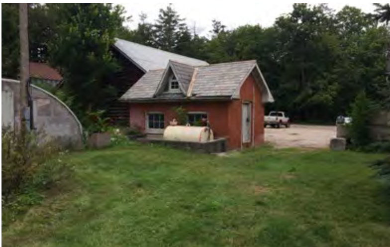
21. View of one of the Riverslea outbuildings, looking north (Source: ERA).
