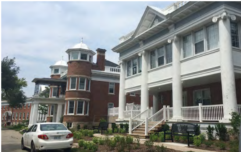
13. Partial view of the Manor building's west elevation (Source: ERA).
