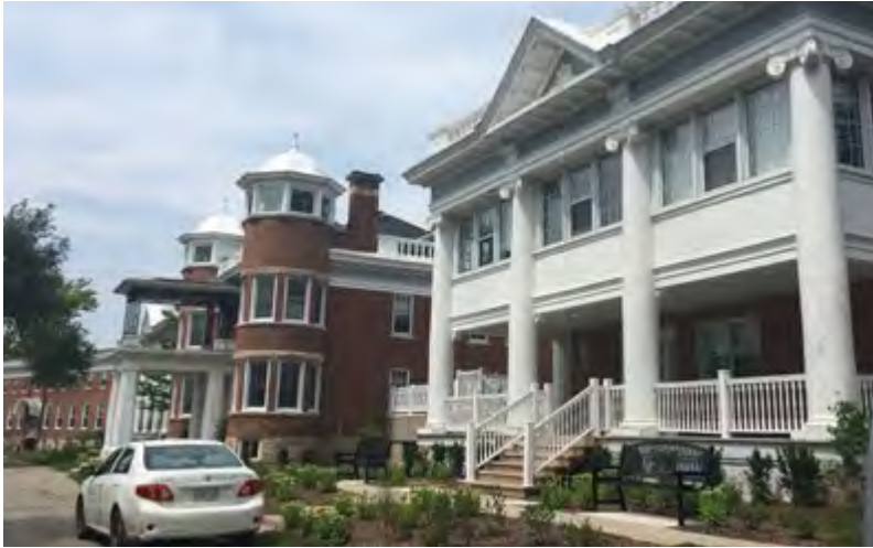
11. Partial view of the Manor building's west elevation (Source: ERA).
