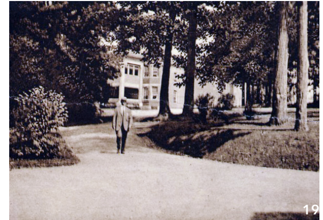
18 View toward the Speed River from The Manor Building (c. 1923)
