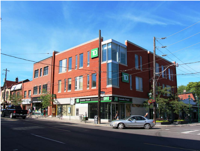
Low-rise mixed-use building with commercial uses at street level.
