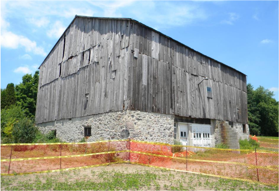
Figure 6 - Weir farm barn, south corner (Photo: S. Robinson, Planning Services)
