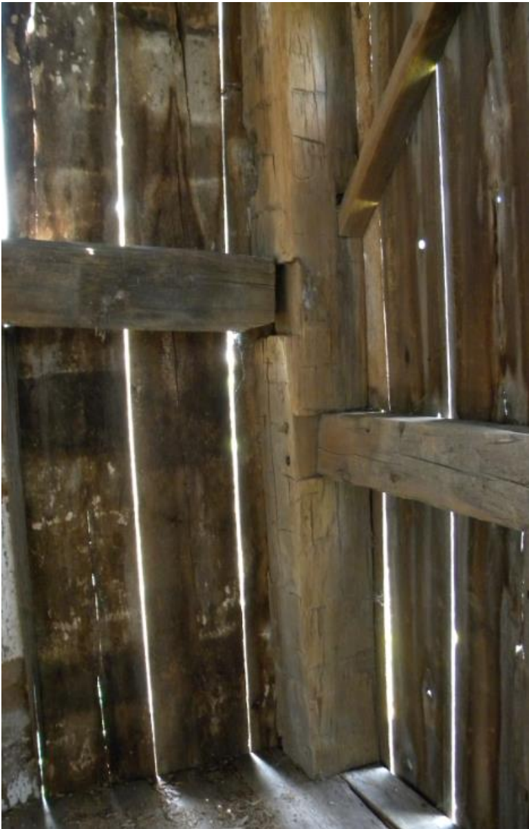
Figure 7 – Heavy timber framing in west corner of main floor. (Photo: S. Robinson, Planning Services)
