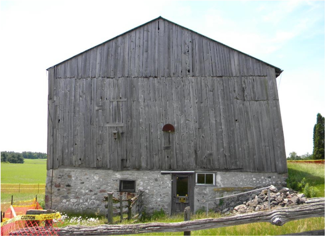
Figure 5 - Weir farm barn, northeast gable wall with man door to lower level. (Photo: S. Robinson, Planning Services)
