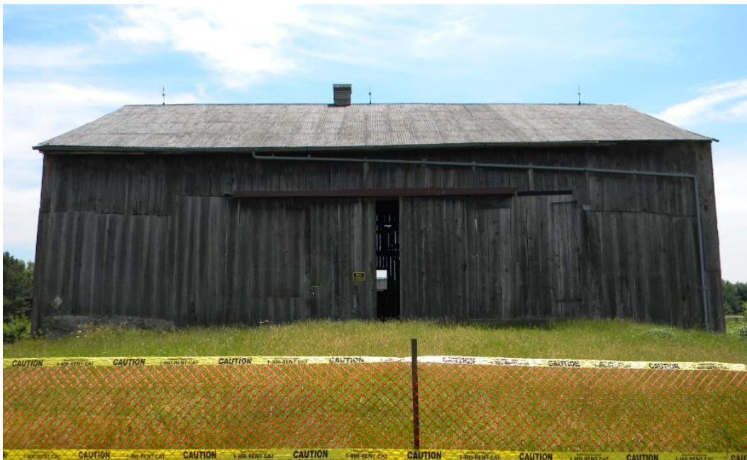
Figure 4 - Weir farm barn, northwest elevation with bank to main doors. (Photo: S. Robinson, Planning Services)
