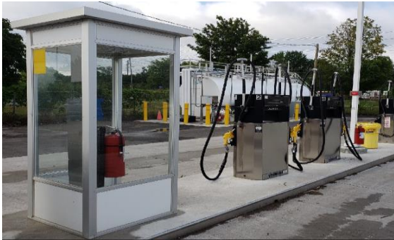
Fuel pump replacement
