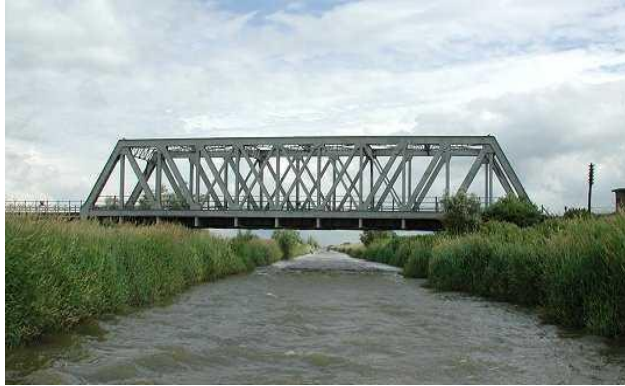
Covered Steel Through Truss Bridge
