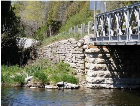
Loss of top wall and mortar, evidence of severe settlement
