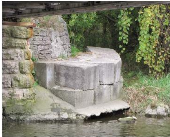
Evidence of continuing settlement due to river undermining and undercutting
