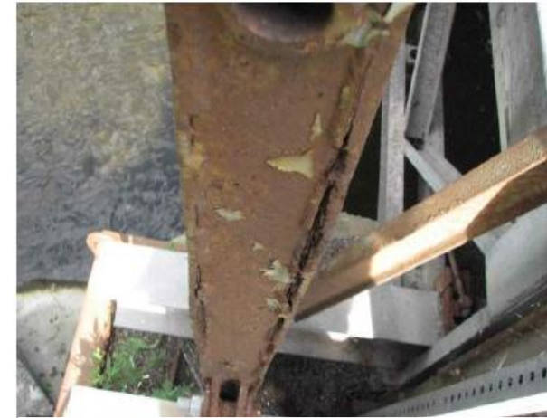
Evidence of severe corrosion evident throughout the structure
