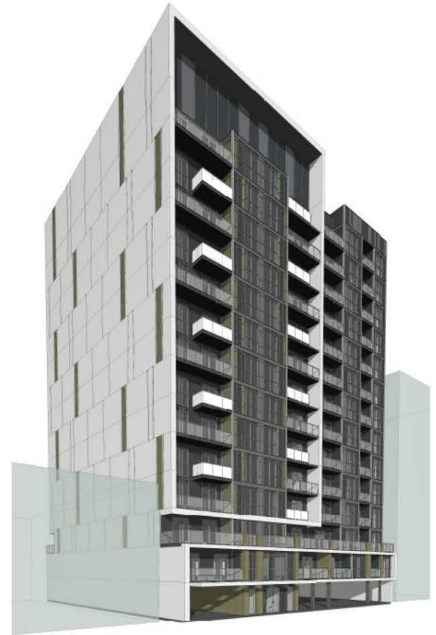
② PEDESTRIAN VIEW TO NORTH WEST ON BAKER ST
