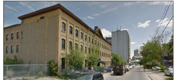
View along Yarmouth Street (to south)
