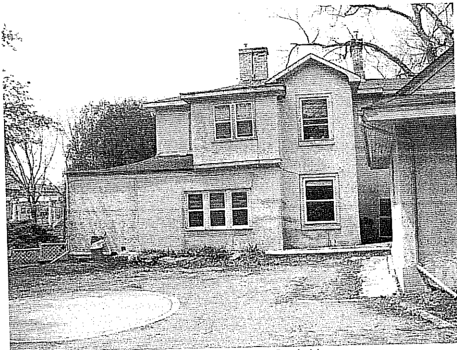
Figure 4.0: Northwest elevation featuring the twin-flued chimneys
