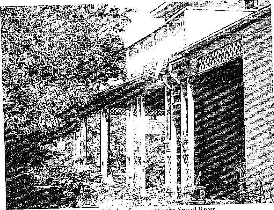
Figure 5.0: Image of the verandah that fronts onto the Speed River
