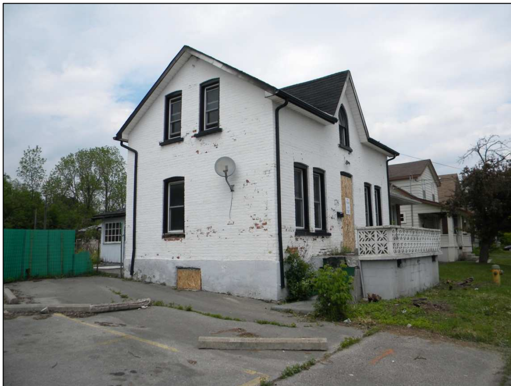
(178 Elizabeth Street - Photos taken by R. Harris, June 2014)
