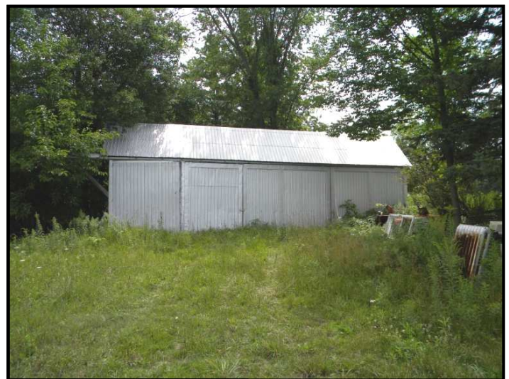
Figure 5.2.7: Exterior view of storage shed
