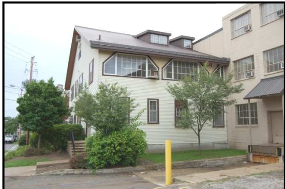
Figure 4.3: 72 Farquhar, northwest elevation
