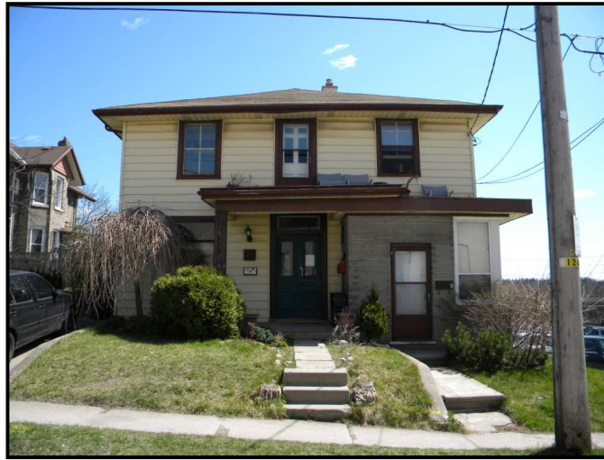
Figure 5.1: Photo of 81 Farquhar Street.
