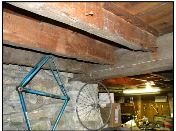
Figure 5.8: Floor beams in the basement
