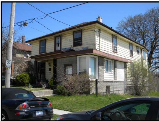
Figure 5.3: 81 Farquhar Street, front elevation.
