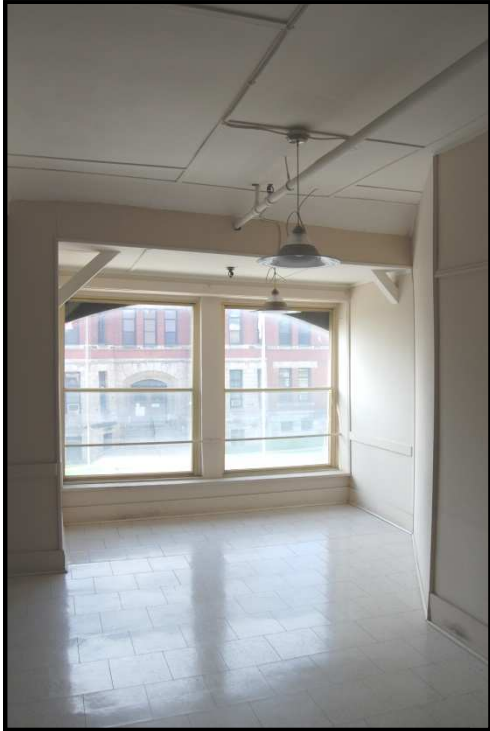
Figure 4.5: Second floor window in west elevation. Note the Armory building through the window
