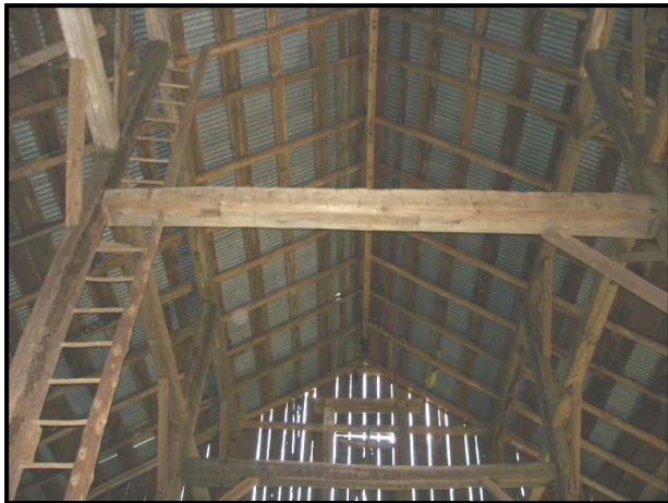
Figure 5.2.2: Interior structure of the bank barn
