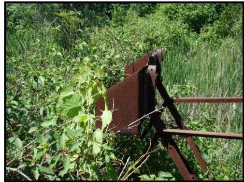
Figure 5.3.2: Detail of one scoop of dash wheel
