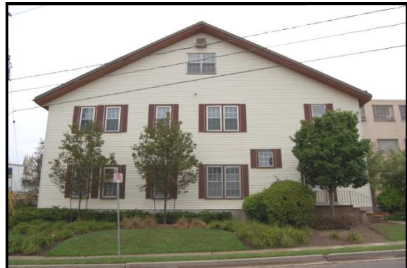
Figure 4.2: 72 Farquhar, west elevation
