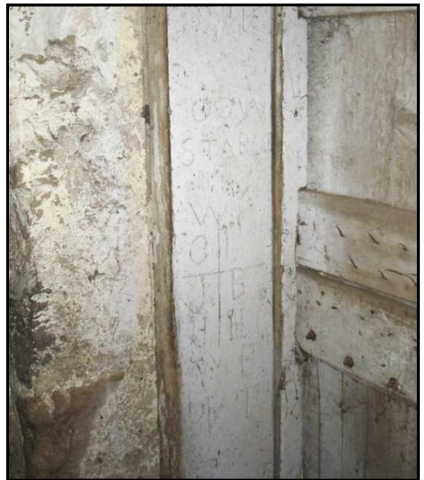
Figure 5.2.3: Carved beam showing the initials of the builders of the bank barn
