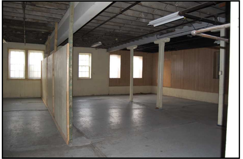
Figure 4.6: Main floor level inside Drill Hall
