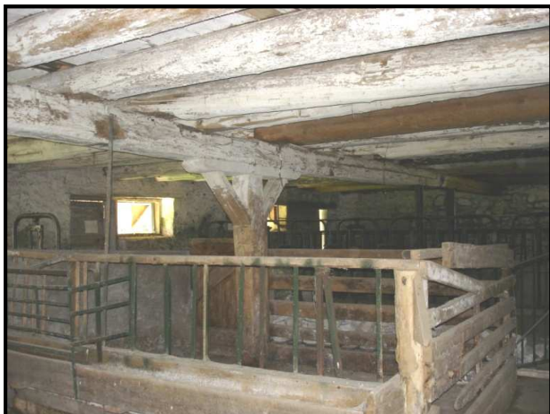
Figure 5.2.4: Interior of the bank barn lower section upper section. Note the original massing and internal volume
