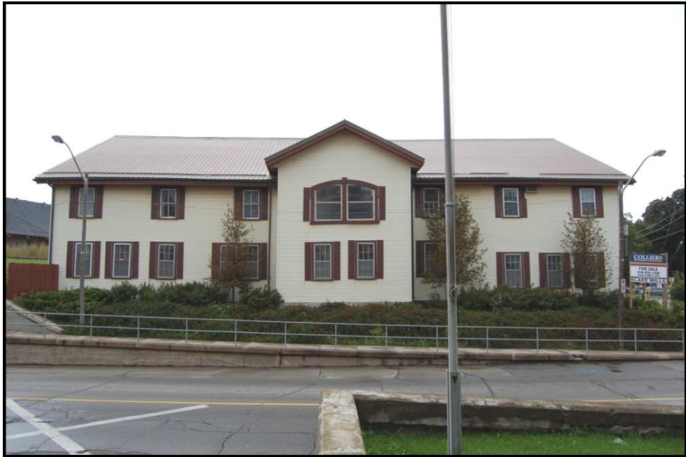
Figure 4.1: 72 Farquhar, north elevation
