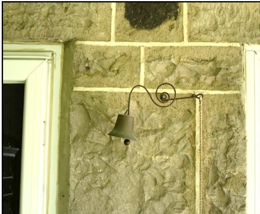
Figure 5.1.9: Detail of the original doorbell
