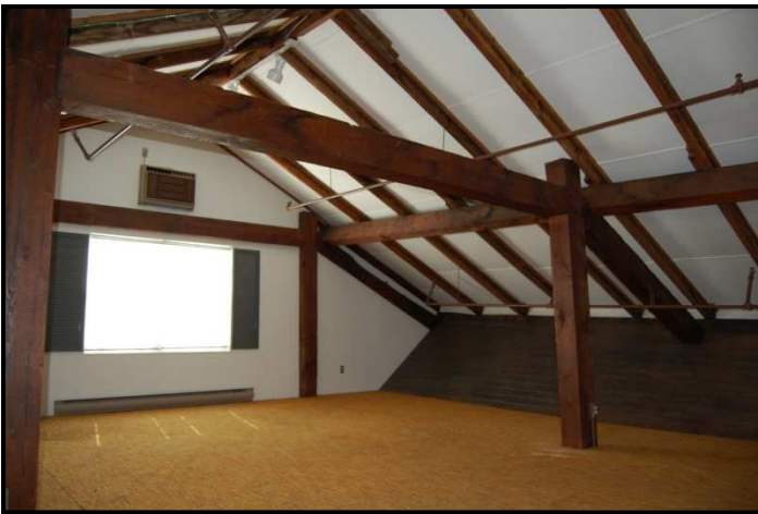
Figure 4.7: View of attic showing timber framing.
