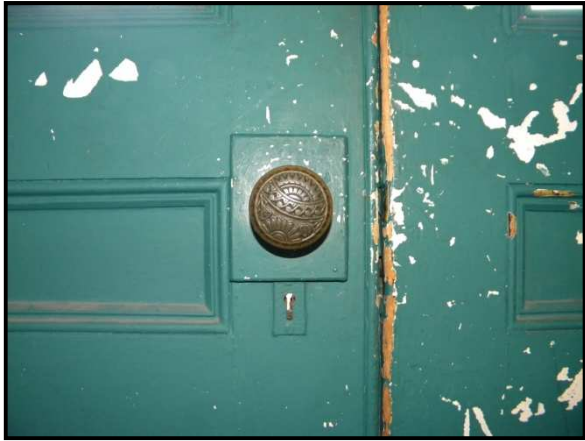
Figure 5.5: Door knob. Interior view of two-leaf half-glass front door.
