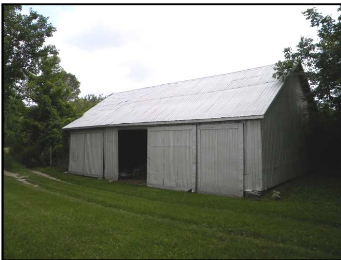
Figure 5.2.6: Exterior view of drive shed
