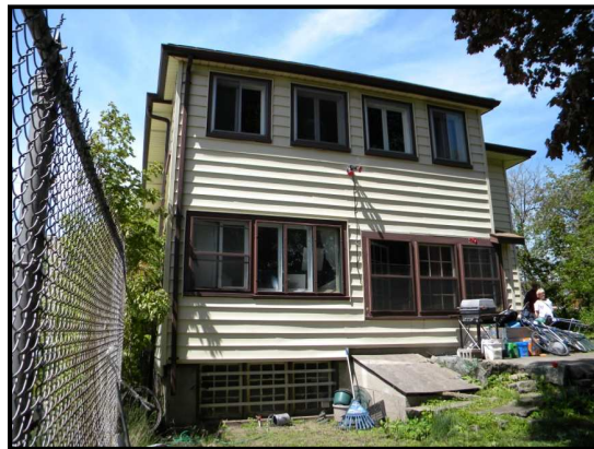
Figure 5.4: 81 Farquhar Street rear elevation.
