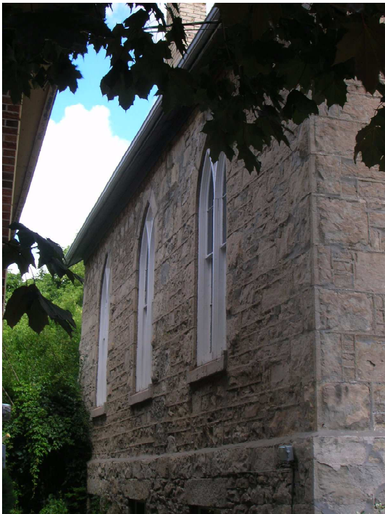
Figure 8. North Elevation Featuring Symmetrically-placed Windows
