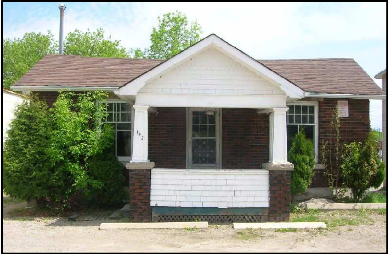
Detached dwelling proposed to be demolished - 192 Waterloo Avenue
