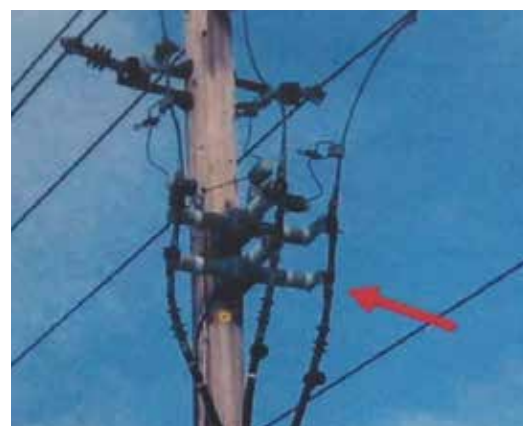
"Hot spots" indicate equipment that is starting to degrade and requires replacement.
