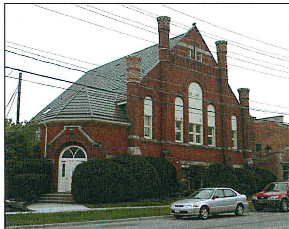
200 Woolwich Street, Guelph
