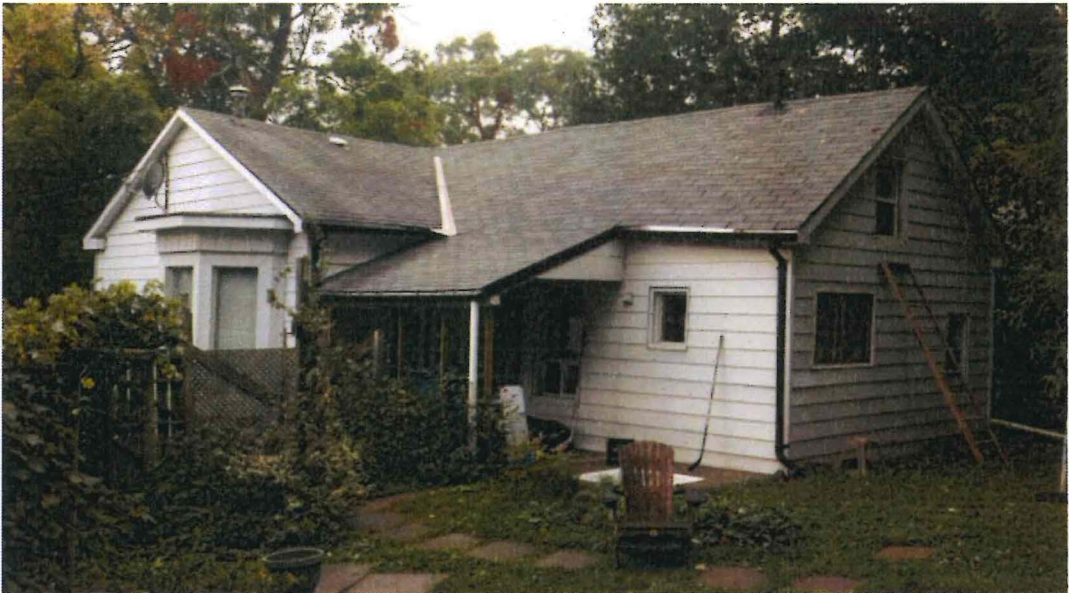
Figure 3 - 251 Arthur Street North – rear
