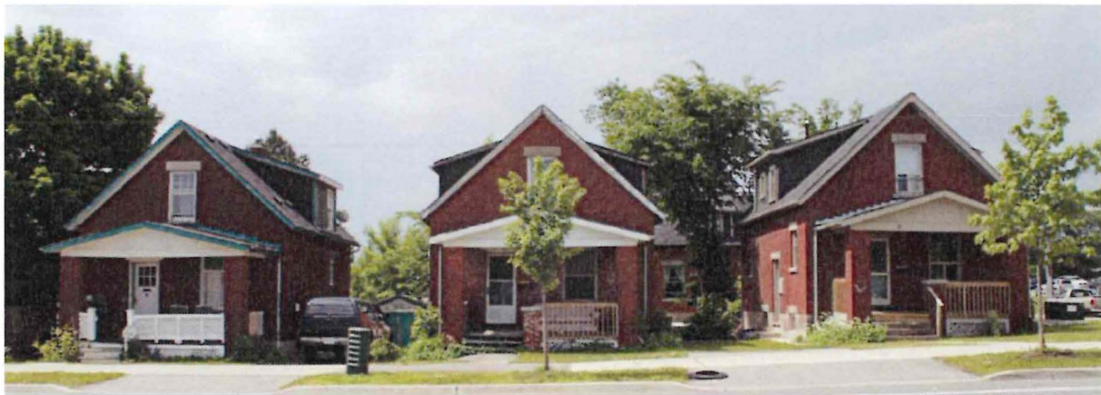
Figure 2 – 41, 43 and 45 Wyndham Street South (Photo: CHC Ltd.)
