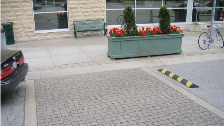
Traffic calming techniques such as textured paving crosswalks help to slow traffic to create a safer pedestrian experience.
