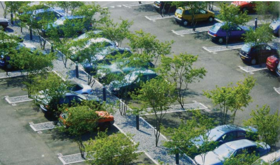
Permeable paving and bio-filtration trenches typically store, filter and slowly release water at a regulated rate into the ground.
