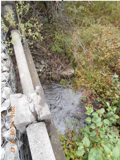
Upstream face of Clythe Creek crossing
