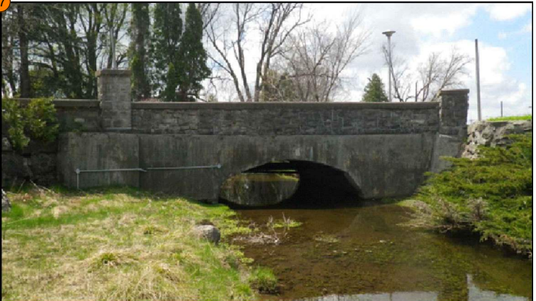
Feature #17: Stone and concrete road bridge (listed, non-designated significant feature). No impact to feature anticipated as a result of proposed channel works, existing capacity dimensions to be maintained.
