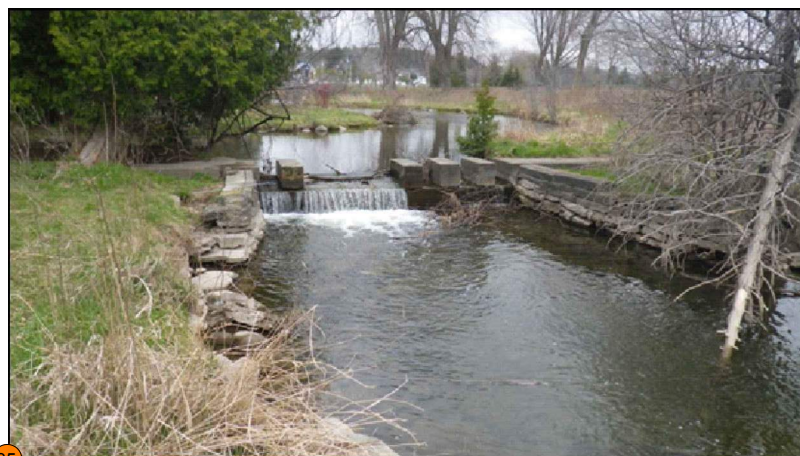
35 Feature #35: Concrete and stone weir (potential significance). Feature to be removed as a result of proposed channel works.
