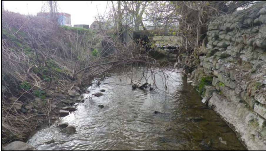
21. Reach HC-1: Looking downstream towards York Road culvert crossing.
