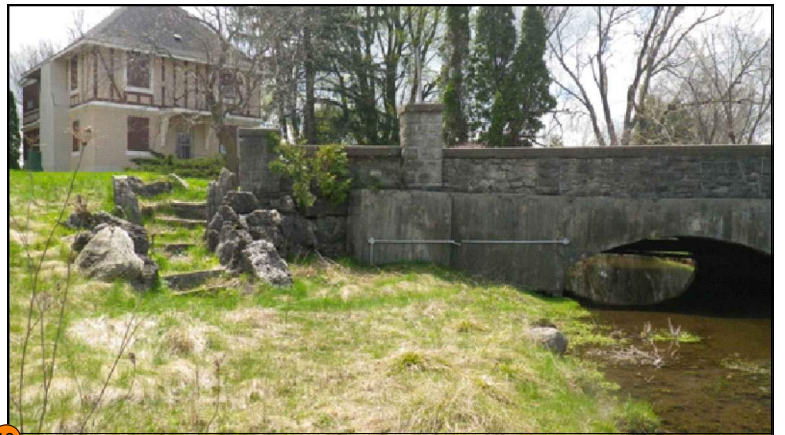
Feature #18: Fieldstone steps to the south of road bridge (listed, non-designated significant feature). No impact to feature anticipated. No impact to feature anticipated.
