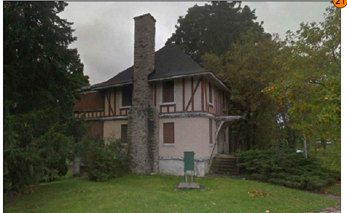
Feature #21: Willowbank Hall (listed, non-designated significant feature). Feature is located within the floodplain and will not be impacted by proposed channel works.
