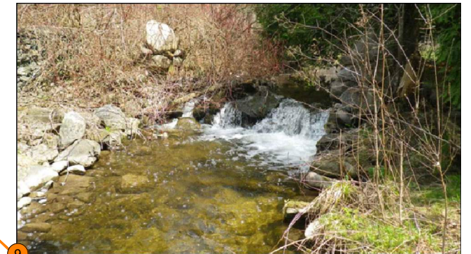
Feature #9: Fieldstone weir (listed, non-designated significant feature). No impact to feature anticipated. Retaining wall required to be built to protect/maintain feature from anticipated roadway grading limits.
