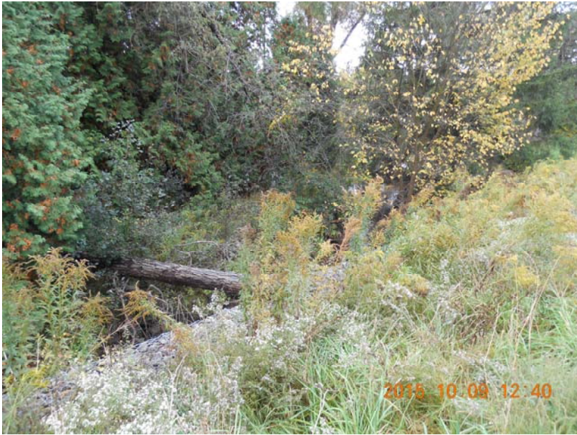
Gabion baskets next to roadway
