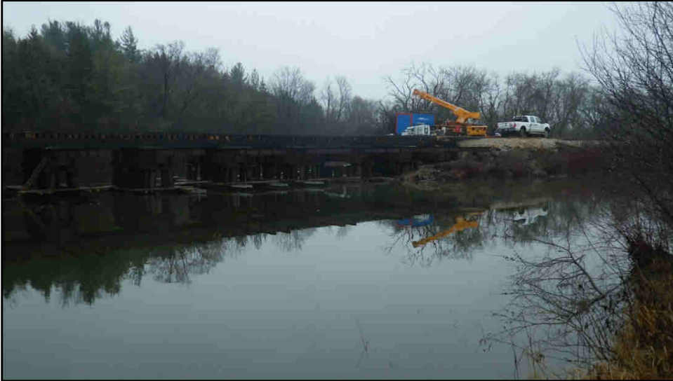
19. Looking downstream along the Eramosa River towards the Clythe Creek confluence located to the right. Railway embankment and bridge structure crossing the Eramosa River also present in background.
