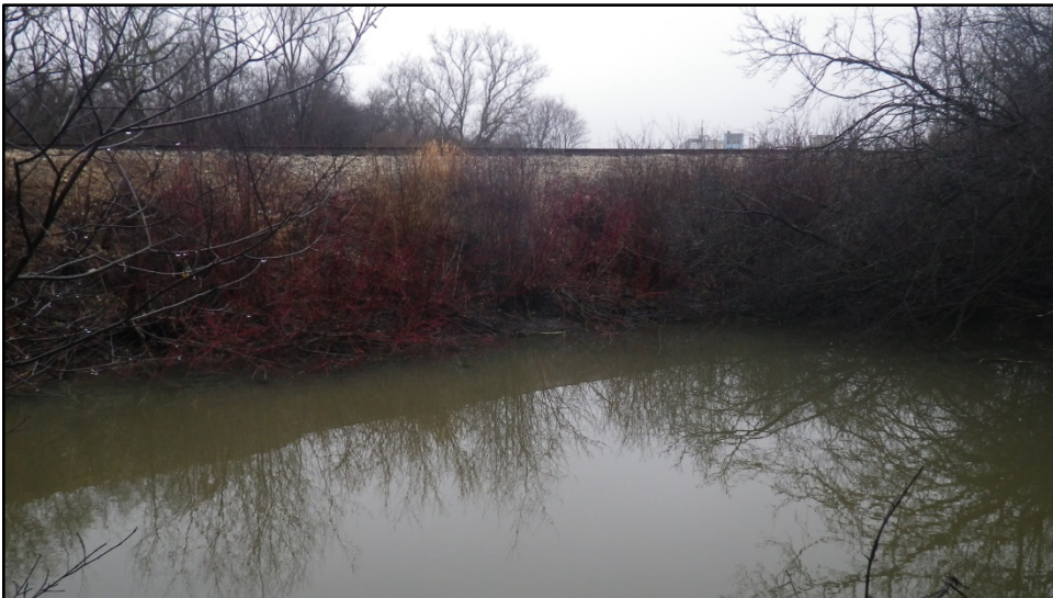
18. Clythe Creek flows immediately adjacent to railway embankment; embankment protection appears to be limited to vegetation. Water turbidity changes colour to appear more beige.
