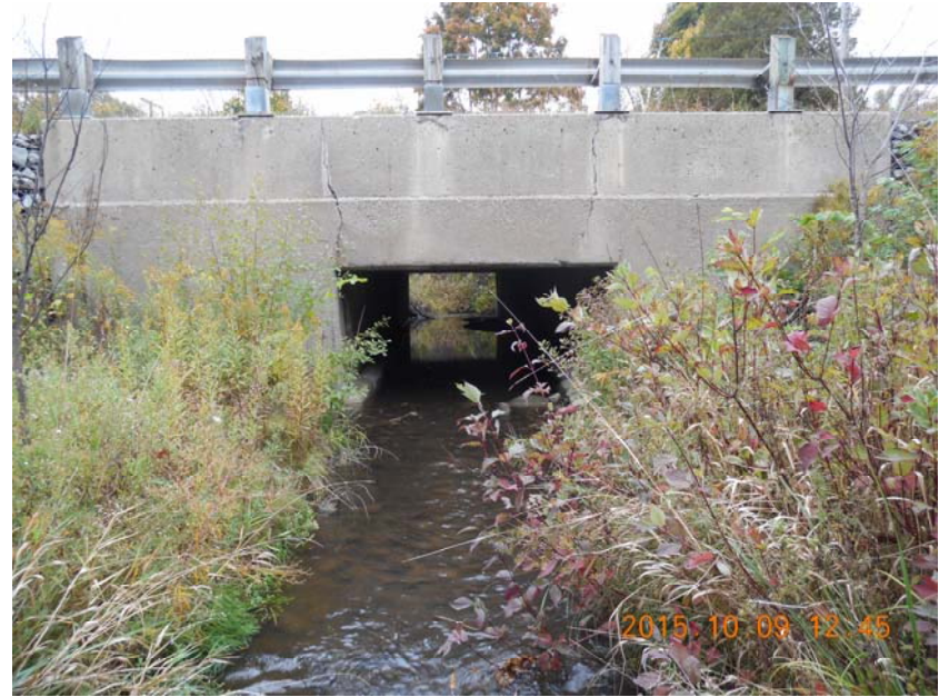
Downstream face of Clythe Creek
