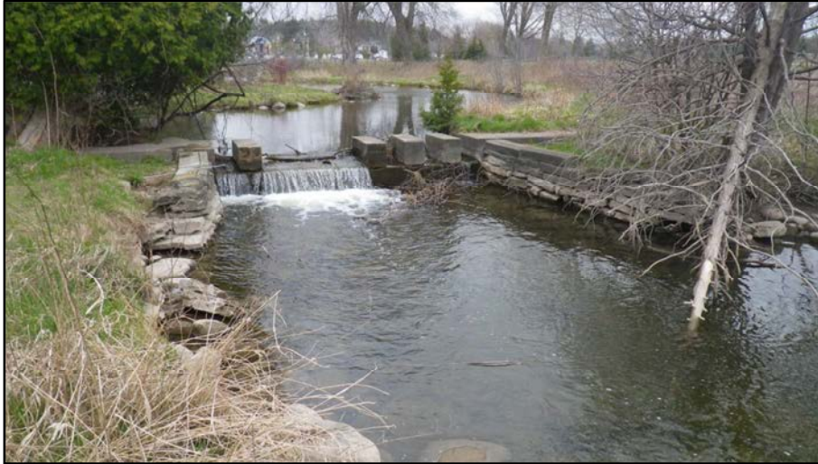
17. Reach C-10: Flow splitter structure installed along Clythe Creek.
