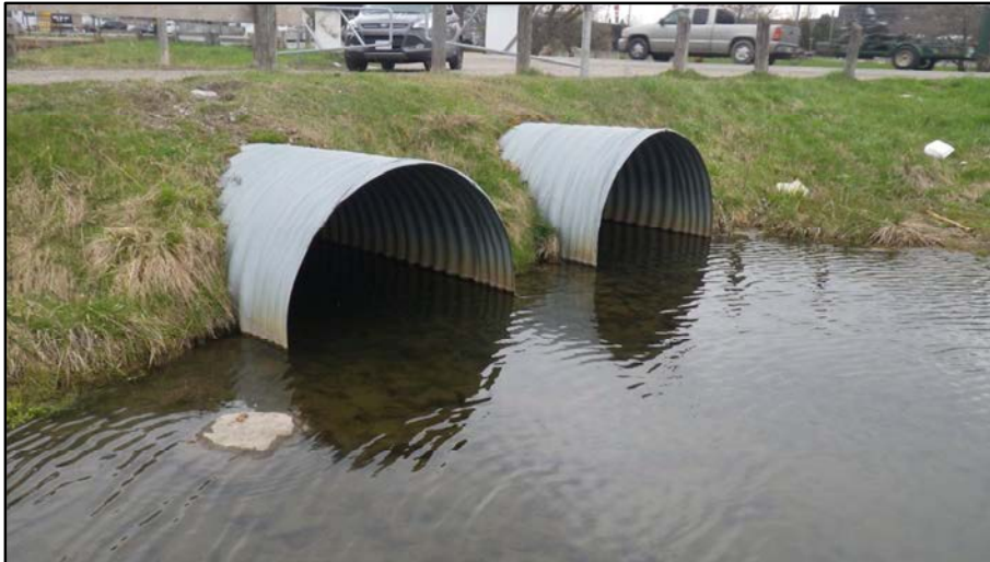
15. Reach C-9B: Double CSP culvert at entrance to Jaycee Park.
