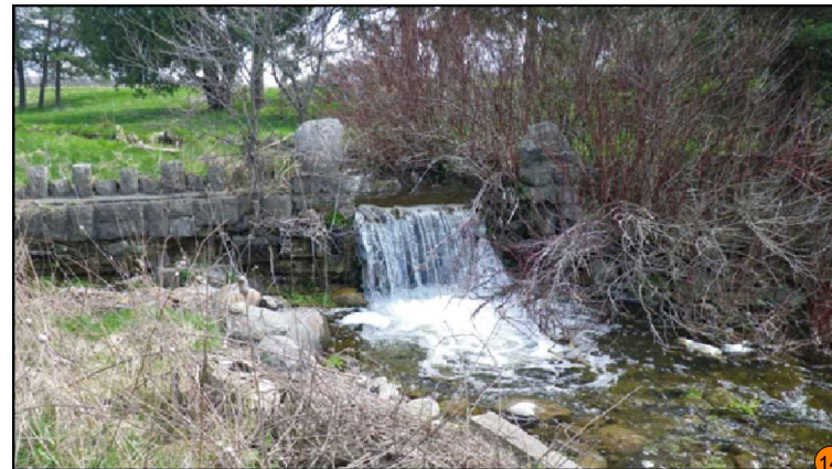
Feature #14: Fieldstone weir with cut stone terrace wall (listed, non-designated significant feature).
