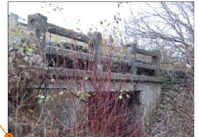
Feature #2: Reinforced concrete road bridge railing (potential significance). Feature to be modified to accommodate road widening works.
