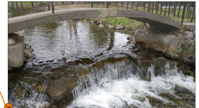
26 Feature #26: Fieldstone weir (listed, non-designated significant feature). No impact to feature anticipated.
