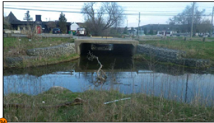
34 Feature #34 (not considered cultural heritage feature): Box culvert at confluence of Clythe Creek and Hadati Creek. Potential culvert extension to accommodate roadway grading requirement and CSP replacement.
