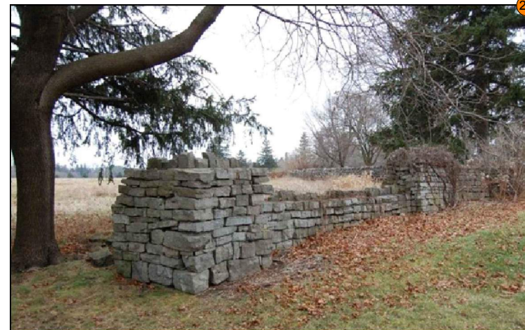
Feature #20: Ashlar dry stone wall (listed, non-designated significant feature). Feature is located within the floodplain and will not be impacted by proposed channel works.
