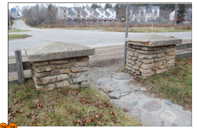
28, 29 Feature #28 and #29: Limestone pillars with wood board fencing leading to main entrance (potential significance). Potential for feature to be modified as a result of roadway grading requirements.
