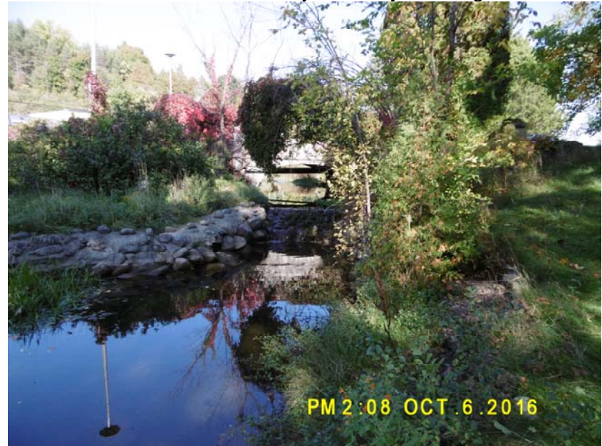
Lined channel downstream of former Reformatory driveway
