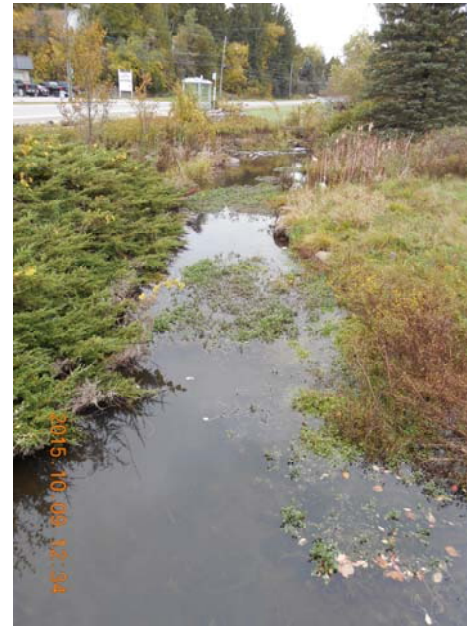
Creek immediately upstream of former Reformatory driveway Note creek is in a backwater condition
