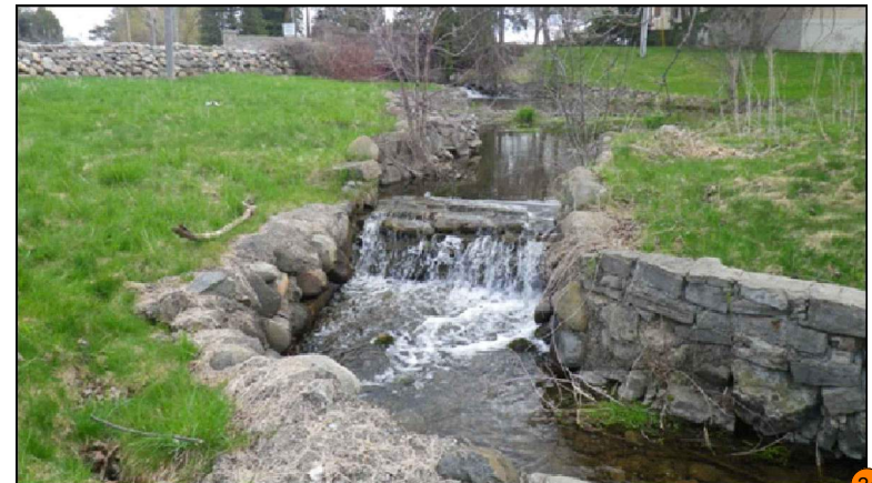
Feature #24: Fieldstone weir (listed, non-designated significant feature). Feature is a substantial barrier to fish passage and limiting factor in overall channel function and health. Feature to be taken off-line and disconnected during low-flow stages as a result of proposed channel realignment. An overflow channel will be incorporated so that the feature will be reconnected during high-flow stages (i.e., flows greater than the 2yr discharge).
