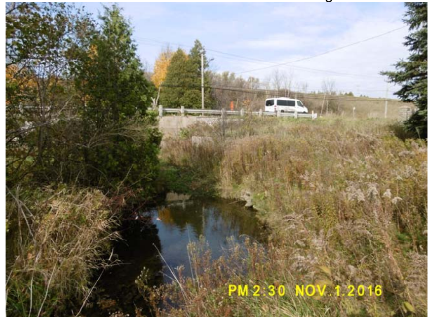
Pool feature immediately downstream of culvert
