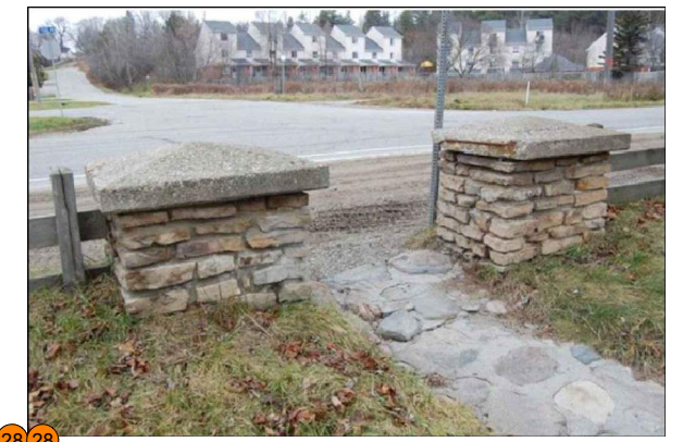
28, 29 Feature #28 and #29: Limestone pillars with wood board fencing leading to main entrance (potential significance). No impact to feature anticipated as a result of proposed channel works.
