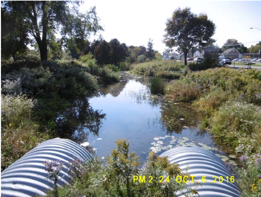
Downstream of twin CSP culverts
