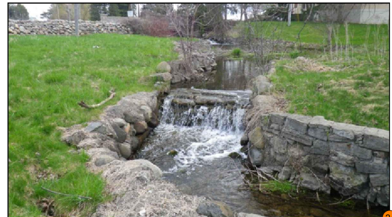
Feature #24: Fieldstone weir (listed, non-designated significant feature). Feature is a substantial barrier to fish passage and limiting factor in overall channel function and health. Feature to be taken off-line/disconnected from active flow as a result of proposed channel works. Potential for feature to be impacted as a result of required grading/fill as a result of proposed channel works.
