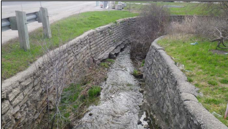
25. Reach HC-1: Channel immediately downstream from Beaumont Cres. Both banks are lined with concrete and shale bricks. Bank protection is undermined along meander bend.
