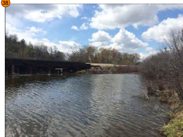
38 Feature #38: GJR railway bridge (potential significance). No impact to feature anticipated.
