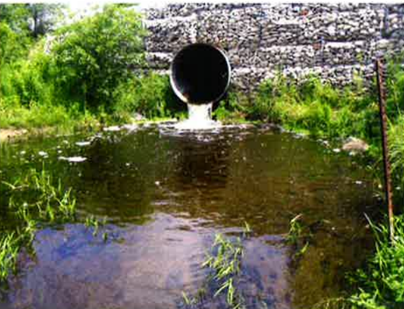
Photo 5: Perched culvert at Watson Road North (Site 4) presents a significant barrier to fish migration. Large schools of minnows (and minnow traps) can usually be observed in the pool below the culvert.
