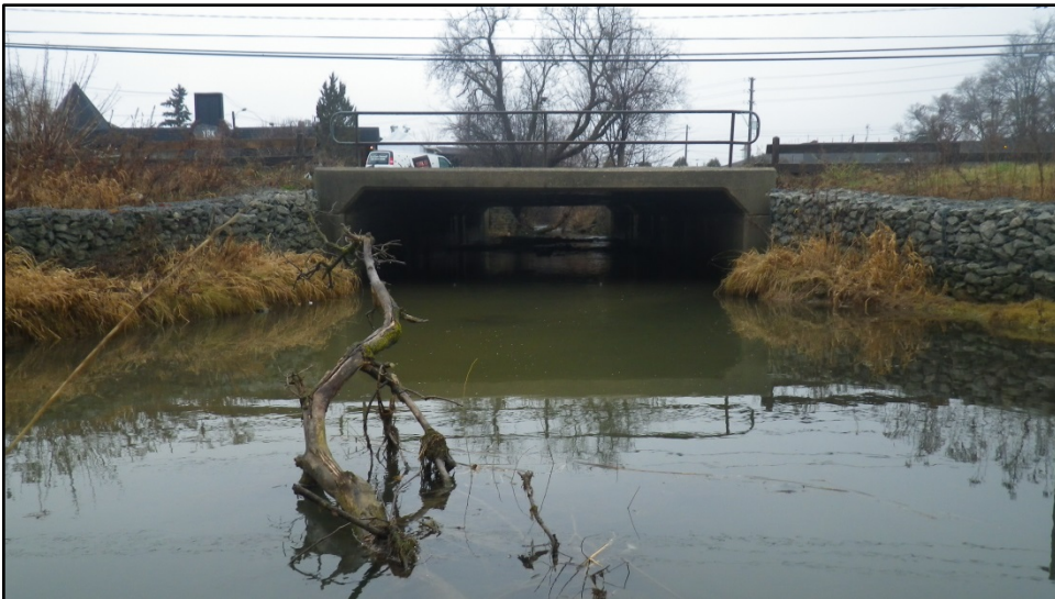
14. York Road crossing of Hadati Creek; structure is a concrete box culvert; gabion wing-walls protect the banks.
