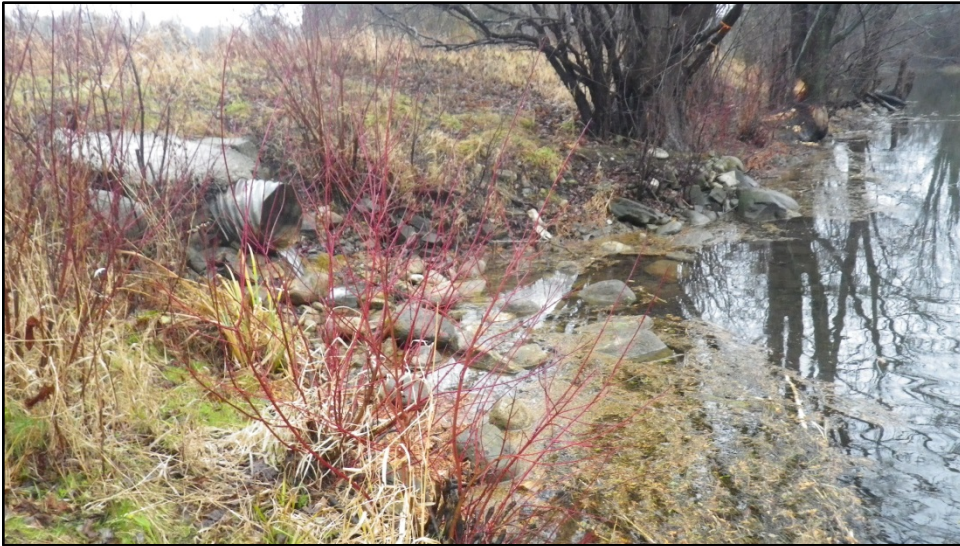
21. South pond connection to the Eramosa River through a CSP pipe elevated approximately 30 cm; the pipe appears to be blocked, and discharge is minimal.
