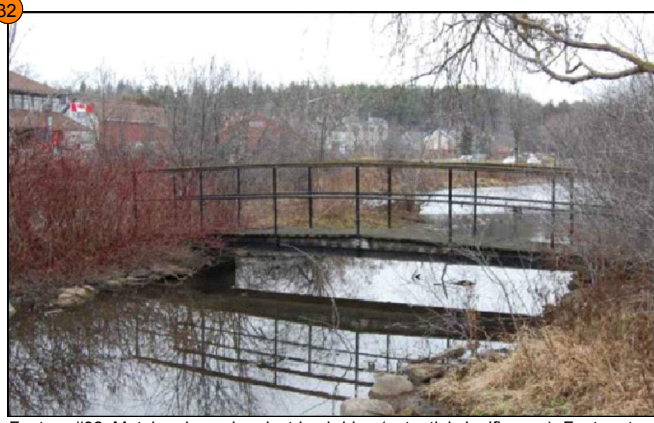
32 Feature #32: Metal and wood pedestrian bridge (potential significance). Feature to be removed as a result of proposed channel works.
