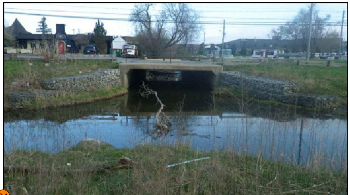
34 Feature #34 (not considered cultural heritage feature): Box culvert at confluence of Clythe Creek and Hadati Creek. Potential culvert extension to accommodate roadway grading requirement and CSP replacement.
