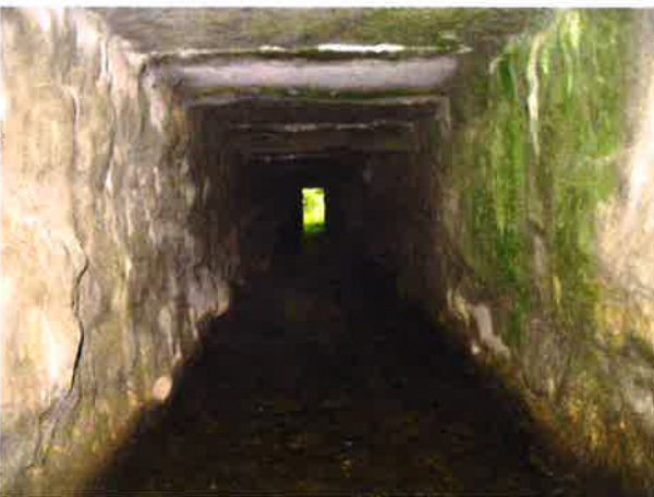
Photo 11: A long, dual-channelled, concrete culvert diverts the Creek from the north to the south side of the railway line.
