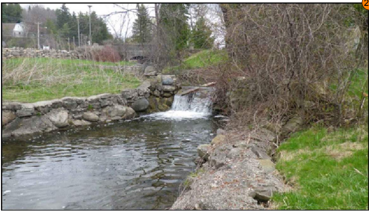
Feature #23: Fieldstone weir (listed, non-designated significant feature). Feature is a substantial barrier to fish passage and limiting factor in overall channel function and health. Feature to be taken off-line and disconnected during low-flow stages as a result of proposed channel realignment. An overflow channel will be incorporated so that the feature will be reconnected during high-flow stages (i.e., flows greater than the 2yr discharge).
