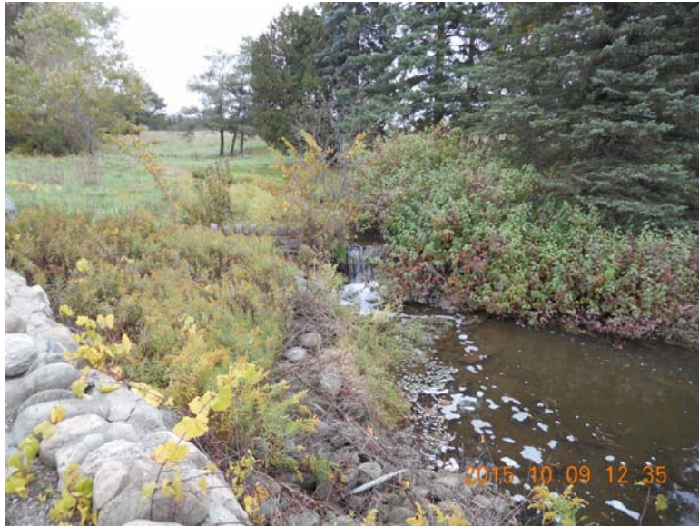
Cultural heritage wall and drop structure just west of former Reformatory driveway
