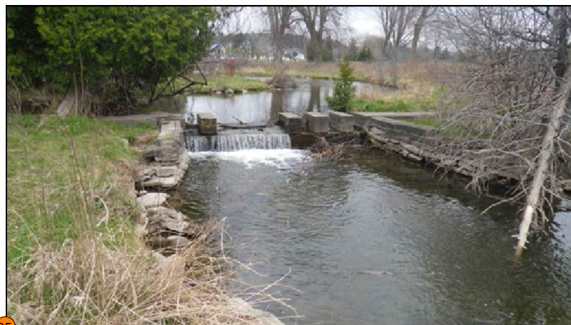
35 Feature #35: Concrete and stone weir (potential significance). Feature to be taken off-line and disconnected during low-flow stages. An allowance for overflow capabilities will be incorporated so that the feature will be reconnected during high-flow stages (i.e., flows greater than the 2yr discharge).
