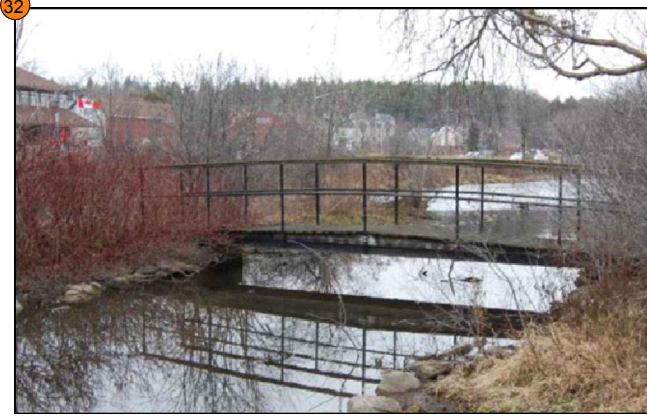
32 Feature #32: Metal and wood pedestrian bridge (potential significance). Feature is likely to be modified or removed as a result of proposed channel works.
