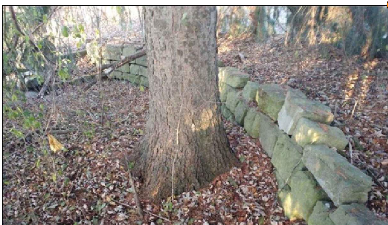
Feature #12: Ashlar limestone wall (listed, non-designated significant feature). Part of feature impacted by proposed creek realignment.
