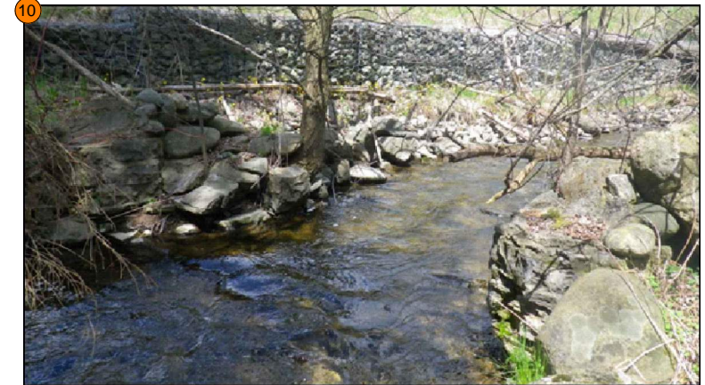
Feature #10: Fieldstone weir (listed, non-designated significant feature). Retaining wall required to be built to protect/maintain feature from anticipated roadway grading limits. Part of flagstone to be removed to accommodate retaining wall.
