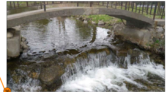
26 Feature #26: Fieldstone weir (listed, non-designated significant feature). Feature is a substantial barrier to fish passage and limiting factor in overall channel function and health. As a result of proposed channel works it is anticipated that the feature will be backwatered, decreasing or eliminating the existing fish passage barrier.
