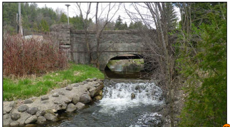
Feature #22: Fieldstone weir (listed, non-designated significant feature). Feature will require modification as a result of proposed channel realignment. Proposed channel realignment will require a "tie-in" location immediately downstream from Feature 17. Full extent of proposed modification to be confirmed during detailed design.
