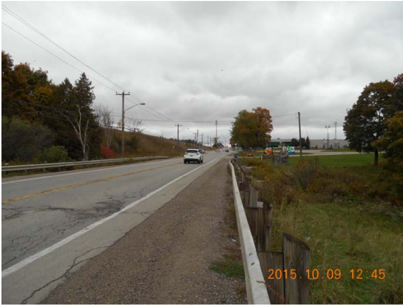
York Road at Clythe Creek crossing
