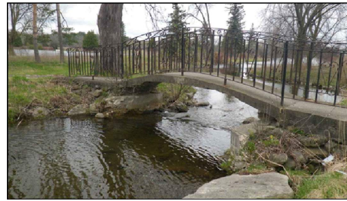
27 Feature #27: Arched concrete and metal pedestrian bridge with stone abutments (potential significance). No impact to feature anticipated.
