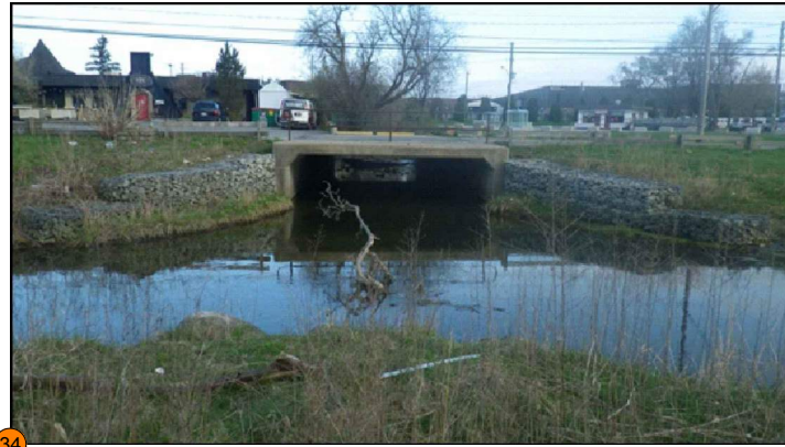
34 Feature #34: Confluence of Clythe Creek and Hadati Creek (potential significance). Potential impact to culvert outlet to accommodate roadway grading requirement and CSP replacement.
