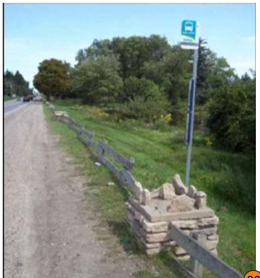
30 Feature #30: Limestone pillars (potential significance). Potential for feature to be modified as a result of roadway grading requirements.
