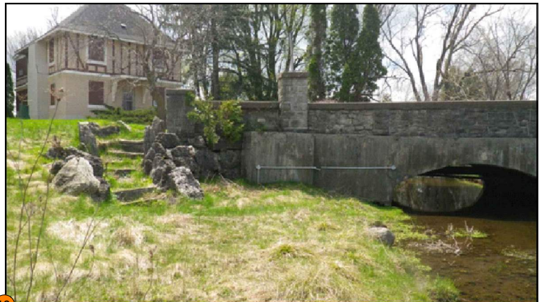
Feature #18: Fieldstone steps to the south of road bridge (listed, non-designated significant feature). Feature is located within the floodplain and will not be impacted by proposed channel works.
