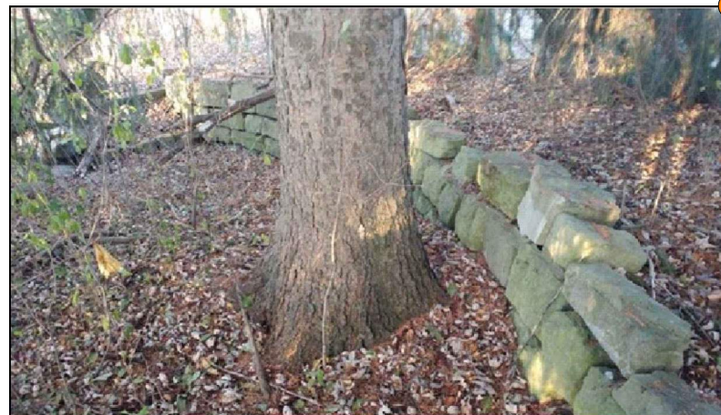
Feature #12: Ashlar limestone wall (listed, non-designated significant feature). Feature is located within the floodplain and will not be impacted by proposed channel works.
