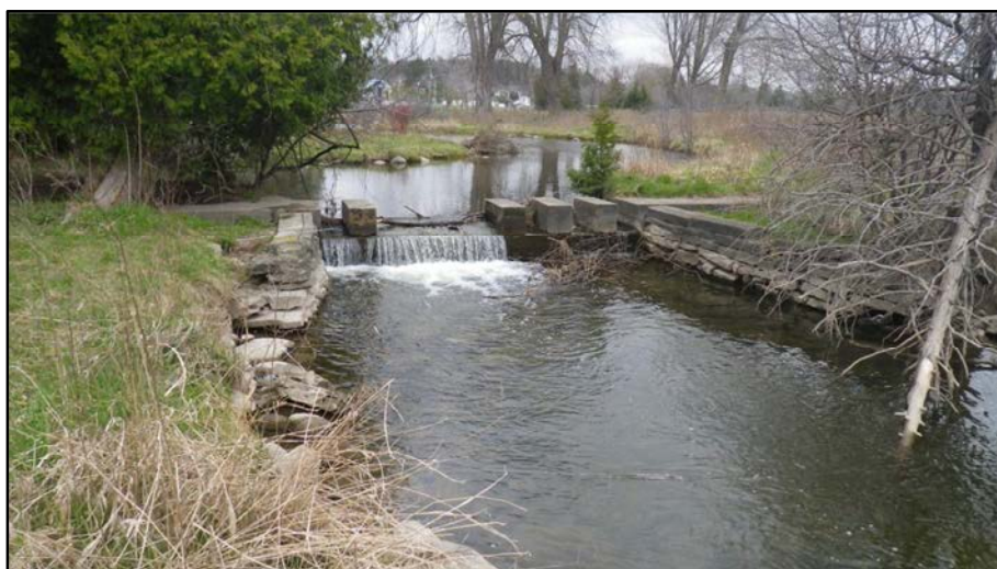
34. Feature #35: Concrete and stone weir (potential significance). Total height of the feature is 0.7 m, with 0.35 m downstream water depth. The structure is 5.5 m wide and is constructed with concrete and decorative limestone blocks along the banks.
