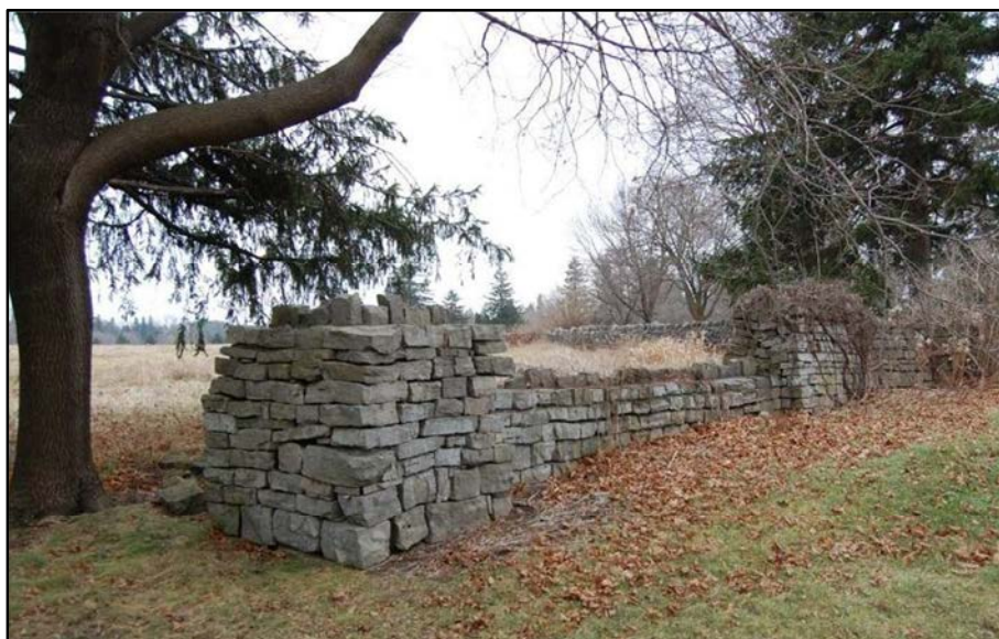
20. Feature #20: Ashlar dry stone wall (listed, non-designated significant feature). The wall is 160 m long and runs parallel to the main entrance driveway south of the creek channel.
