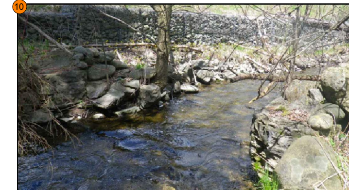
Feature #10: Fieldstone weir (listed, non-designated significant feature). No impact to feature anticipated. Feature is a substantial barrier to fish passage and limiting factor in overall channel function and health. Feature to be taken off-line/disconnected from active flow as a result of channel realignment. Feature will be maintained in landscape but will be impacted by loss of flow.
