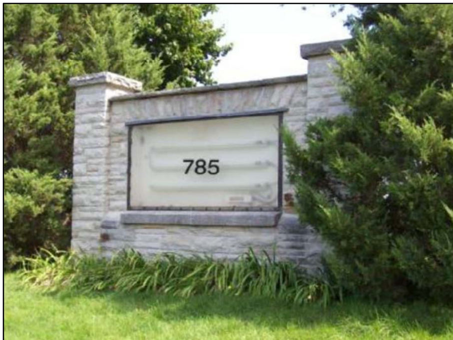
19. Feature #19: Entrance sign, ashlar stone with jack arch (potential significance). The sign is located south of the creek channel and east of the main entrance drive way.
