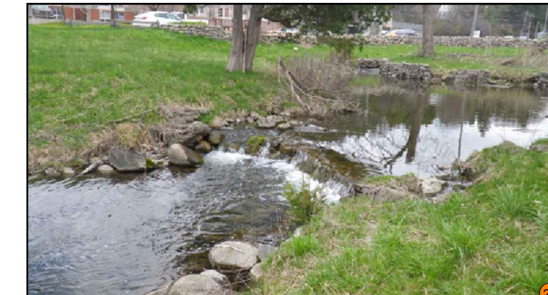
Feature #25: Fieldstone weir (listed, non-designated significant feature). Feature is a substantial barrier to fish passage and limiting factor in overall channel function and health. Feature to be taken off-line and disconnected during low-flow stages as a result of proposed channel realignment. An overflow channel will be incorporated so that the feature will be reconnected during high-flow stages (i.e., flows greater than the 2yr discharge).
