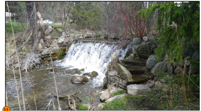
Feature #11: Fieldstone weir with steps and ashlar stone terrace wall (listed, non-designated significant feature). No impact to feature anticipated.
