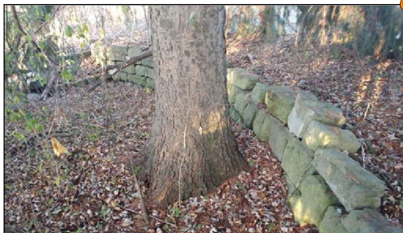
Feature #12: Ashlar limestone wall (listed, non-designated significant feature). No impact to feature anticipated.
