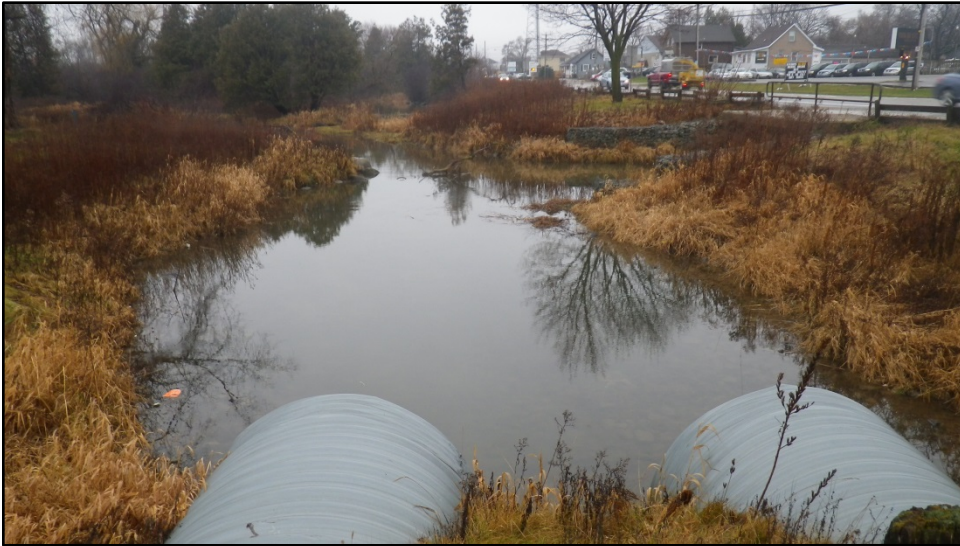
13. Two CSP culverts convey flows downstream from a parklands access road; channel immediately regains width downstream before Hadati Creek Confluence (background, right bank).
