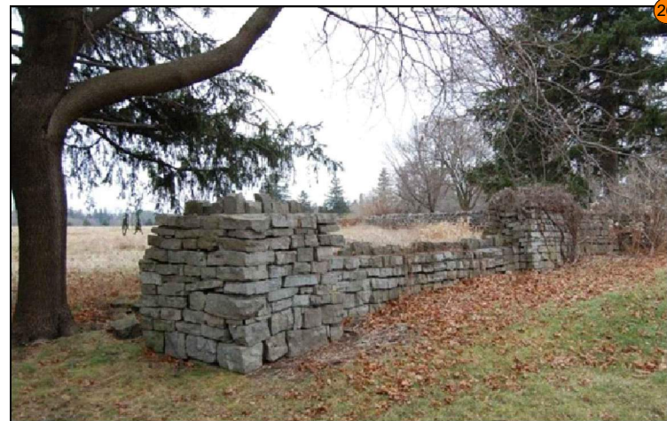
Feature #20: Ashlar dry stone wall (listed, non-designated significant feature). No impact to feature anticipated.
