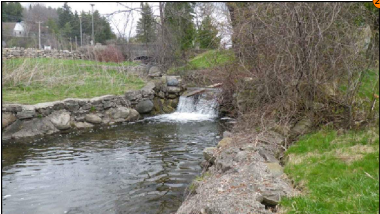
Feature #23: Fieldstone weir (listed, non-designated significant feature). Feature is a substantial barrier to fish passage and limiting factor in overall channel function and health. Feature will require modification or removal (confirmed during detailed design) as a result of channel works.
