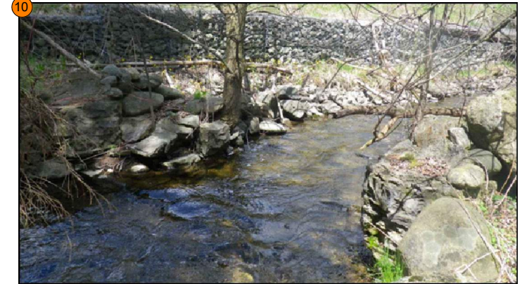
Feature #10: Fieldstone weir (listed, non-designated significant feature). Feature is a substantial barrier to fish passage and limiting factor in overall channel function and health. Feature to be taken off-line and disconnected from active flow as a result of channel realignment. A retaining wall will be installed in order for the feature to be maintained in the landscape.
