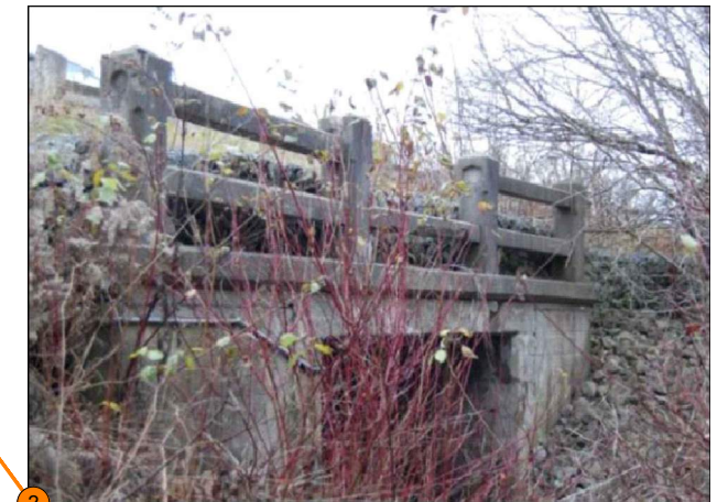
Feature #2: Reinforced concrete road bridge railing (potential significance). No impact to feature anticipated as a result of proposed channel works.
