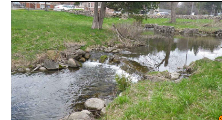
Feature #25: Fieldstone weir (listed, non-designated significant feature). Feature is a substantial barrier to fish passage and limiting factor in overall channel function and health. Feature will require modification or removal (confirmed during detailed design) as a result of channel works.
