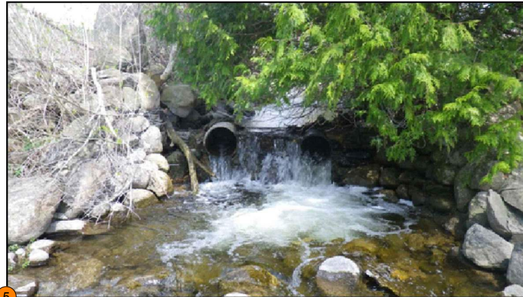
Feature #5: Fieldstone weir with clay pipes (listed, non-designated significant feature). No impact to feature anticipated. Feature is a substantial barrier to fish passage and limiting factor in overall channel function and health. Feature to be taken off-line/disconnected from active flow as a result of channel realignment. Feature will be maintained in landscape but impacted by loss of flow.
