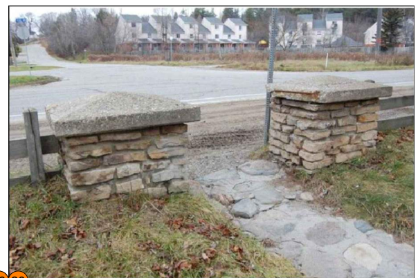
28, 29 Feature #28 and #29: Limestone pillars with wood board fencing leading to main entrance (potential significance). Potential for feature to be modified as a result of roadway grading requirements.
