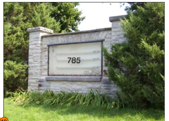
Feature #19: Entrance sign, ashlar stone with jack arch (potential significance). No impact to feature anticipated.
