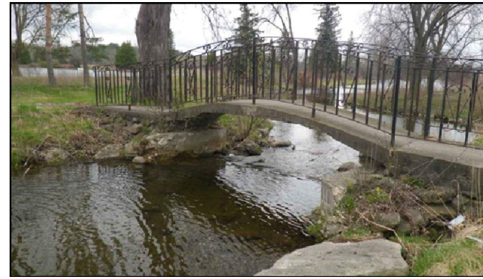
27 Feature #27: Arched concrete and metal pedestrian bridge with stone abutments (potential significance). Potential for feature abutments to be modified as a result of proposed channel works. The proposed channel will require a "tie-in" location in the vicinity of the abutments both upstream and downstream. Full extent of proposed modification to be confirmed during detailed design.
