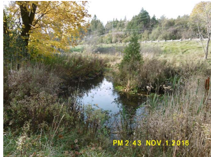
Pool downstream of culvert
