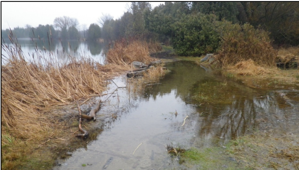
22. South pond breaches its banks at the pond's northeast corner; flow is contributed to a surface drainage tributary that flows adjacent to the pond and into the Eramosa River.
