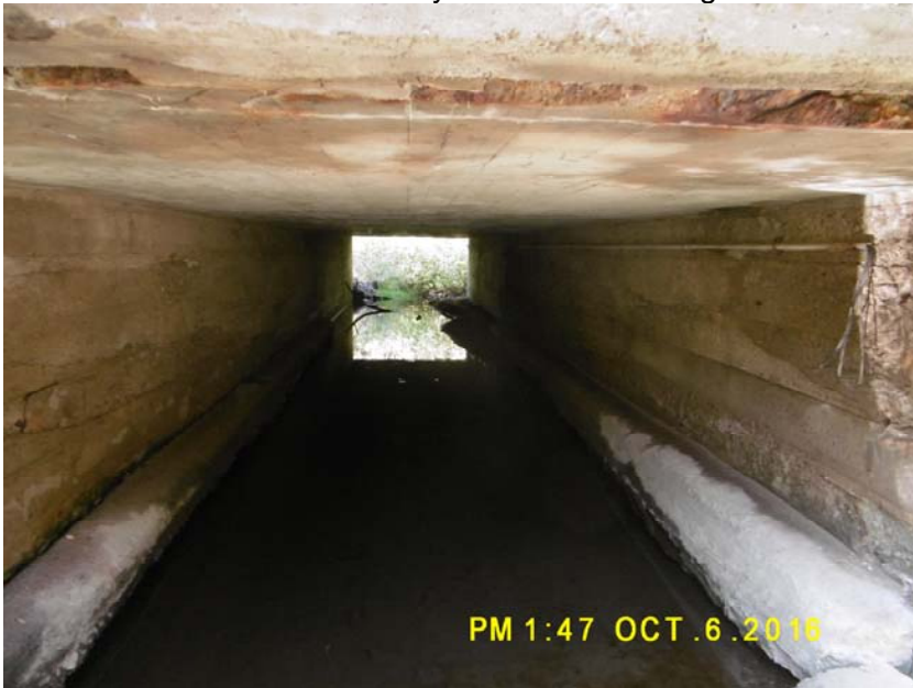
Clythe Creek culvert
