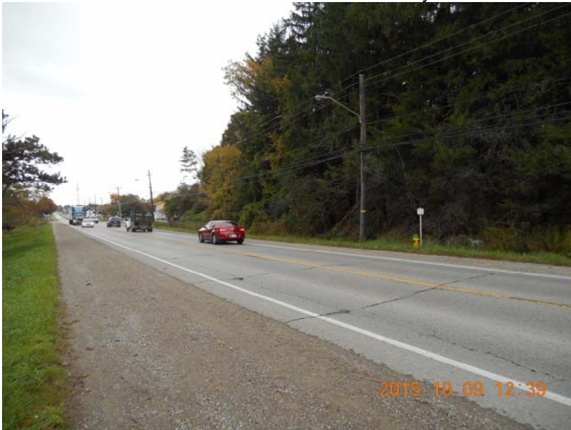
Looking west along York Road
