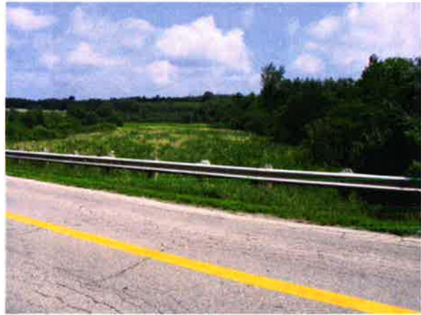
Photo 4: The Creek meanders through a wetland immediately upstream of Watson Road North (Site 4). Hills to the north of the Creek have been cleared for development (construction in progress) and storm water ponds have been constructed.
