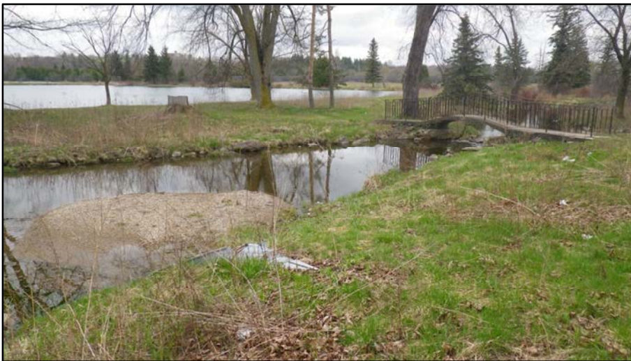
12. Reach C-9B: CSP outlet and sediment deposition plume upstream from pedestrian bridge.
