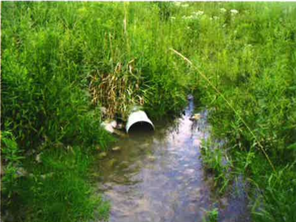
Photo 9: Discharge from the storm water pond was consistently turbid throughout the summer. Water quality in Clyde Creek was noticeably impacted and sedimentation of the Creek channel downstream of the pond outlet was observed.
