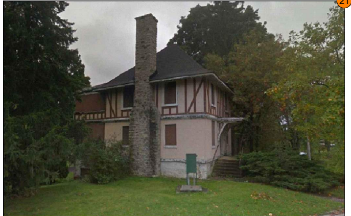
Feature #21: Willowbank Hall (listed, non-designated significant feature). No impact to feature anticipated.
