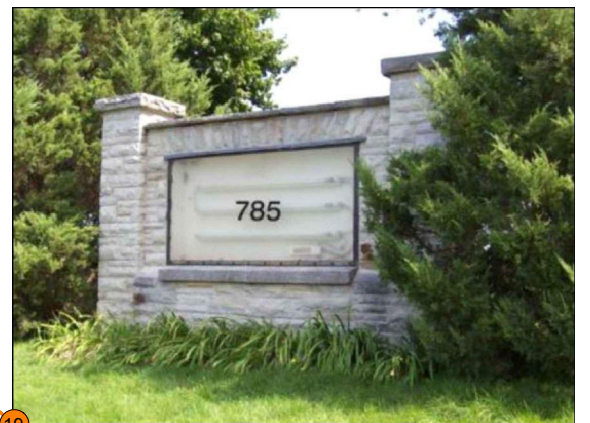
Feature #19: Entrance sign, ashlar stone with jack arch (potential significance). Feature is located within the floodplain and will not be impacted by proposed channel works.
