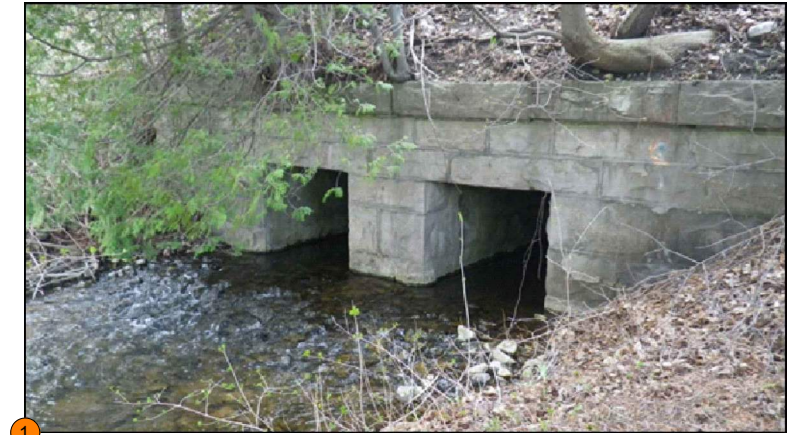
Feature #1: Ashlar stone culvert (potential significance). Channel works are not proposed upstream from York Road therefore the feature will not be impacted by proposed channel works.
