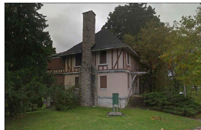
Feature #21: Willowbank Hall (listed, non-designated significant feature). No impact to feature anticipated.
