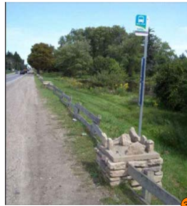
30 Feature #30: Limestone pillars (potential significance). Potential for feature to be modified as a result of roadway grading requirements.
