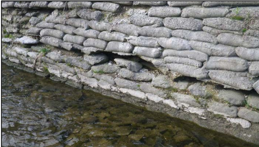
23. Reach HC-1: Concrete cushion bank protection installed along the west bank is failing.
