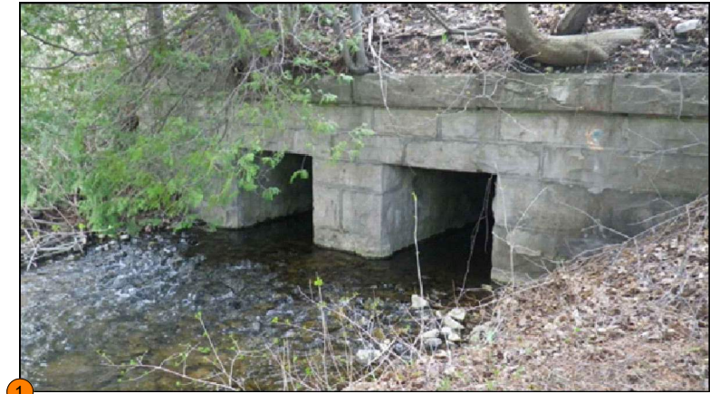
Feature #1: Ashlar stone culvert (potential significance). No impact to feature anticipated.
