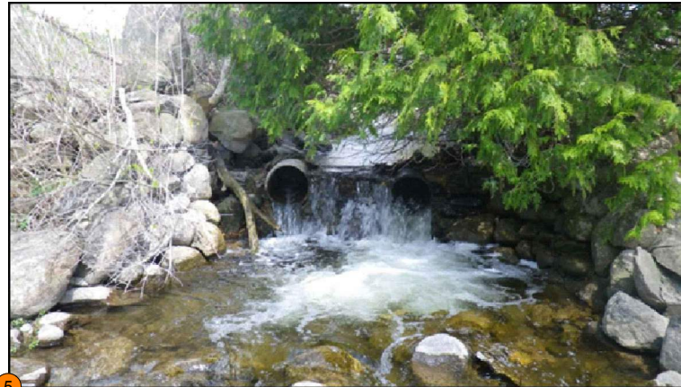
Feature #5: Fieldstone weir with clay pipes (listed, non-designated significant feature). Feature is a substantial barrier to fish passage and limiting factor in overall channel function and health. Feature to be taken off-line and disconnected from active flow as a result of channel realignment. Feature will be maintained in the landscape.
