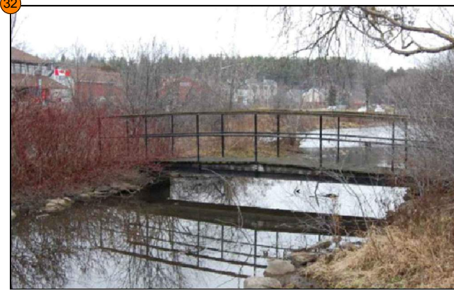
32 Feature #32: Metal and wood pedestrian bridge (potential significance). No impact to feature anticipated.
