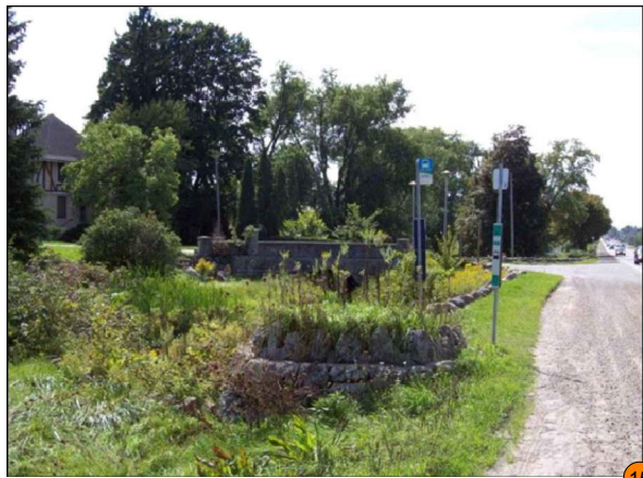
Feature #15: Fieldstone east entrance wall with sentinel stones (listed, non-designated significant feature). No impact to feature anticipated as a result of proposed channel works.
