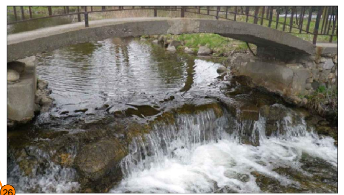
26 Feature #26: Fieldstone weir (listed, non-designated significant feature). Feature is a substantial barrier to fish passage and limiting factor in overall channel function and health. Feature will require modification or removal (confirmed during detailed design) as a result of channel works.
