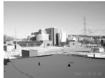
In 1993 a cogeneration and energy facility was constructed. The purpose was to use the digester gas produced in the digesters to heat the buildings and the digesters. The digester gas was also used to produce electricity to help reduce the electrical demand of the plant. Two 240 kW cogeneration units were installed along with two boilers, and a gas room
