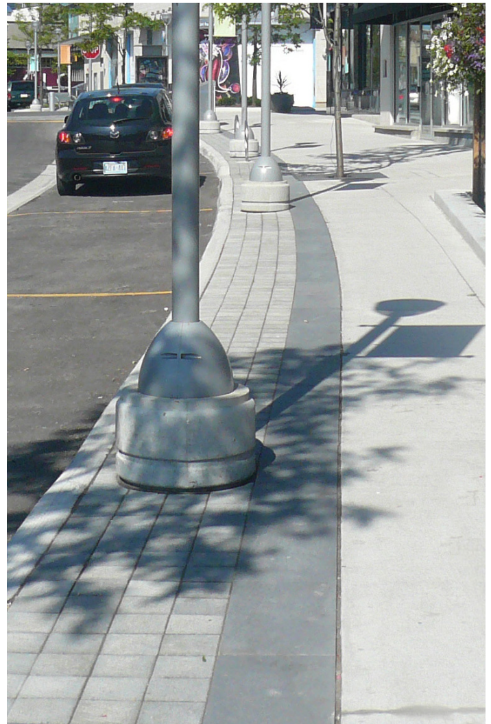
Edge zones provide a safety buffer against car doors and mirrors and accommodate road signage.
