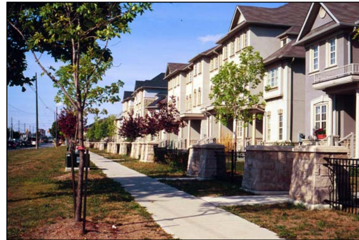
This townhouse complex on Yonge Street in Richmond Hill demonstrates a good street edge with direct a decorative fence treatment. The 3-st height offers a good scale for a medium density development along a wide road cross-section.
