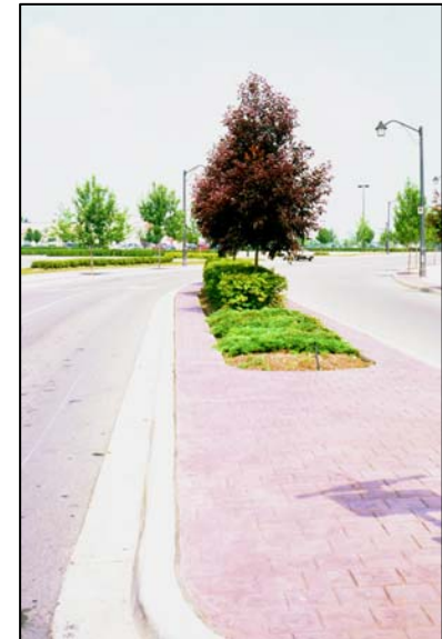
This planted and decoratively paved median at the entrance of a retail plaza in Burlington at Appleby Line & Upper Middle demonstrates a visually pleasing treatment, which also provides a pedestrian refuge.
