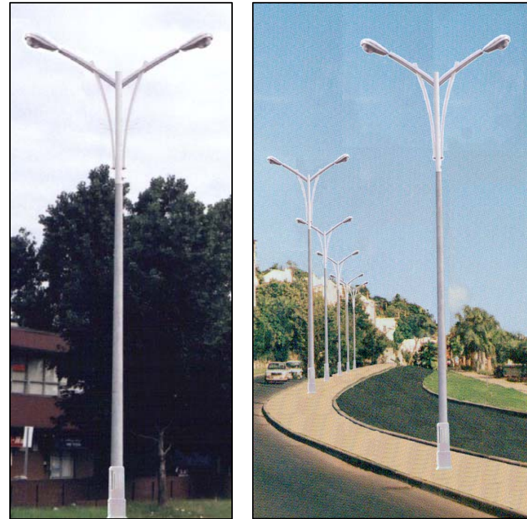
The examples above indicate the recommended design approach to median roadway lighting on Gordon Street, north of Clair Road
