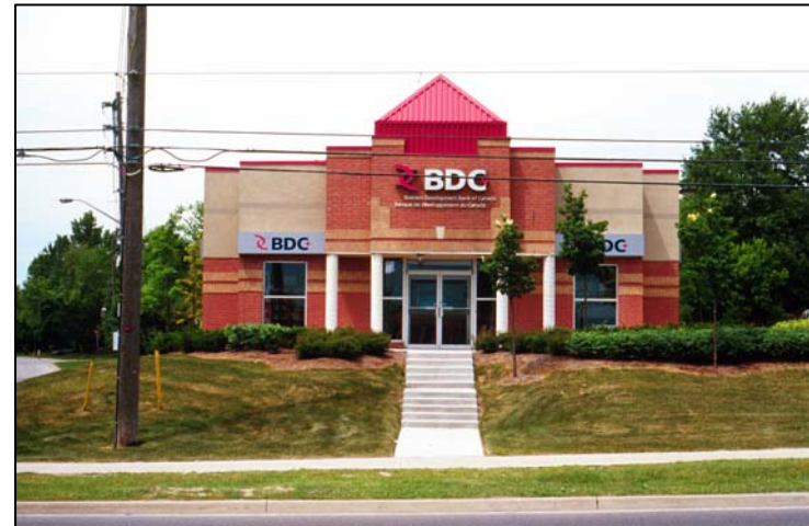
Wherever possible, it is preferred to place buildings in close proximity to the street to support pedestrian activity and provide visual interest, as this bank building in a retail plaza in Markham at Highway 7 near Woodbine demonstrates. Also note the roof top treatment, which blends well with the rest of the building
