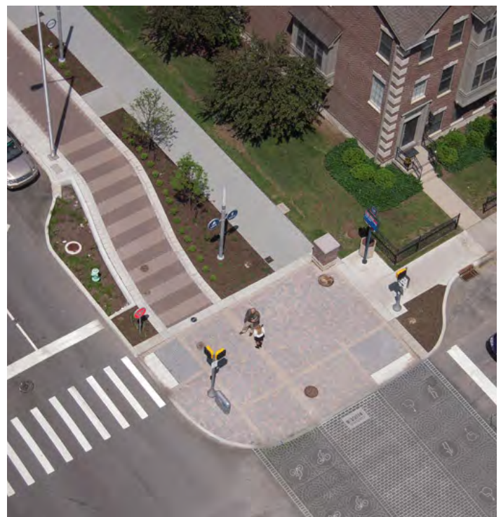
Curb extensions should be considered in intersection design to reduce crossing distance.
