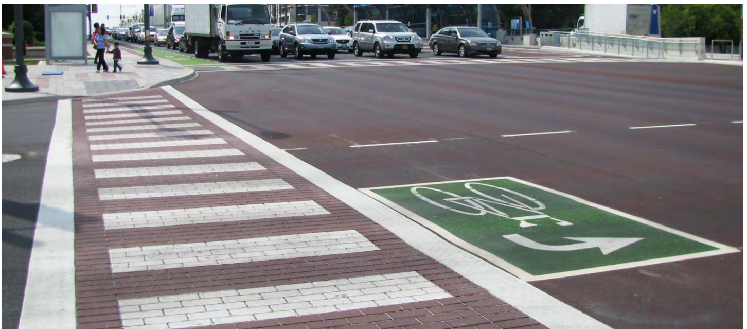
Zebra markings at crosswalk enhance visibility.
