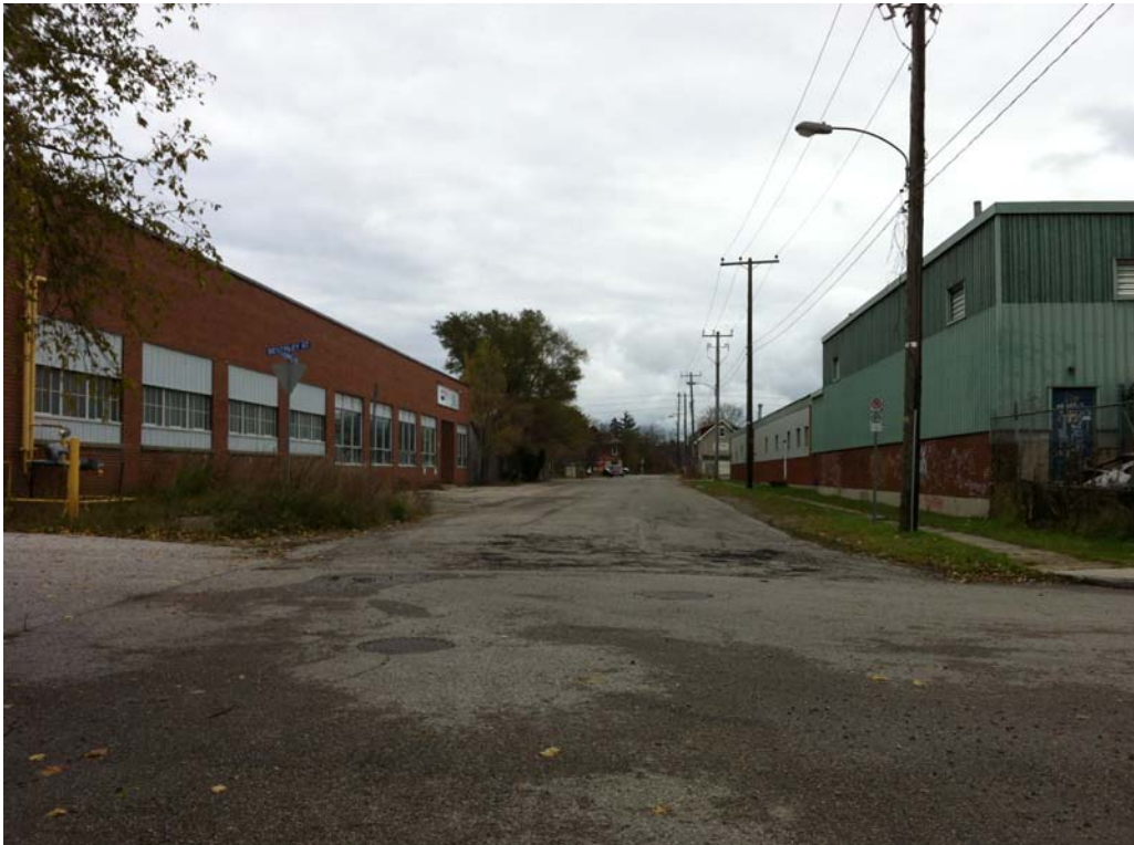
Photograph No. 10: View of adjacent properties (Kingsmill Avenue) to the east
