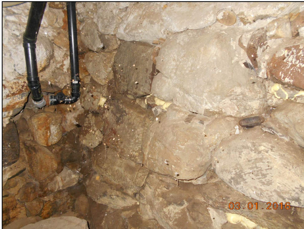
Photograph 7: View of the stone foundation and sewer pipes exiting to the south, looking south.
