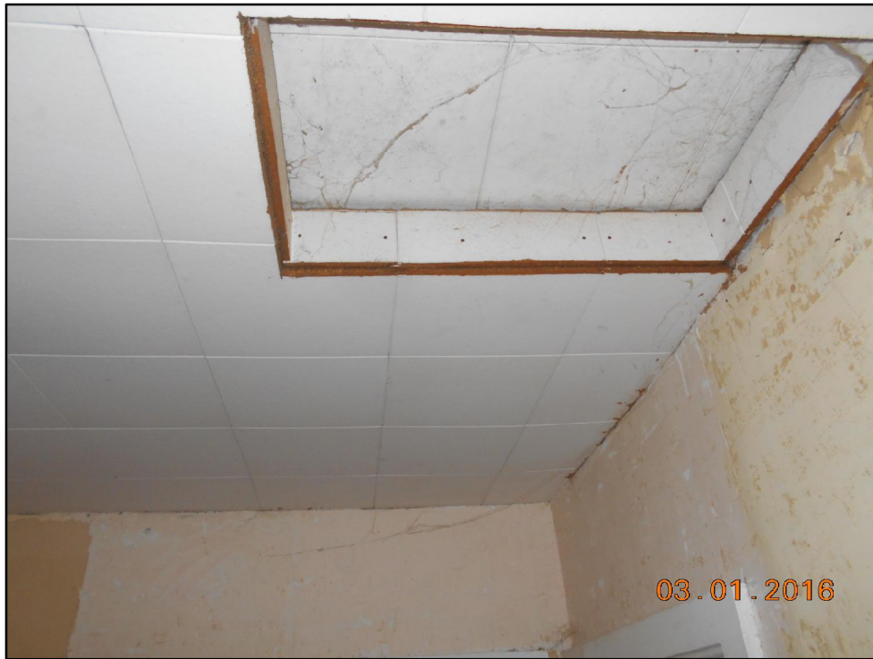
Photograph 9: View of potential ACM ceiling tiles on second floor ceiling.
