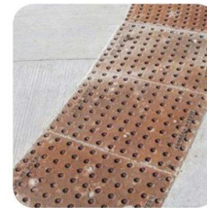
Detectable Warning Surface
