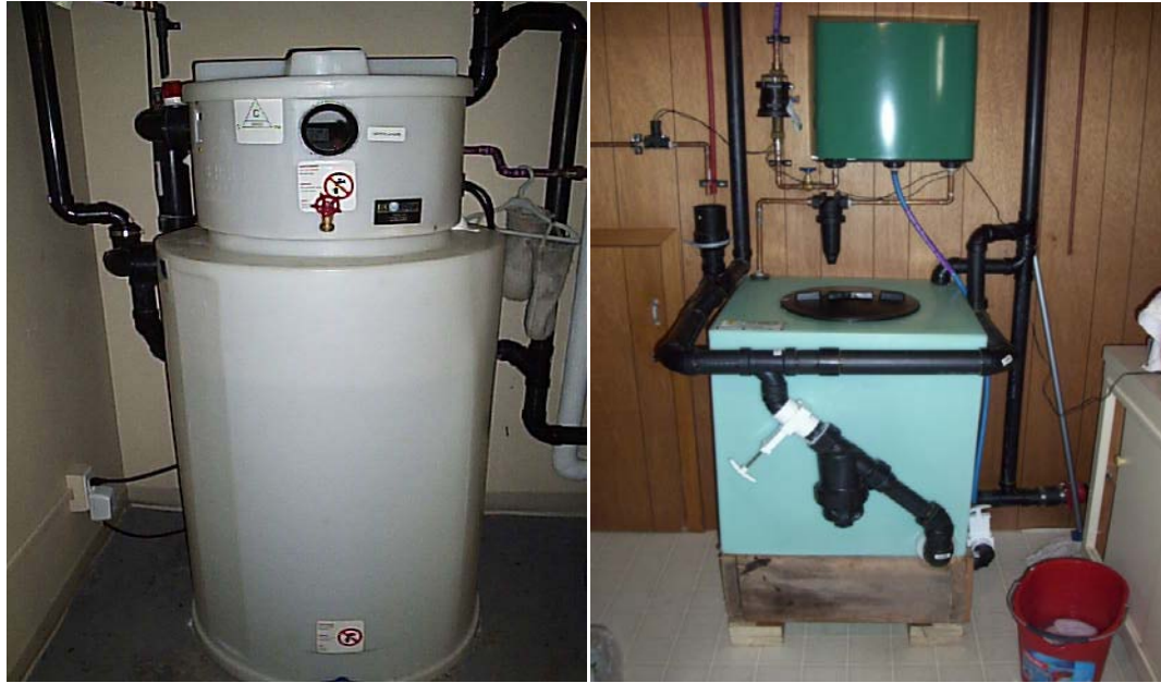
Figure 1: Brac Greywater Reuse System (left) and IDus Controls' ConservePump Greywater Reuse System (right)
