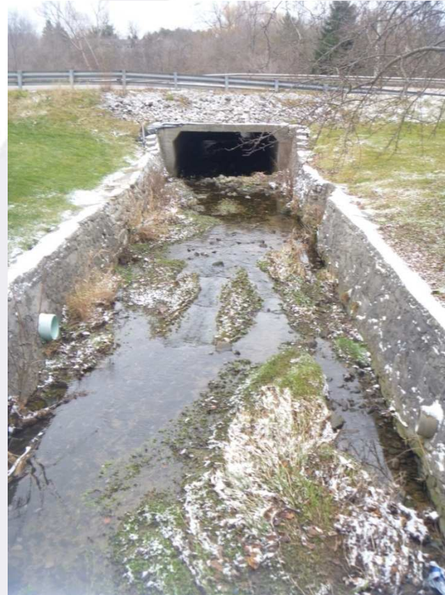
Photo 20: Downstream from the proposed crossing location (December 2012).
