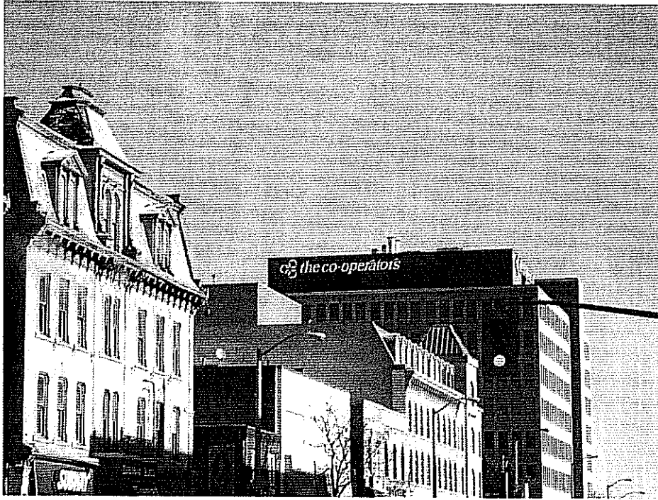
CO-OPERATORS- 128-130 MACDONELL STREET
