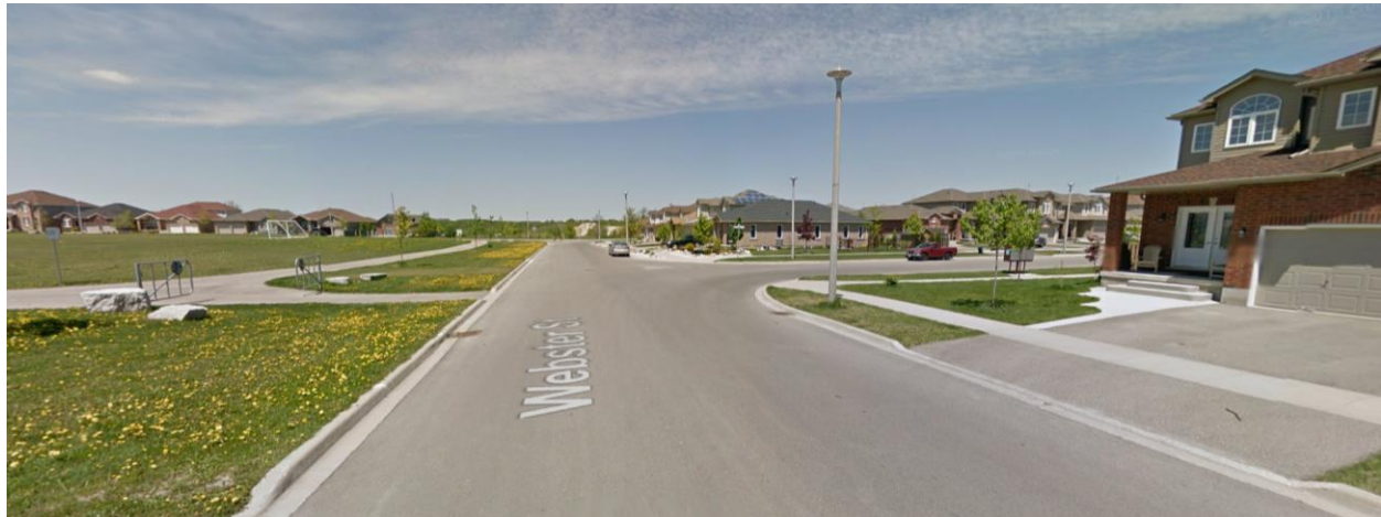
Figure 36. Example of Road Segment in Very Good Category (PCI \geq 80 )
