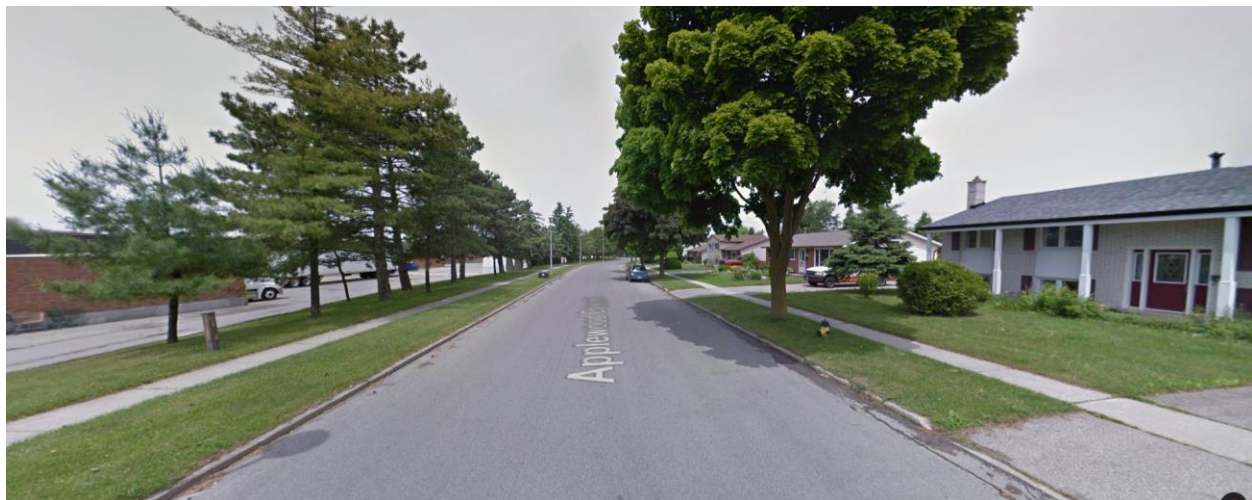
Figure 37. Example of Road Segment in Good Category (PCI 60 to 79)
