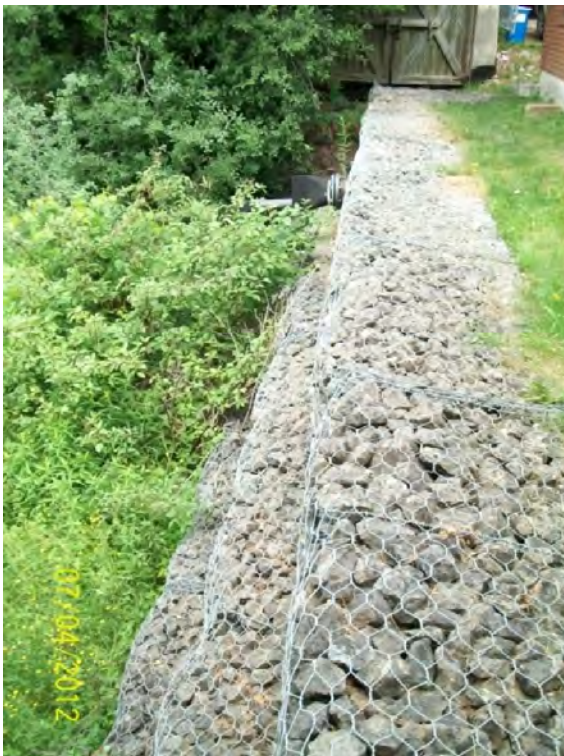
Photos 2 and 3. Gabion wall along north side of facility adjacent to Clythe Creek floodplain. Localized minor settlement but overall in good condition.
