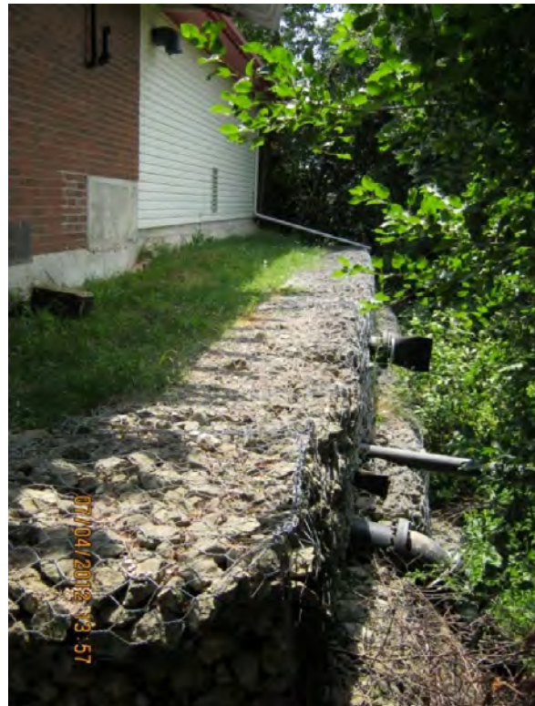
Photos 2 and 3. Gabion wall along north side of facility adjacent to Clythe Creek floodplain. Localized minor settlement but overall in good condition.
