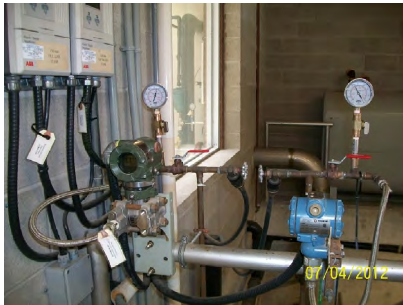
Photo 25. Station inlet and discharge pressure transmitters
