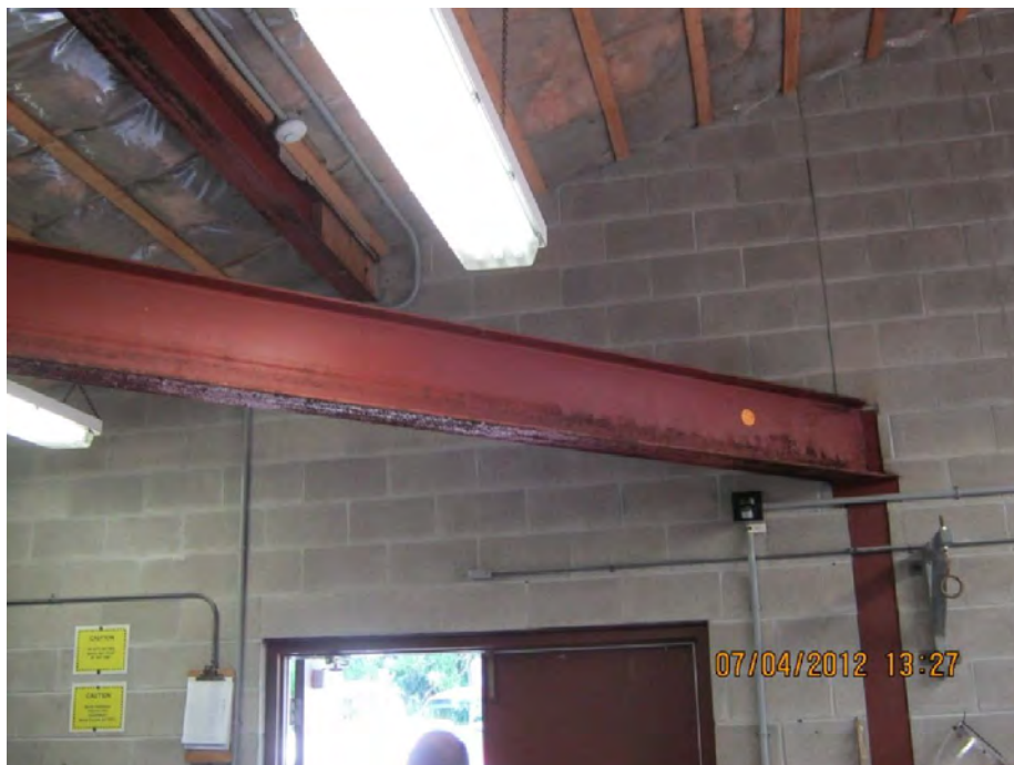
Photo 5. Interior of well house, ceiling and I-beam
