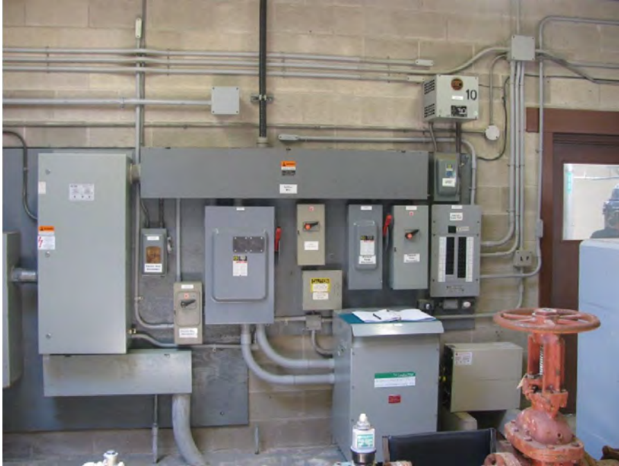
Photo 27. Existing electrical distribution to be replaced with MCC which is to include new power meter, feeder breakers, main breaker, well pump soft starter, and new ATS.
