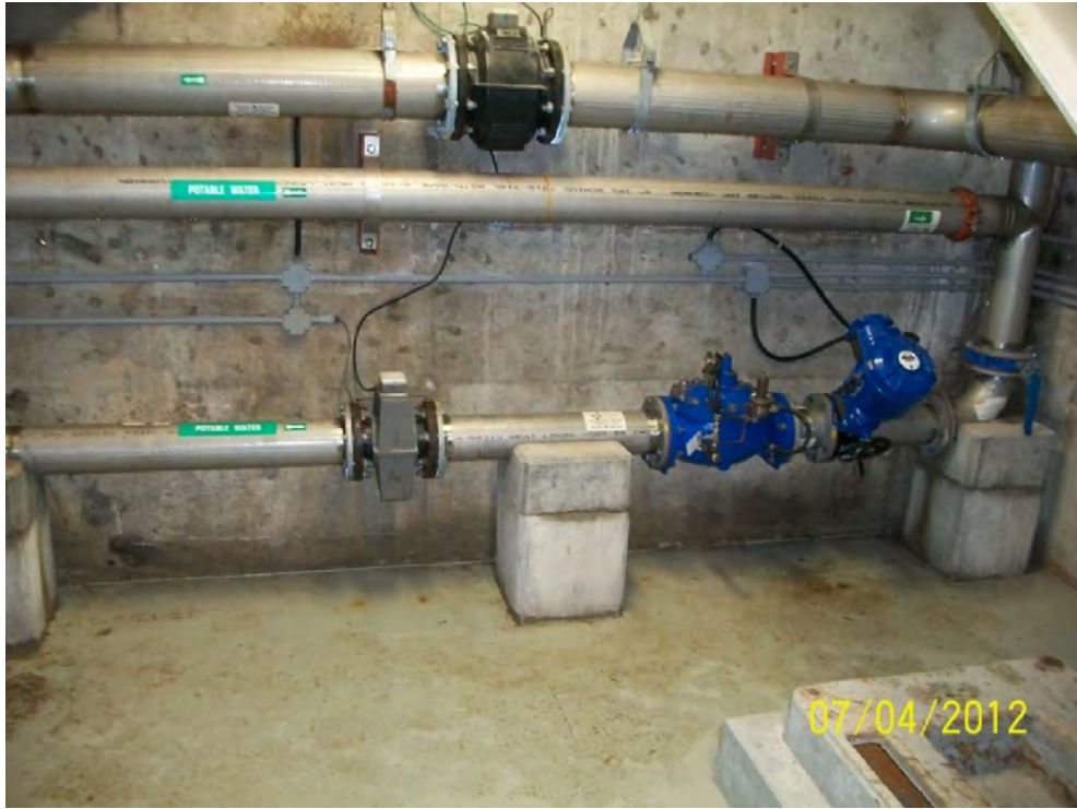
Photo 19. Stainless steel process piping, instrumentation (mag meters) and actuated butterfly valve in lower level valve room
