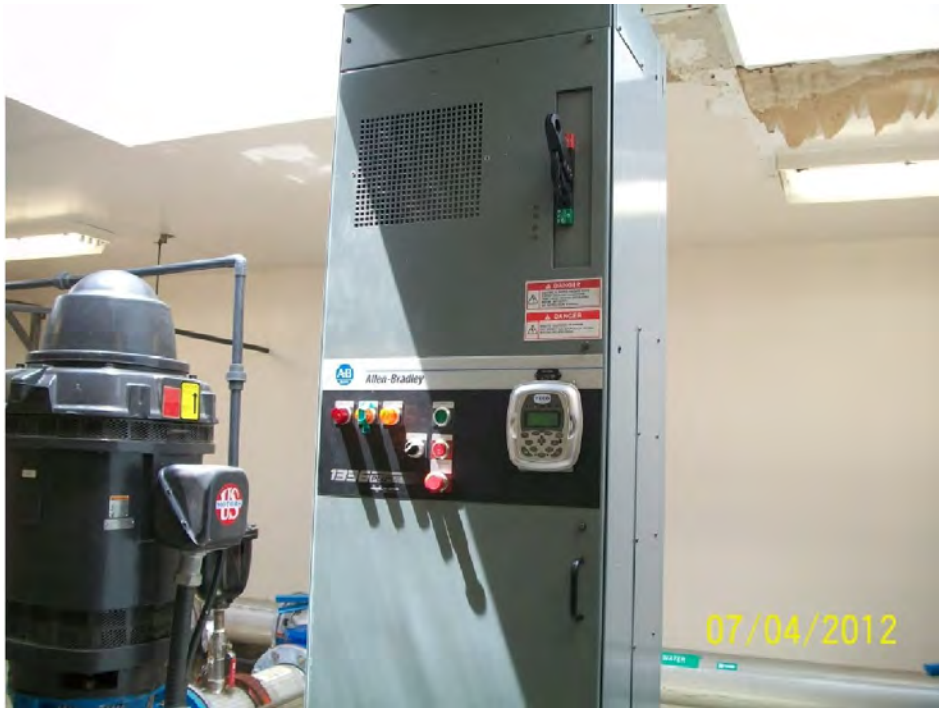
Photo 6. Pump Room showing water damage at skylight above Booster Pump 2
