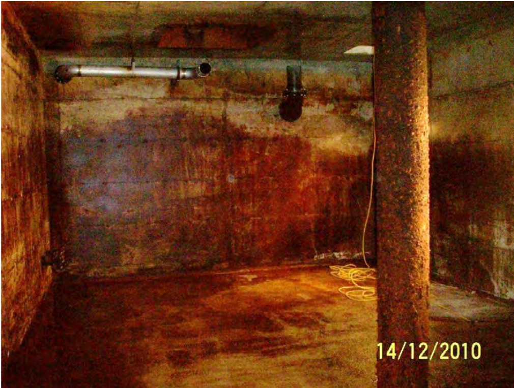
Photo 12. Inside of reservoir showing well casing, Zone 1 inlet piping, and overflow pipe.
