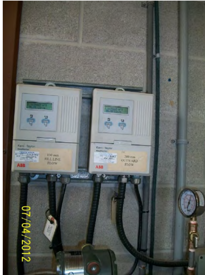
Photo 24. Indicators/transmitters for the inlet and discharge magnetic flow meters
