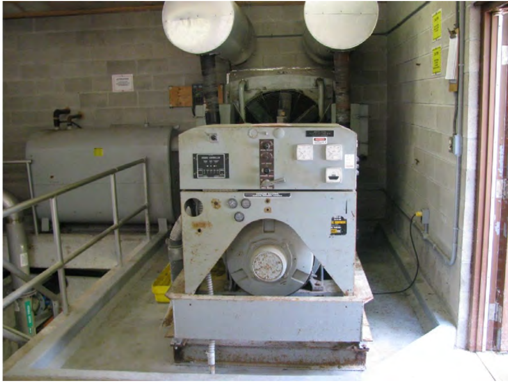
Photo 22. Existing standby generator with secondary containment.
