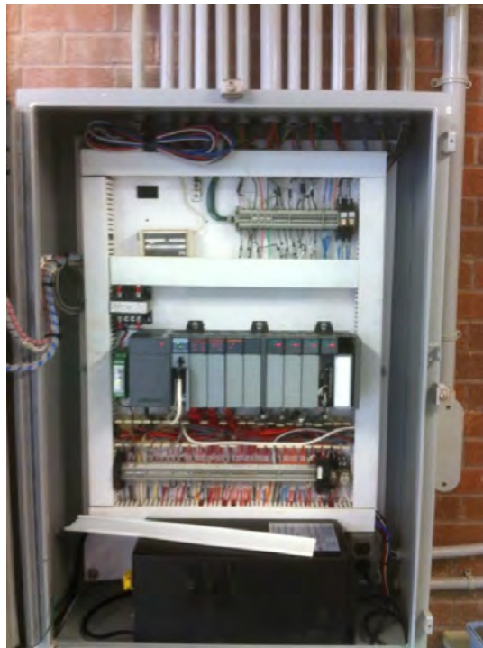
Photo 28. Existing PLC panel is recommended for replacement based on I/O capacity.
