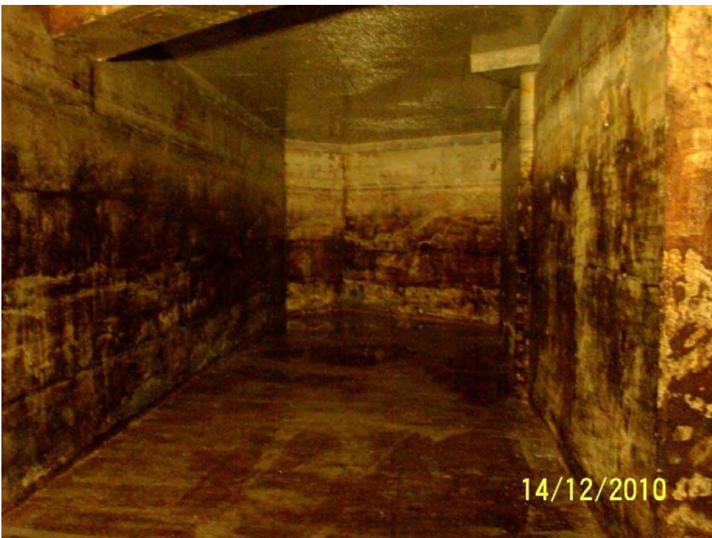
Photo 13. Inside of reservoir at western corner.
