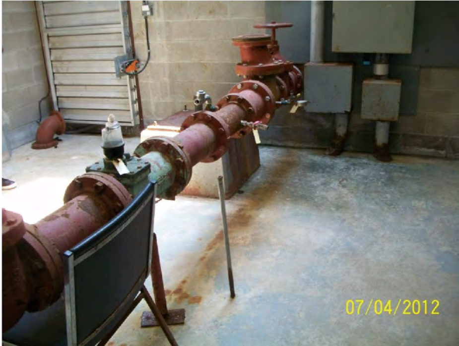
Photo 17. Existing ductile iron piping and wellhead pedestal in the well house
