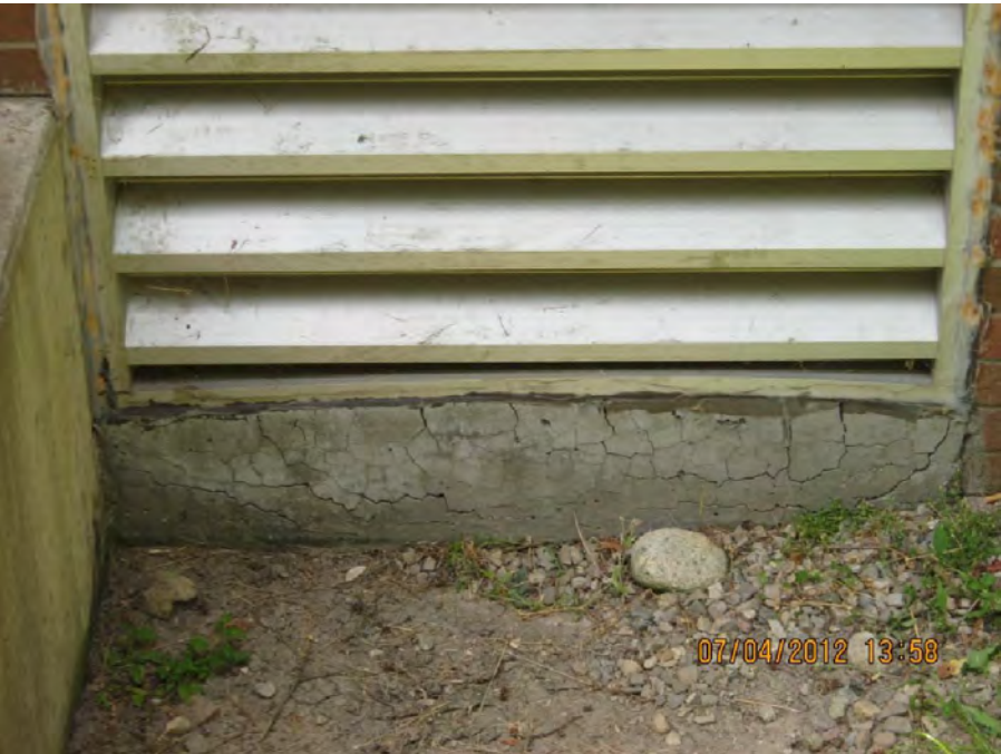
Photo 11. Exterior : Concrete deterioration beneath intake louver on south wall of well house.
