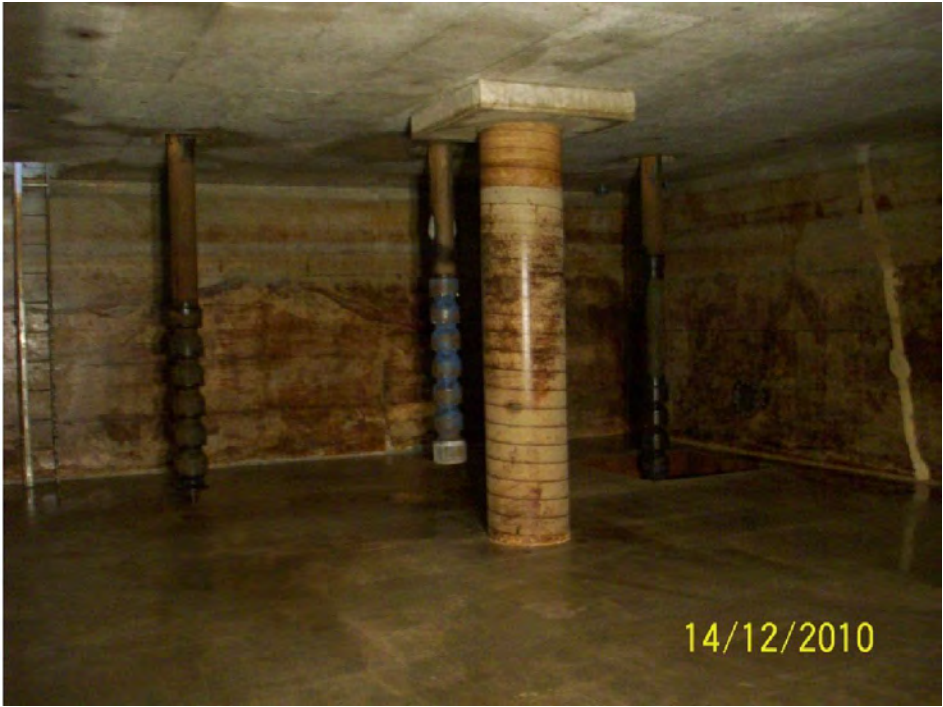
Photo 15. Inside of reservoir showing all 3 Booster Pumps and sump at Booster Pump 3.
