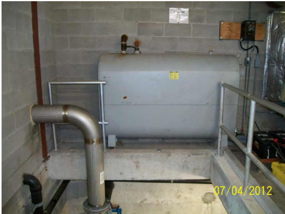
Photo 23. Diesel fuel tank for generator with secondary containment
