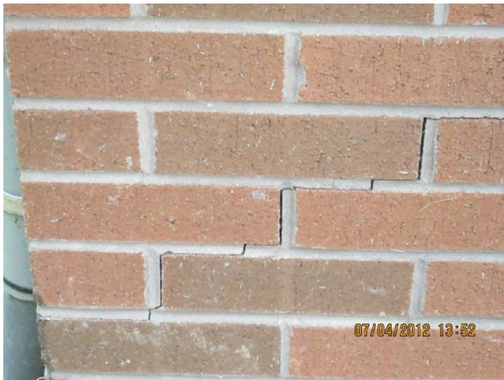
Photo 9. Close up view of exterior of east wall at south end – mortar crack in brick work
