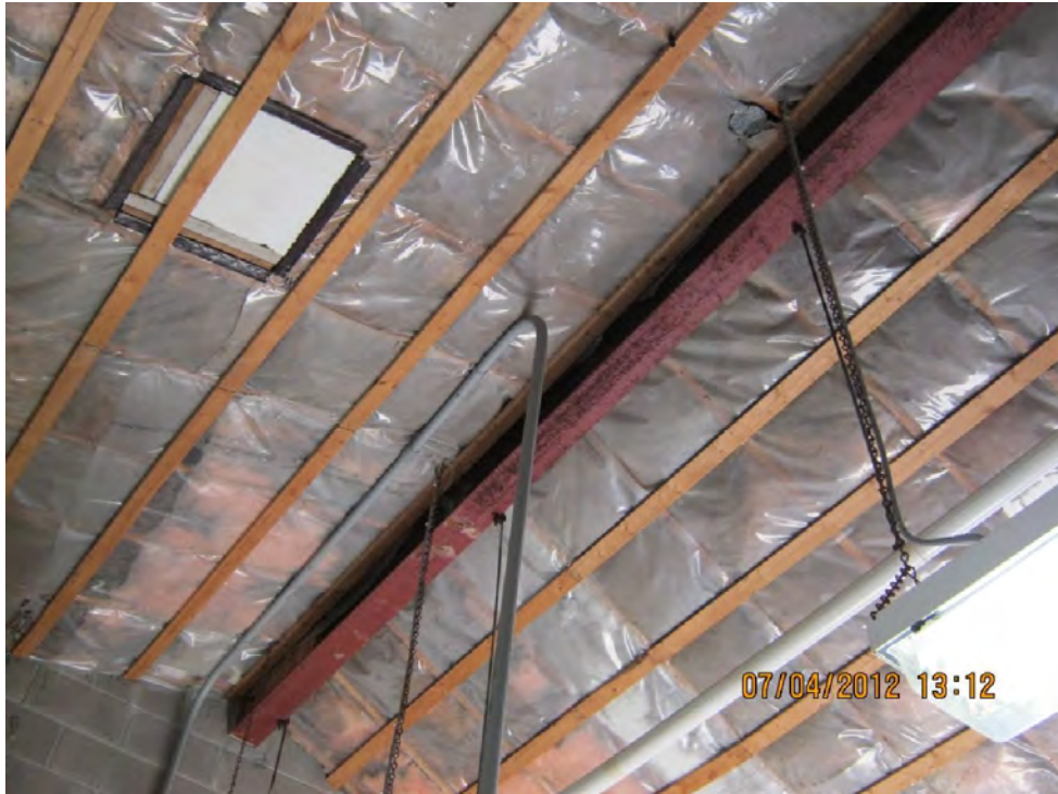
Photo 4. View of ceiling in well house
