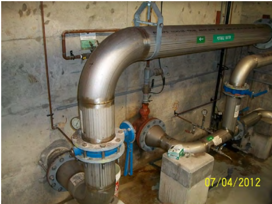
Photo 18. Stainless steel process piping entering and leaving the station at the east wall of the lower level valve room
