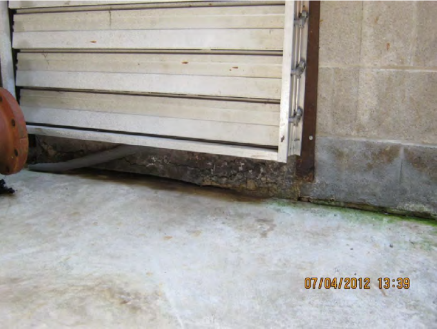
Photo 10. Interior : Concrete deterioration beneath intake louver on south wall of well house.
