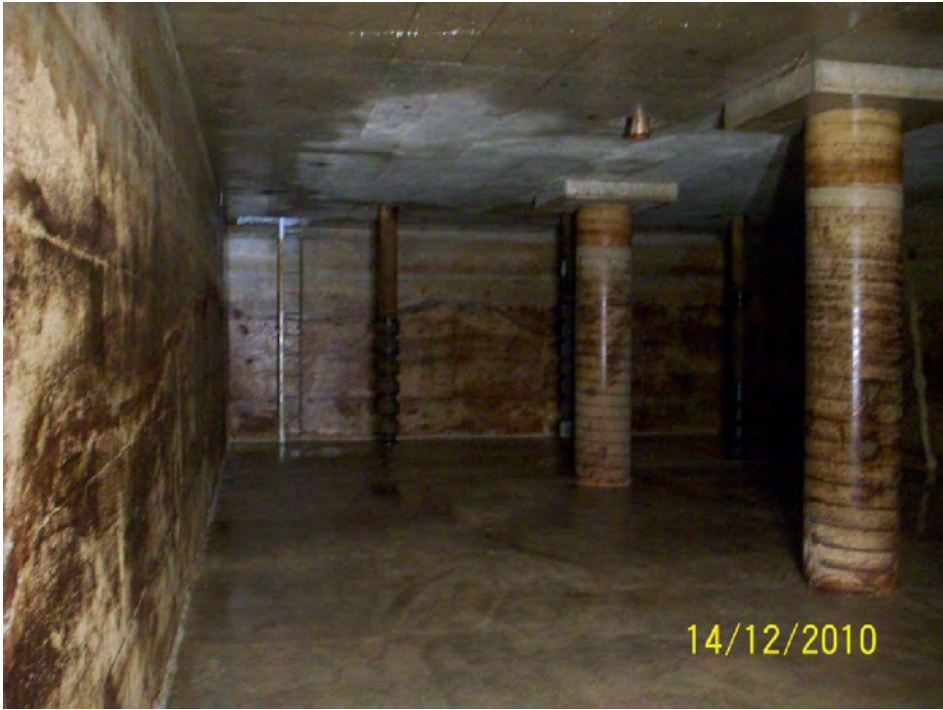
Photo 14. Inside of reservoir showing columns and Booster Pumps 1 and 2.
