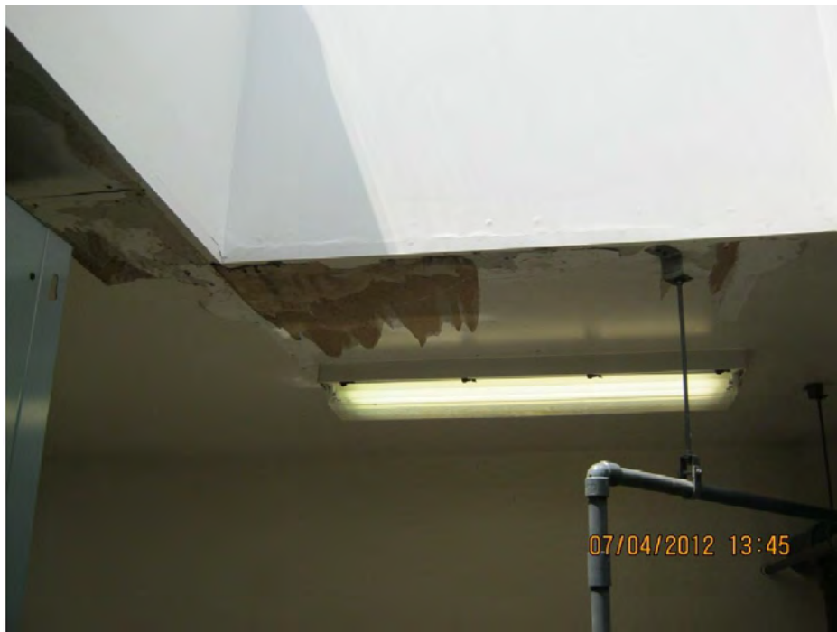
Photo 7. Pump Room showing close up view of water damage at skylight above Booster Pump 2
