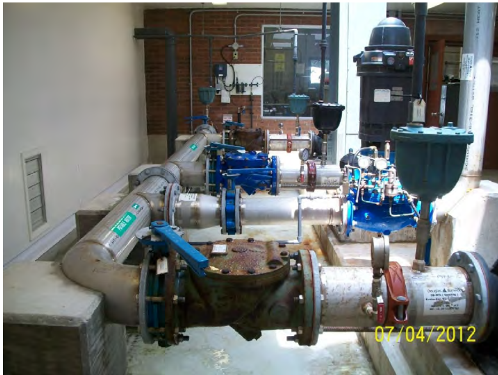
Photo 20. Booster pumps, discharge piping, and valve arrangement
