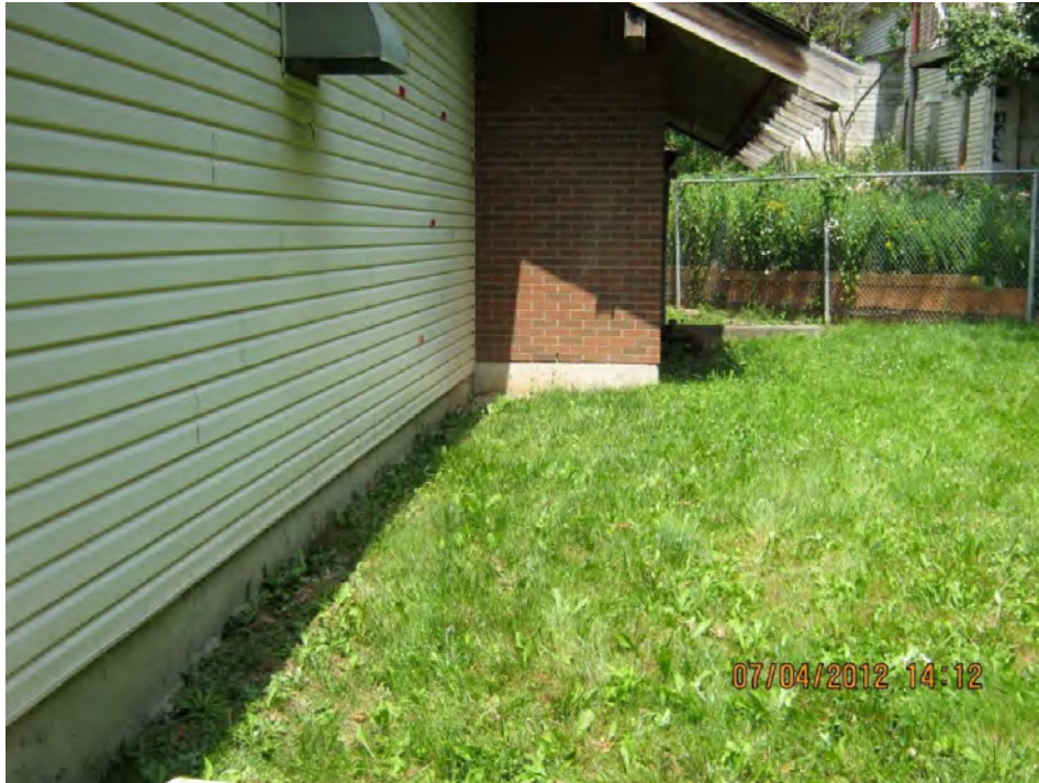
Photo 1. Site grading along south side of building directed towards building. Note lack of eave troughs and down spouts
