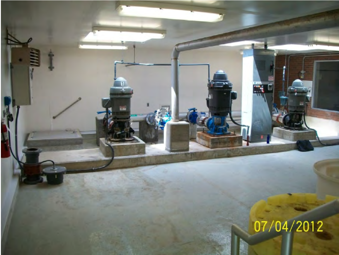
Photo 21. Pump room constructed in 1998 showing 3 vertical turbine booster pumps
