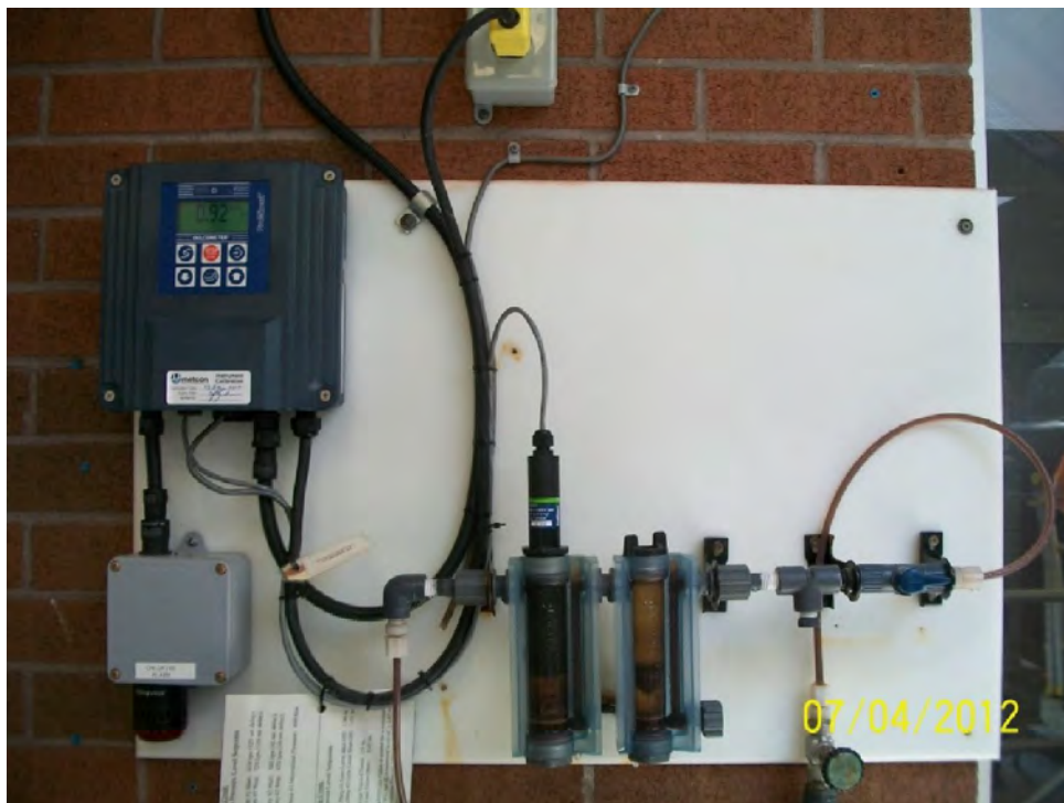
Photo 26. Chlorine residual analyzer with probe holders
