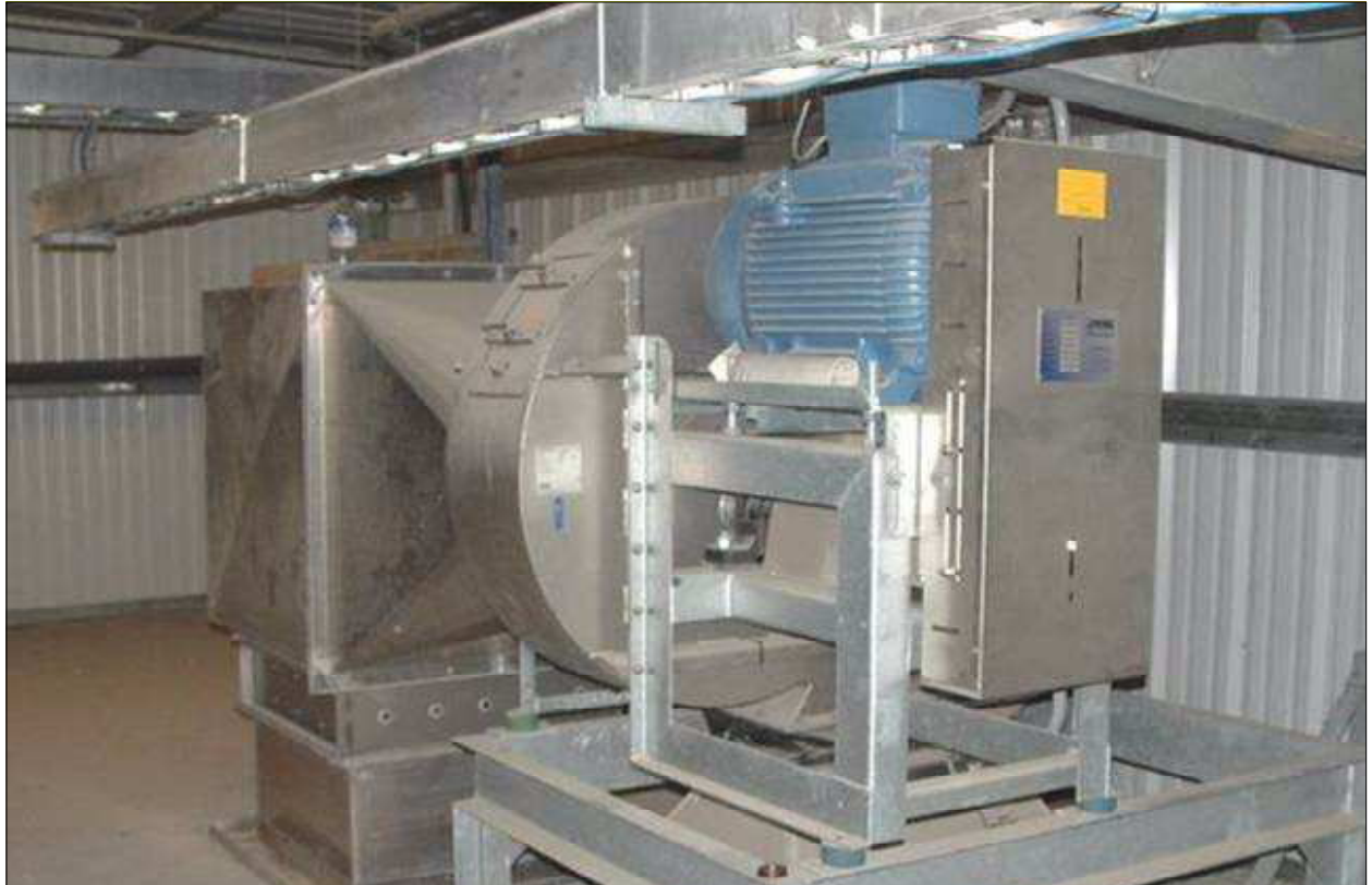
Air Handling System
