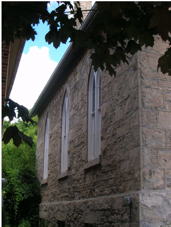
Figure 8. North Elevation Featuring Symmetrically-placed Windows
