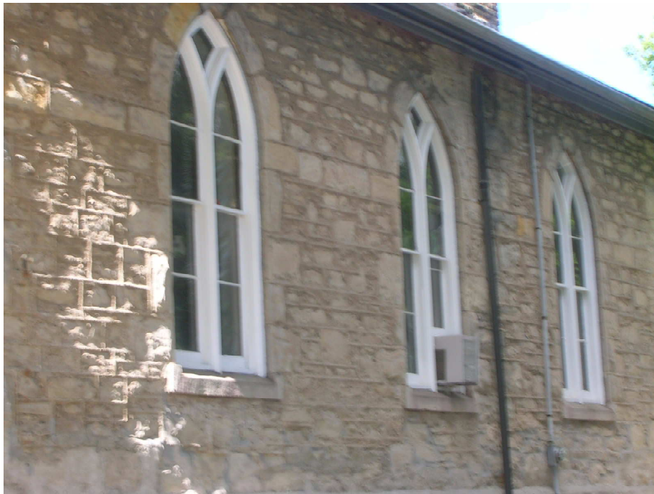
Figure 7. South Elevation Featuring Lancet Windows
