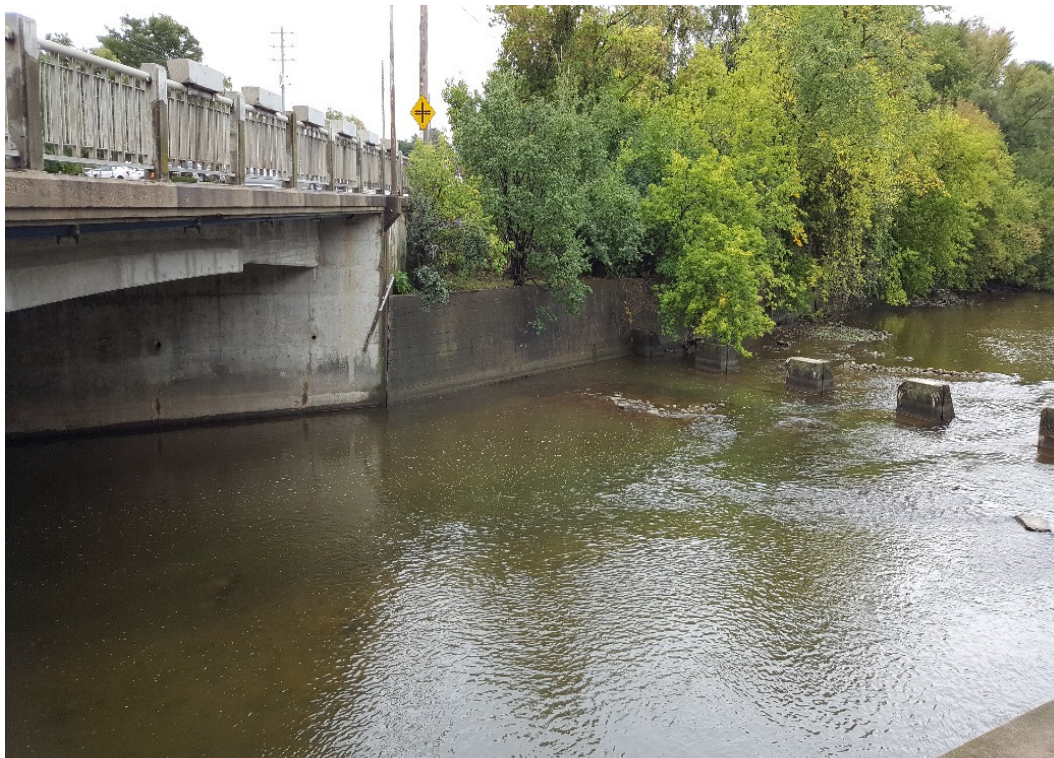
Figure 2: Retaining Wall (South End)
