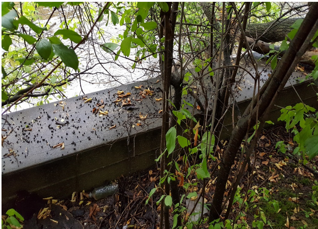
Figure 3: Top of the Retaining Wall (South End)
