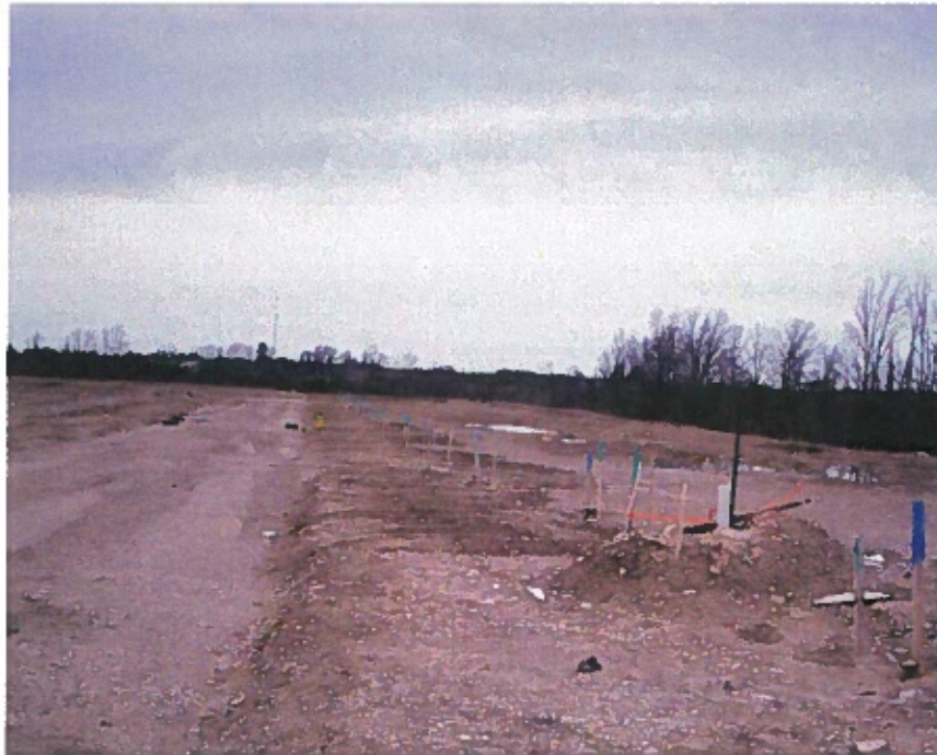
Photo 9: View of Mussen Street under construction looking north. Markers for the watermain, water service lines, sanitary sewer lines and storm sewers within the site can be seen.
