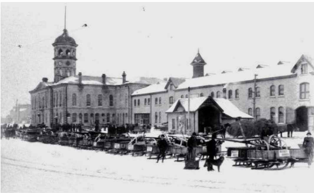
Guelph City Hall and Winter Fair Building, c. 1910.
