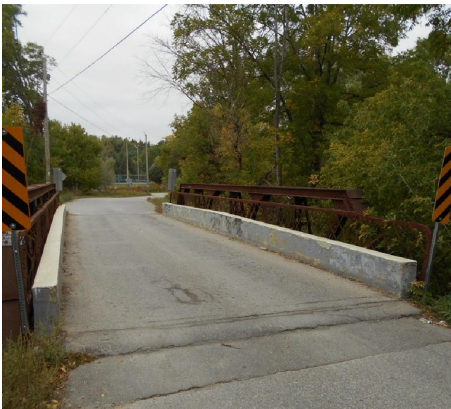
Figure 7: Similar truss bridge with FRP deck, where the steel trusses carry only their own weight
