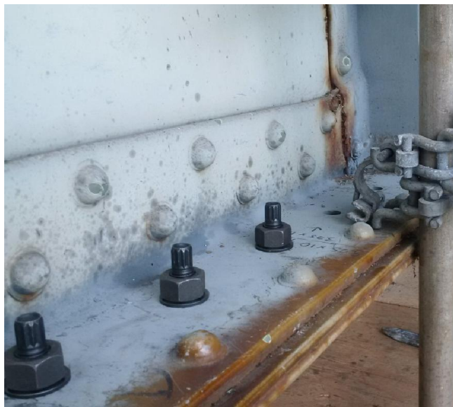
Figure 6: As viewed from the opposite side, these bolts resemble a typical threaded bolt and nut assembly
