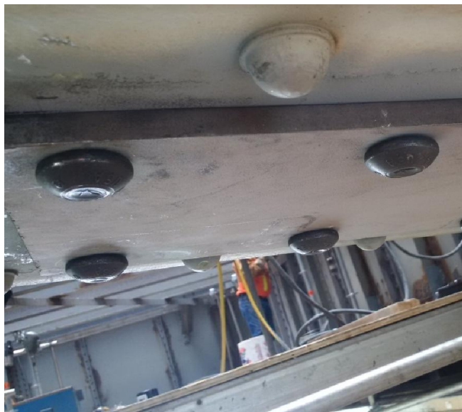
Figure 5: As viewed from the surface, bolts used adjacent to existing rivets to mimic the appearance of rivets
