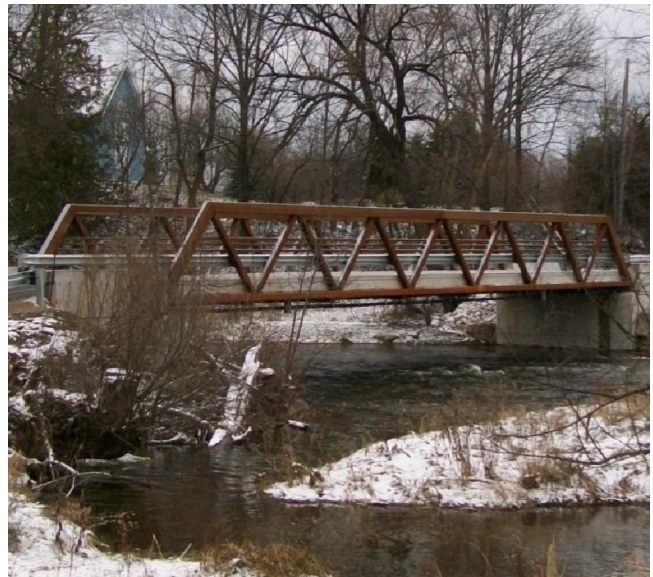
Figure 10: New steel truss bridge constructed with welded connections
