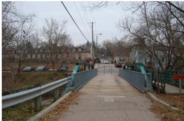
Plate 4: North view of existing bridges; Area is disturbed, no potential
