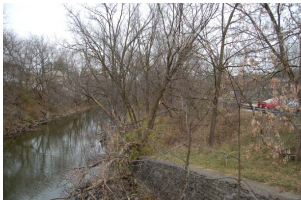
Plate 6: Northwest view of Study Area; Existing bridge footing is disturbed, areas beyond are sloped, no potential
