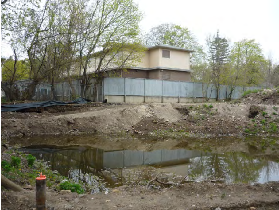
Photograph C-3: View of excavation, looking south
