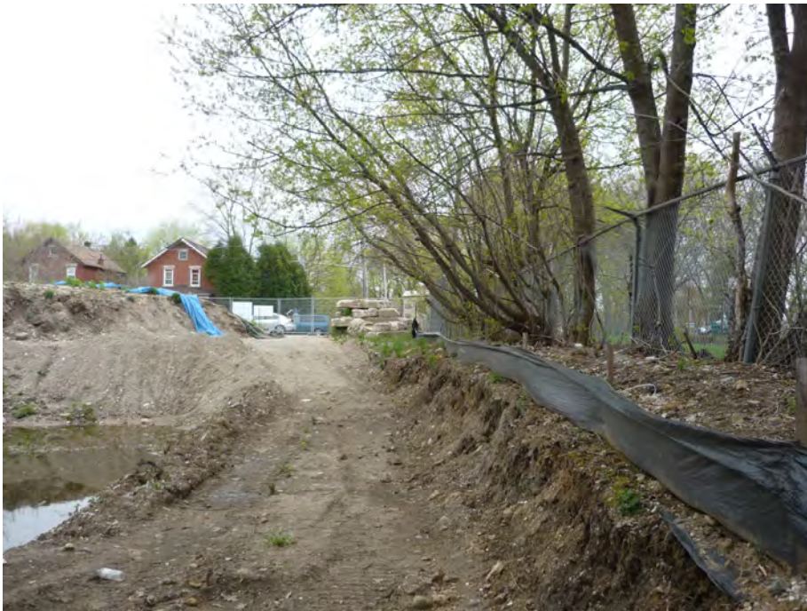
Photograph C-4: 180 Gordon Street west property boundary, looking south
