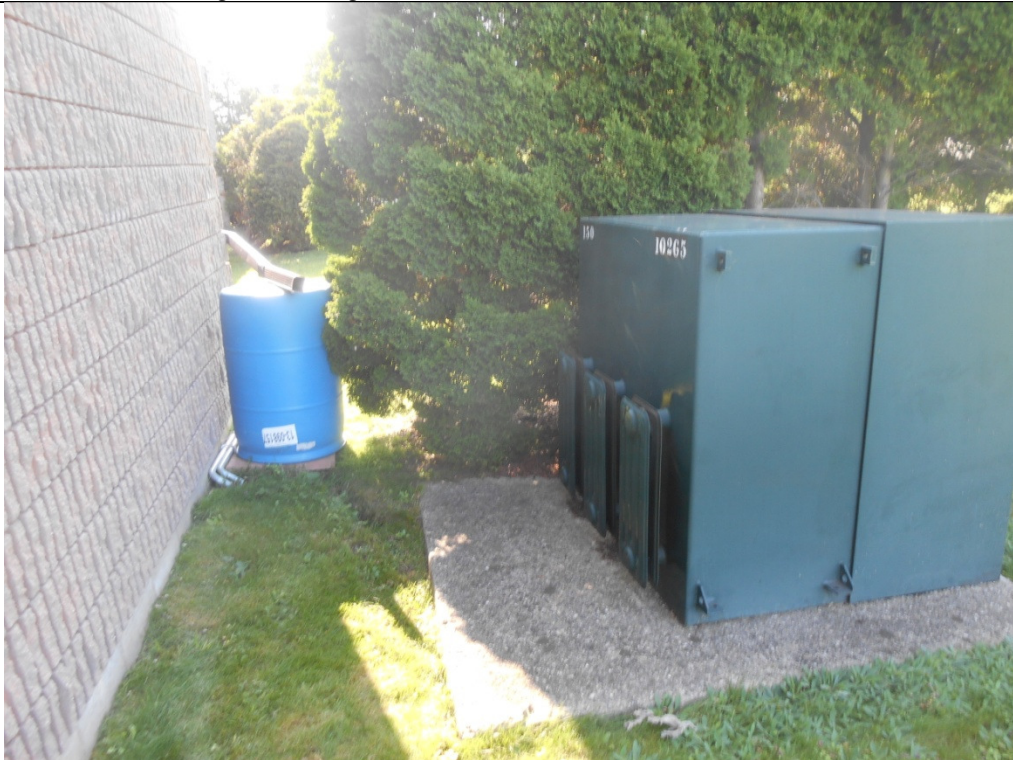
Photograph No. 2 View of transformer and drum holding downspout on adjacent church property to the west.
