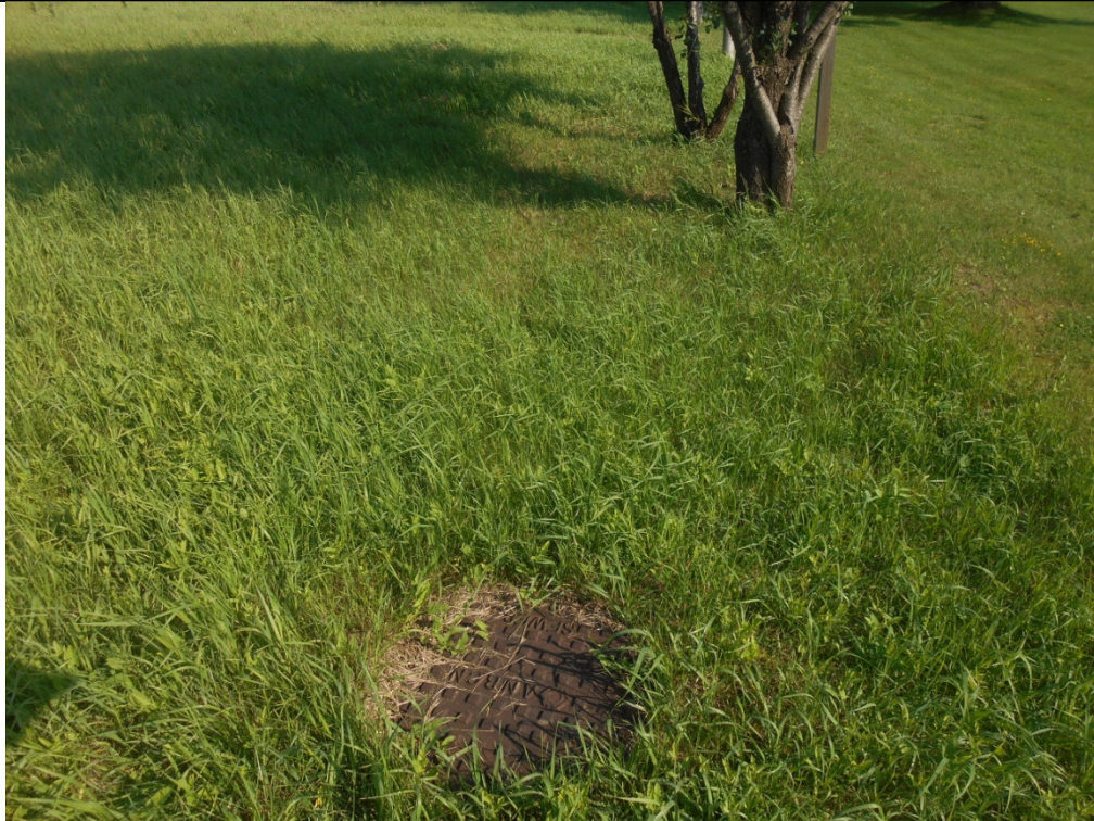
Photograph No. 3 View of manhole cover along western Property boundary.
