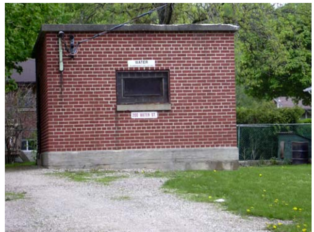
Water Street well house, Guelph, ON
