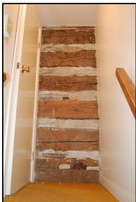
Figure 11 – Log wall construction exposed on interior of rear wall.
