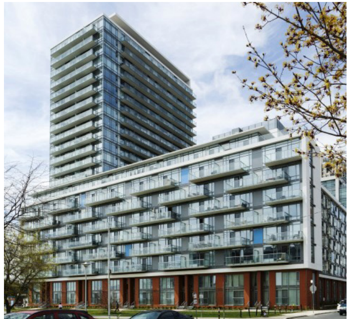
Taller buildings should be massed with clearly defined podium and tower features.
