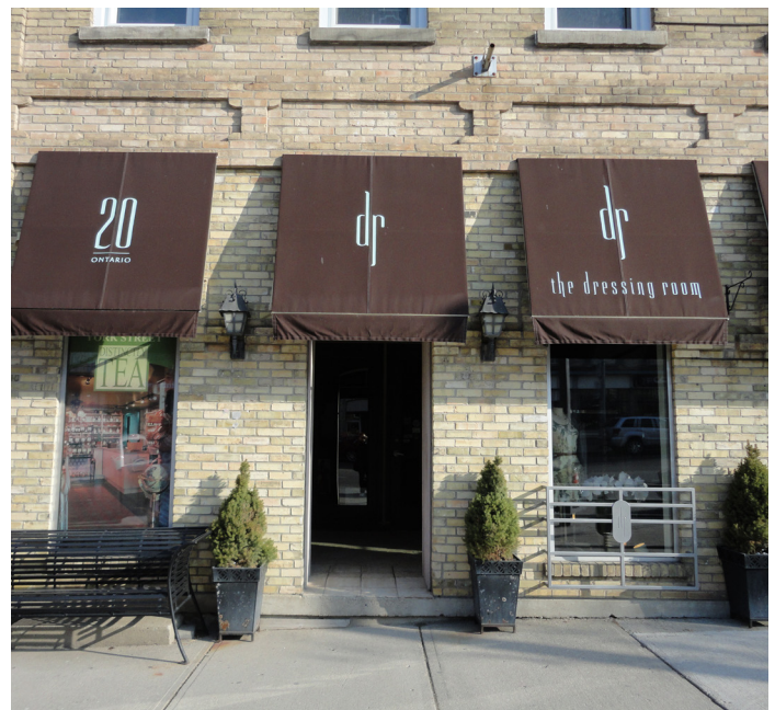
Example of successful application of chemical cleaners.
