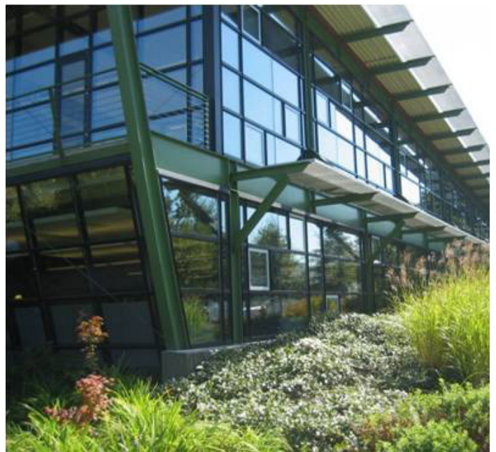
Vegetated or “green” roofs are recommended, especially in areas with minimal landscaping.
