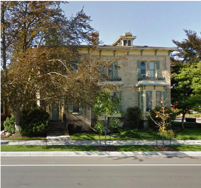
View of an existing residential dwelling on the corner of Norfolk and Suffolk Streets.
