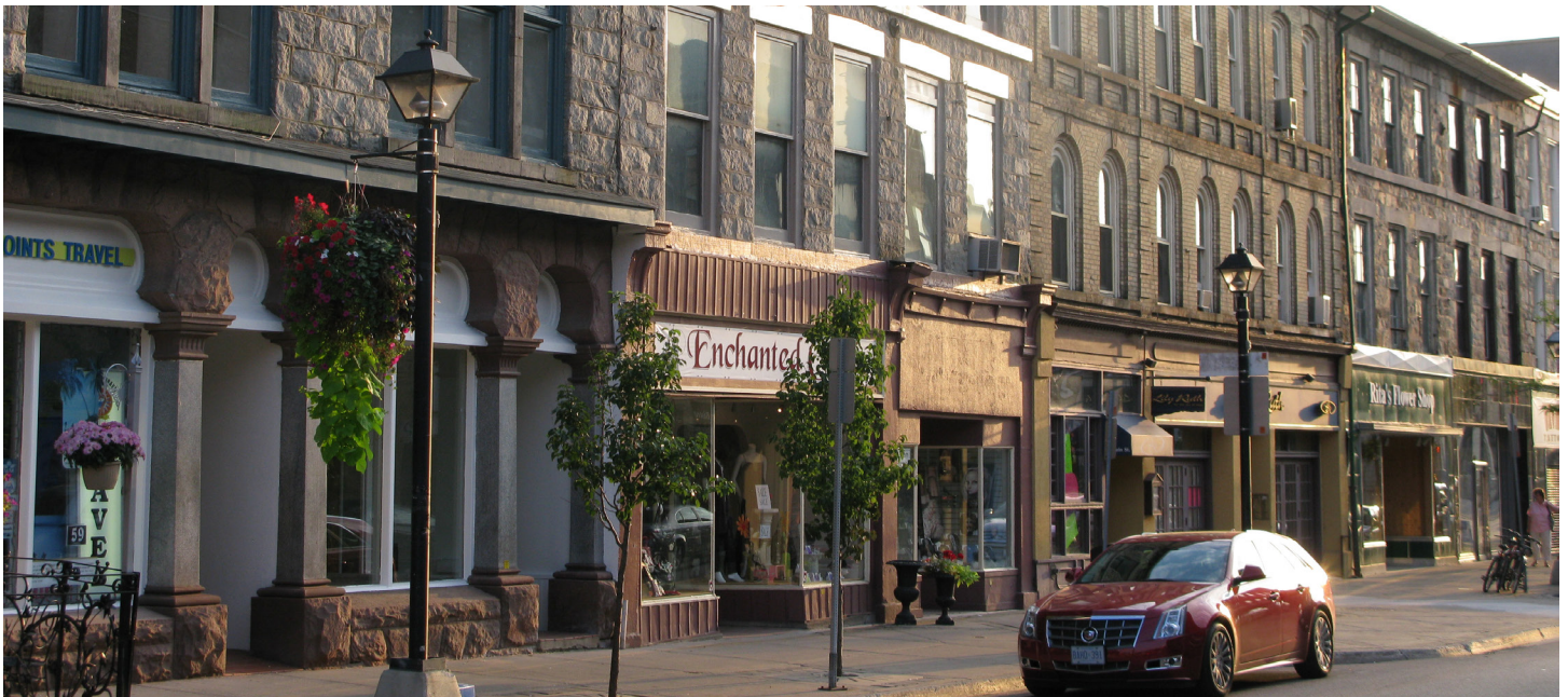
The use of natural stone and solid bricks is encouraged over the use of veneers and manufactured / composite materials.
