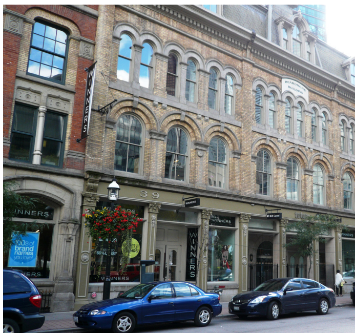
Existing brick should be retained and/or repaired.
