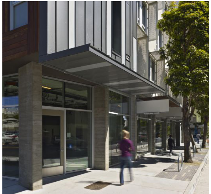
A single style of canopy should be used throughout the length of the building.
