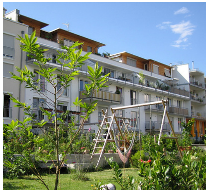
Locate and design shared private outdoor amenity space to maximize access to sunlight.
